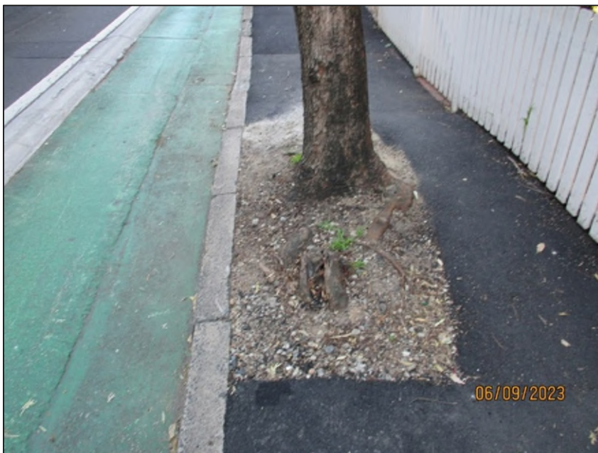
Plate 2: Street tree with small, unsealed area over part of the SRZ. Note exposed surface roots (facing east)
