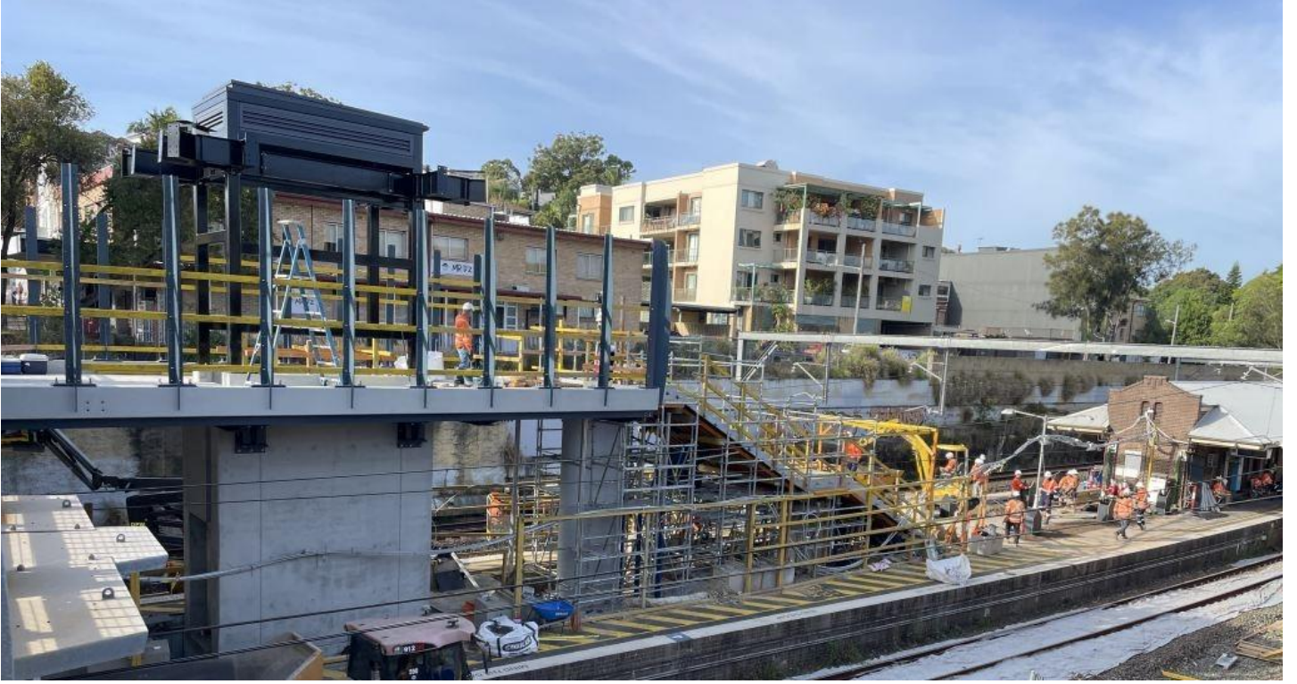
Construction of new stairs and elevated walkway connecting Hartill-Law Avenue to the station platform
