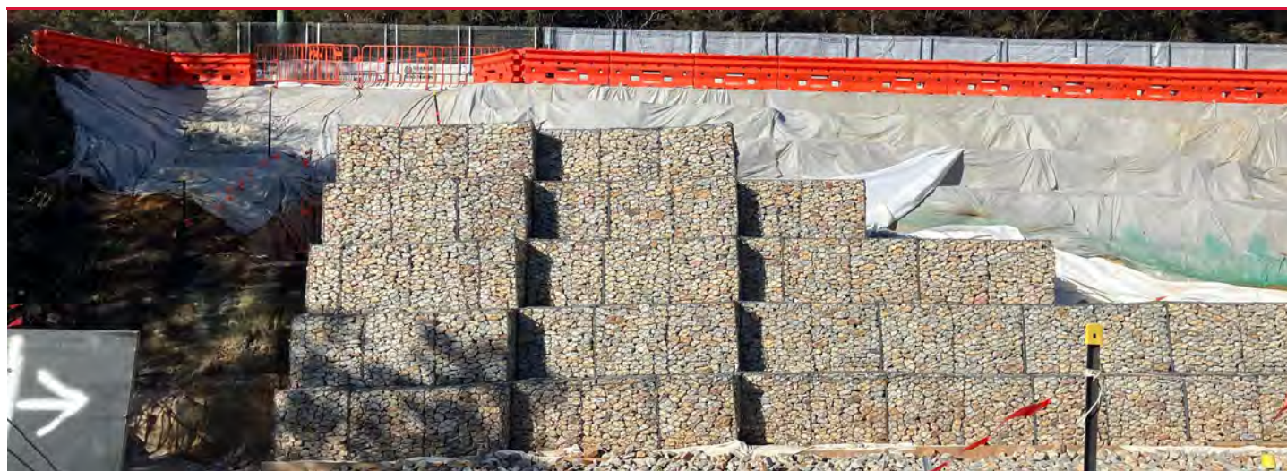
The gabion baskets being constructed at the Katoomba U-turn Bay slope failure site.
