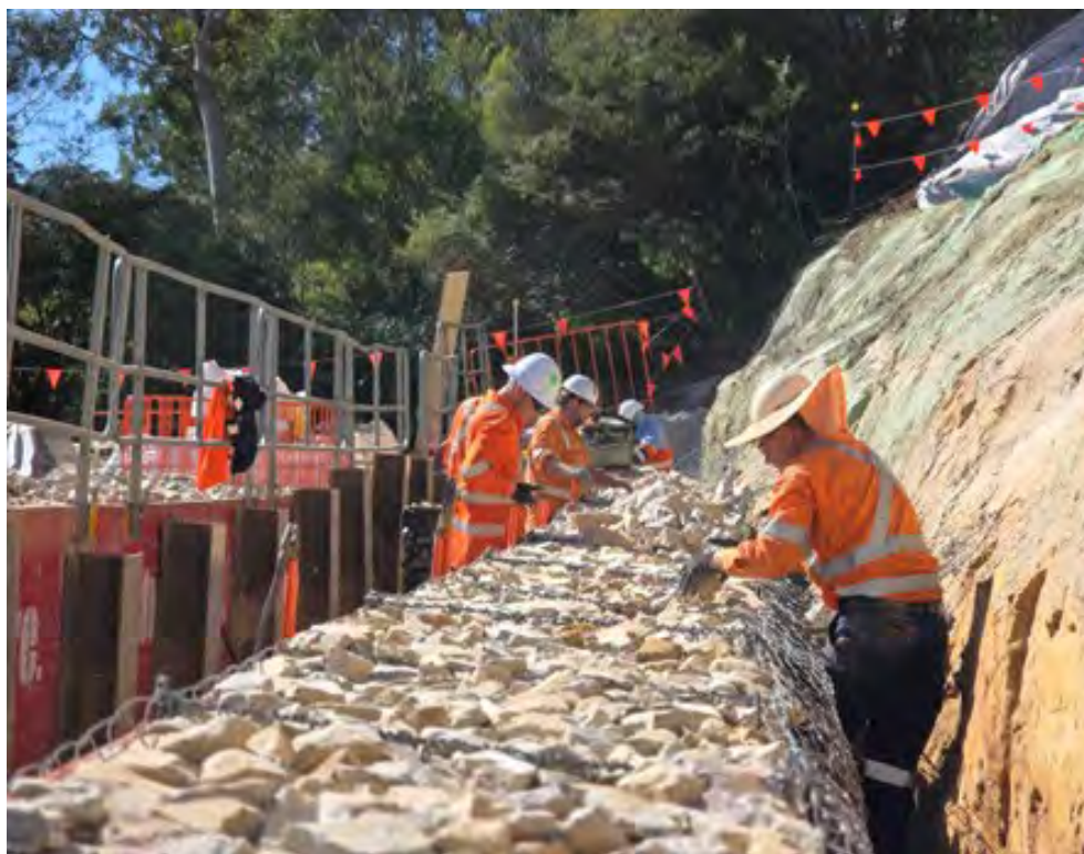
Building the gabion basket at Katoomba U-turn Bay
