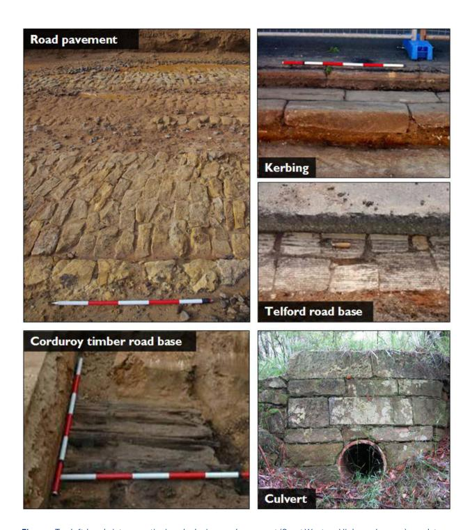
Figures: Top left-hand picture continuing clockwise: road pavement (Great Western Highway, Lawson); sandstone kerbing (Parramatta Road, Mays Hill); Telford sandstone road base (Great Western Highway, Leura); ceramic conduit and sandstone culvert headwall (Blue Mountains, NSW); corduroy timber road base (Entrance Road, Wamberal).
