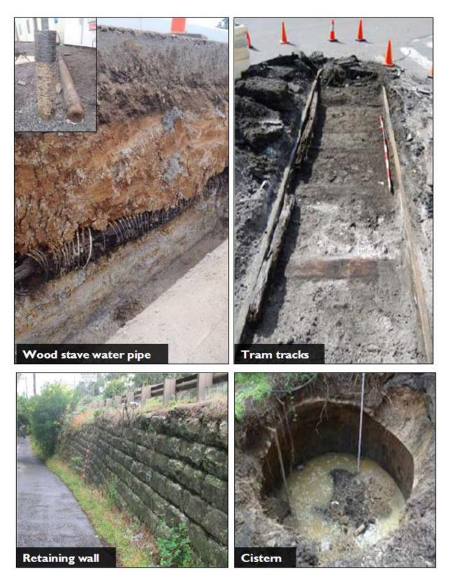
**Figures**: Top left hand picture continuing clockwise: woodstave water pipe with tar and wire sealing (Horsley drive); tram tracks (Sydney); brick lined cistern (Clyde); retaining wall (Great Western Highway, Leura).
