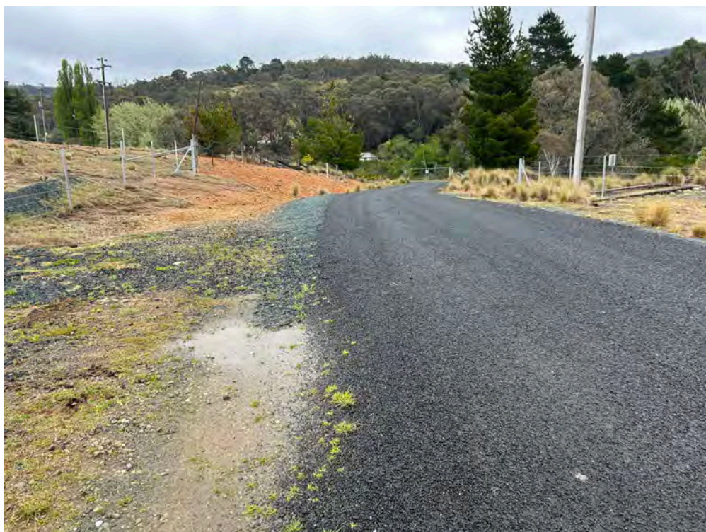
Photo 8: Sealed road over Copper Creek Road crossing, preventing inadvertent access to site materials underneath.
