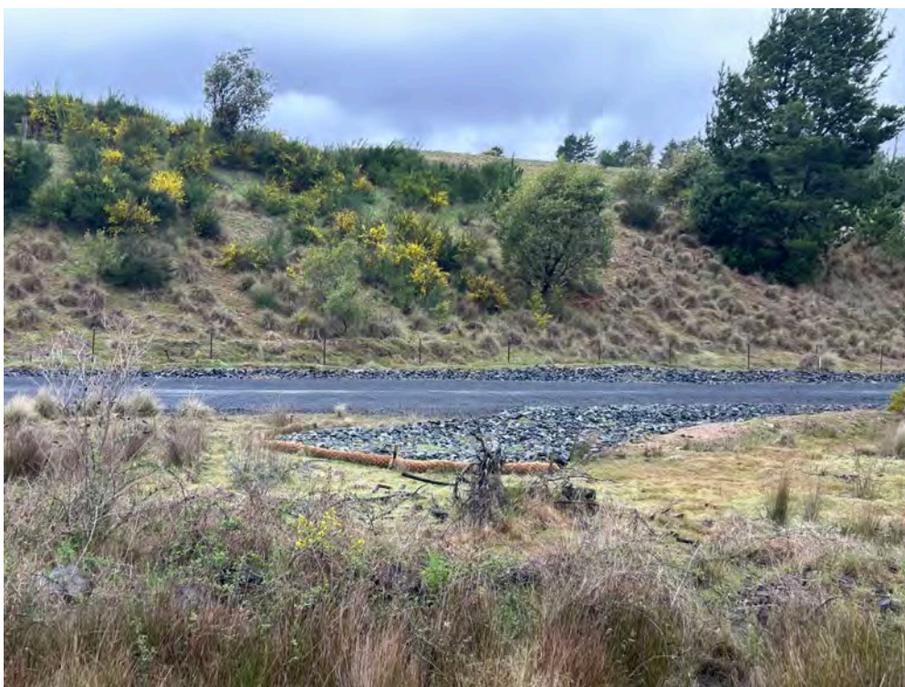
Photo 10: Rock armoury and sediment coir logs adjacent to the north of the site observed in the previous site inspection installed due to mine site remediation works are in good condition.
