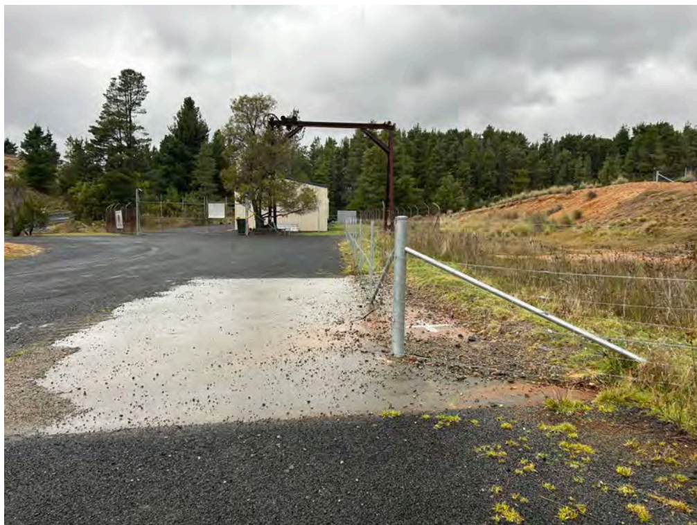
Photo 4: Some minor sediment visible on asphalt surface on site upgradient of Coppers Creek.
