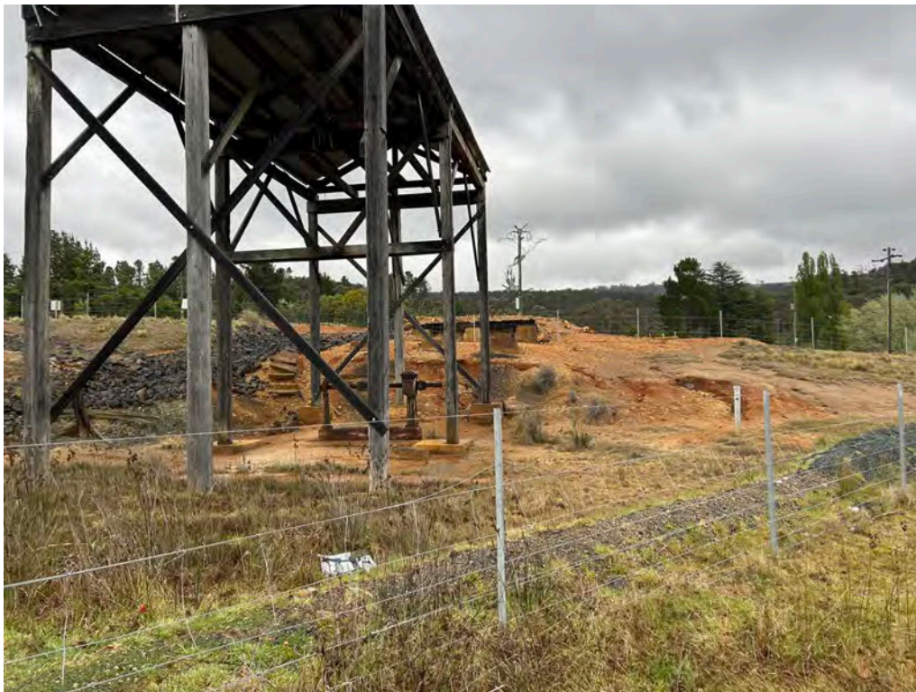
Photo 3: Minor evidence of erosion of soils on site. The condition has been observed during multiple previous inspections and has remained stable. Located adjacent to Former Loadout Facility and Weigh Bridge. Facing south.
