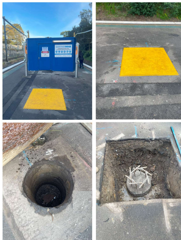
Image: Piling and foundation work on the station platform.
