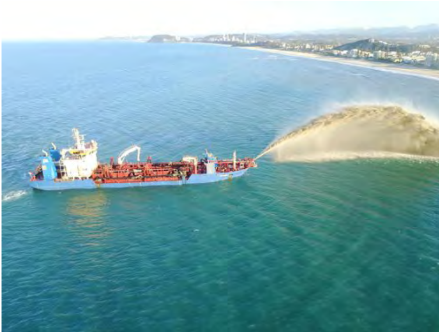
Figure 4-1: TSHD 'Rainbowing' dredged sand for beach nourishment (Source: Maritime and Civil Delivery Group)
