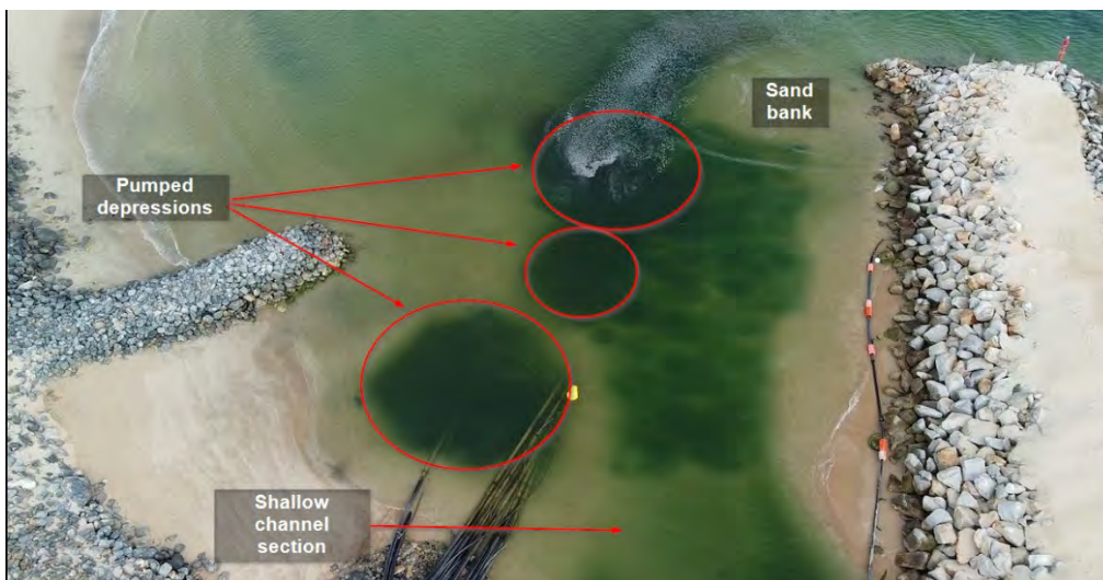
Figure 3-8: Visible non-uniform bed levels from pumping
