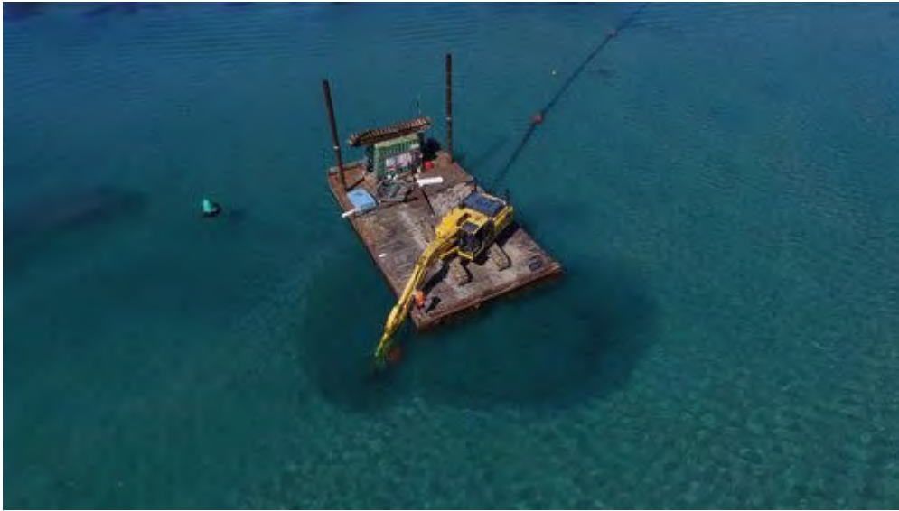
Figure 4-9: Barge-mounted backhoe (Source: Maritime and Civil Delivery Group)
