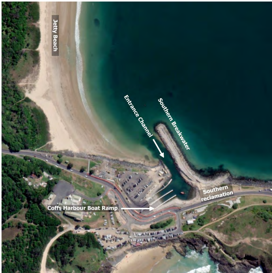
Figure 1-2: Coffs Harbour Boat Ramp
