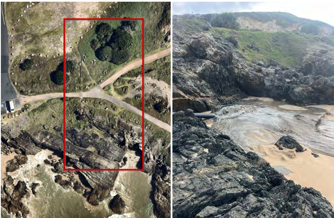
Figure 3-2: Aerial imagery of the discharge pipeline exiting at Gallows Beach (left), Photo of the discharge pipeline outlet at Gallows Beach (right)
