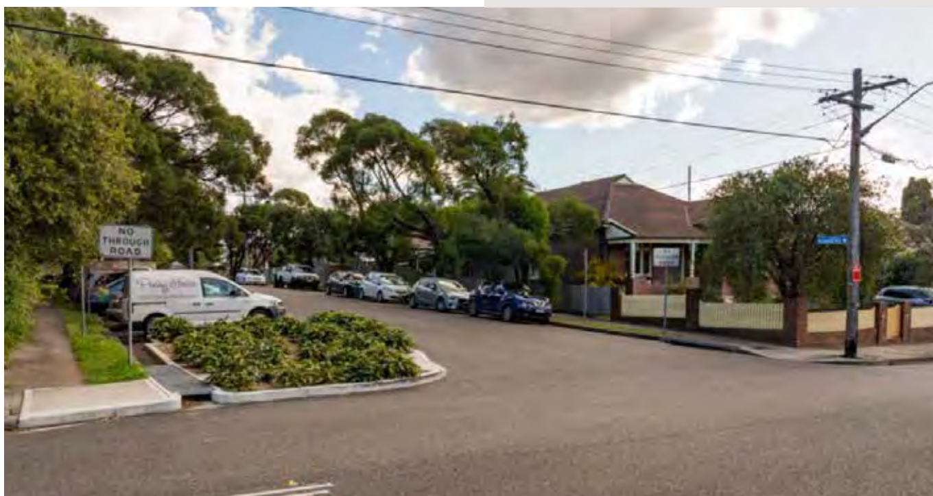
Kerb build outs improve place outcomes by increasing and expanding pedestrian space and providing opportunities for landscaping
