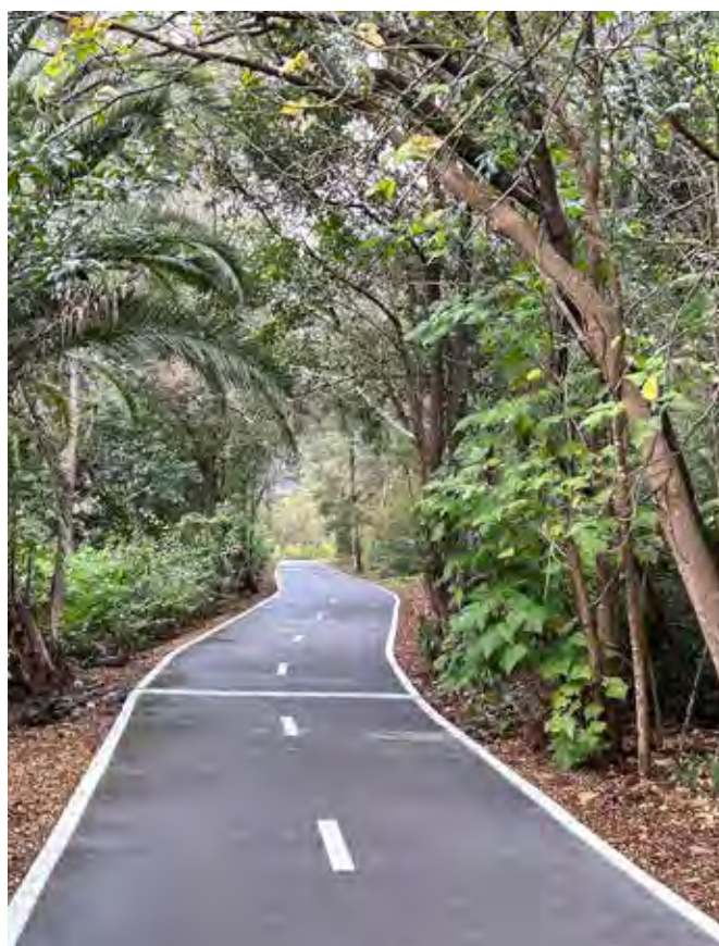
Shared path through bushland that links with the Kangaroo Point Boardwalk. Funded by Get NSW Active and delivered by Hornsby Shire Council
