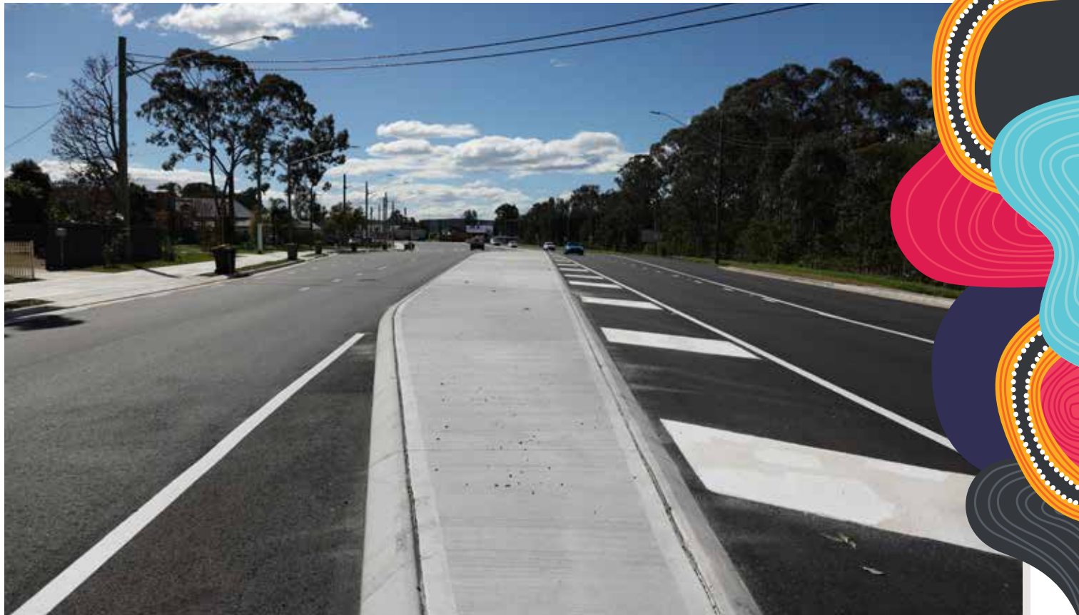
The new raised concrete median improves safety for motorists by separating northbound and southbound traffic along Henry Lawson Drive.
