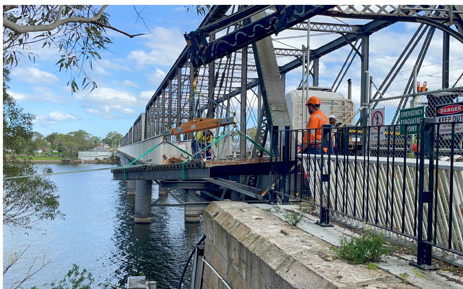
The crew maneuvering a section of the walkway through the truss at the northern end of the bridge.
