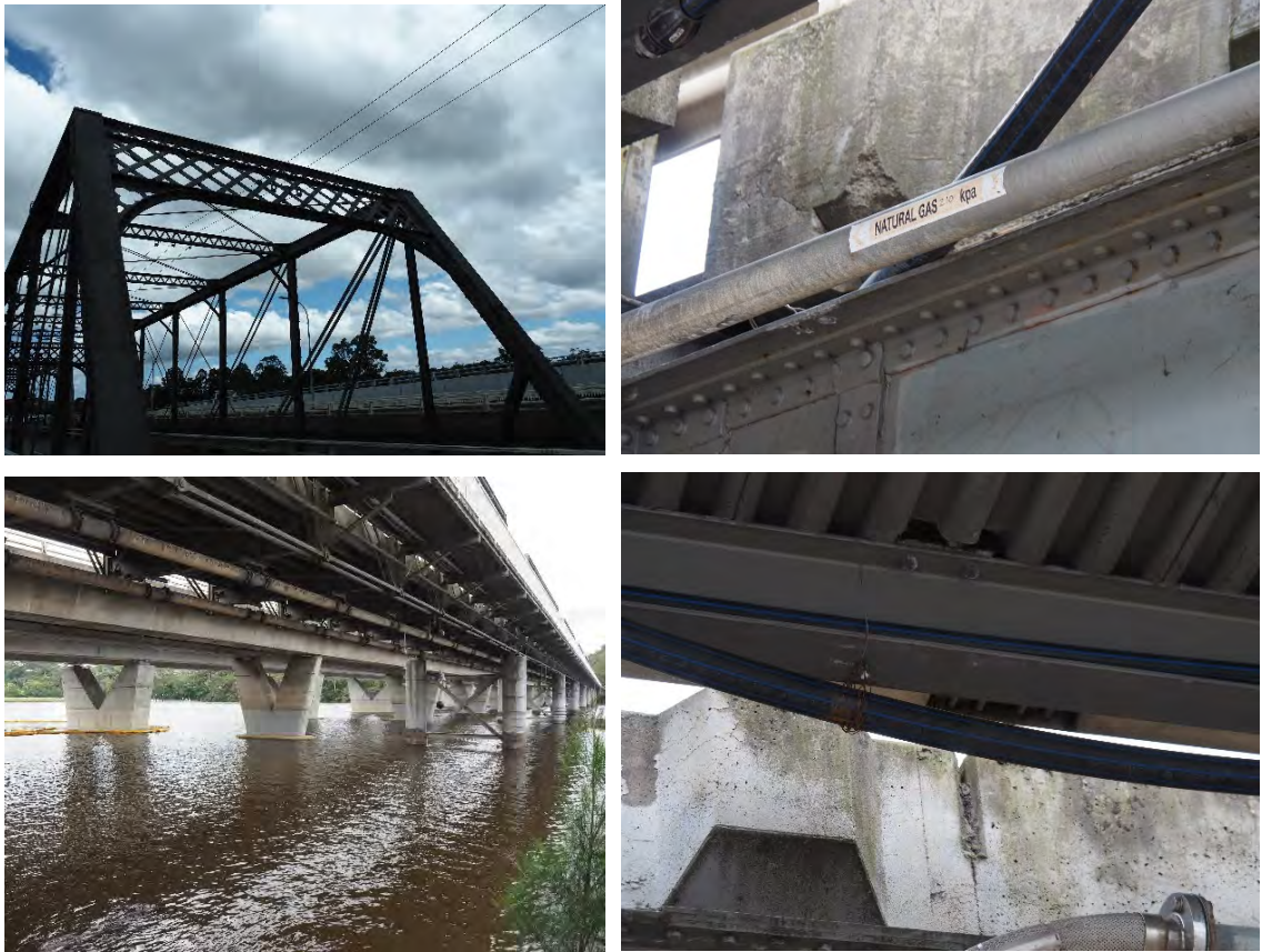
Figure 3-11 Utilities located on the bridge (Source: FBE)
