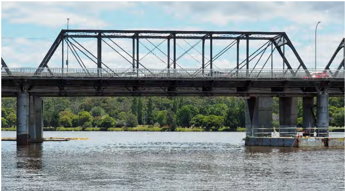
Figure 4-4 Whipple Truss Nowra Bridge (Source: FBE)
