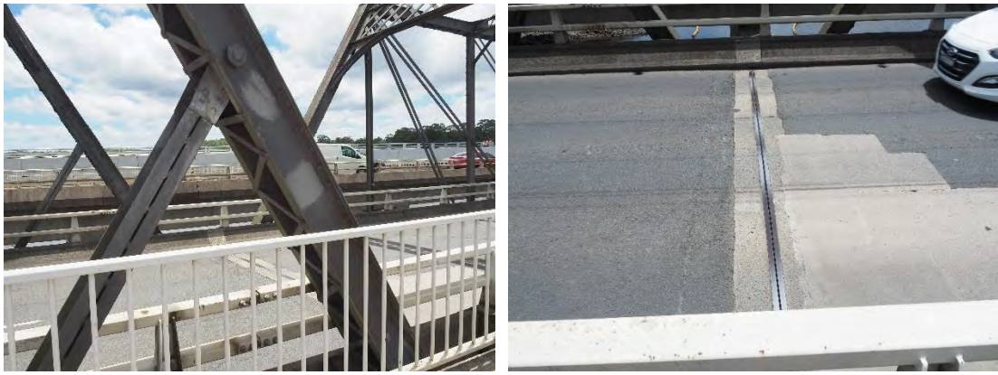
Figure 3-4 Bridge joint with steel nosing (Source: FBE)
