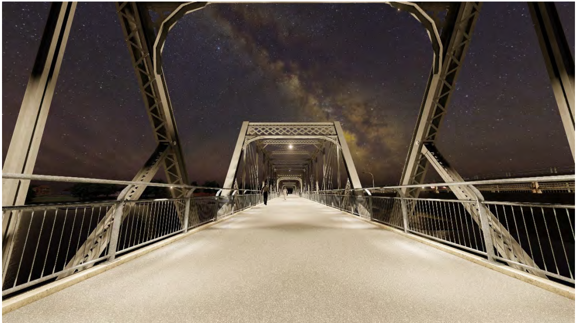
Figure 9-10 Handrail lighting combined with feature lighting (Source: FBE)
