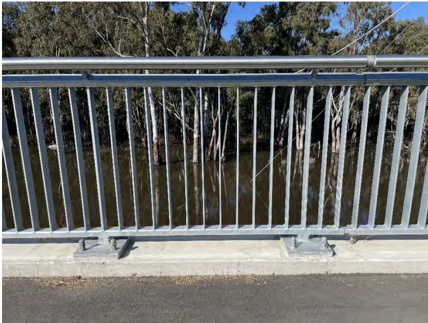
Figure 9-5 Pedestrian balustrade railing at Echuca Campaspe River (Source: TfNSW)
