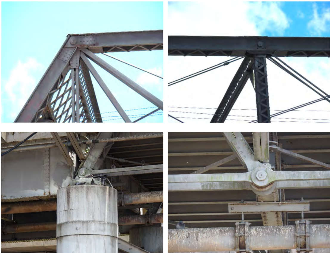
Figure 4-9 Various Aspects of the "Pin Connection" Whipple Truss (Source: FBE)
