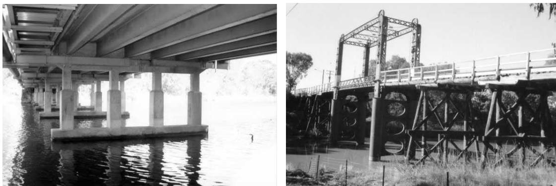
Figure 4-3 Steel beams at Wallarah Creek and lift Bridge at Brewarrina (Source: TfNSW)
