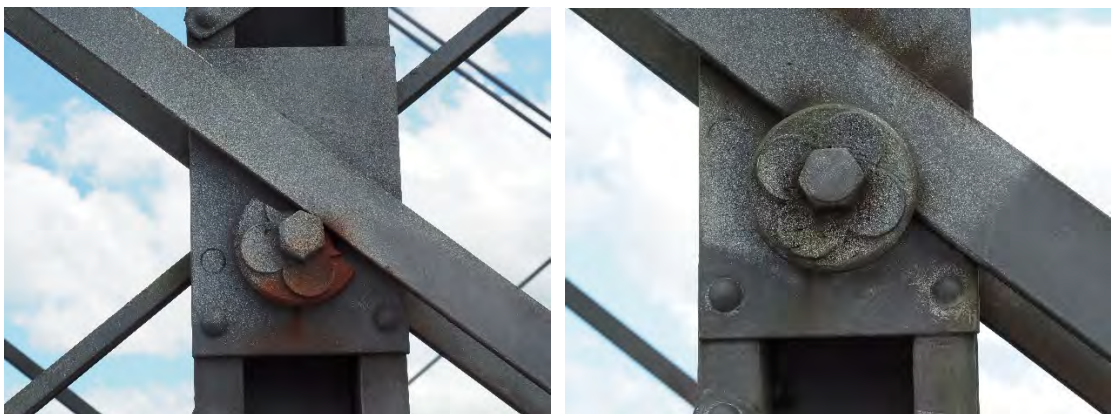
Figure 4-13 Tension member rosettes, LHS: broken, RHS: as-built condition (Source: FBE)
