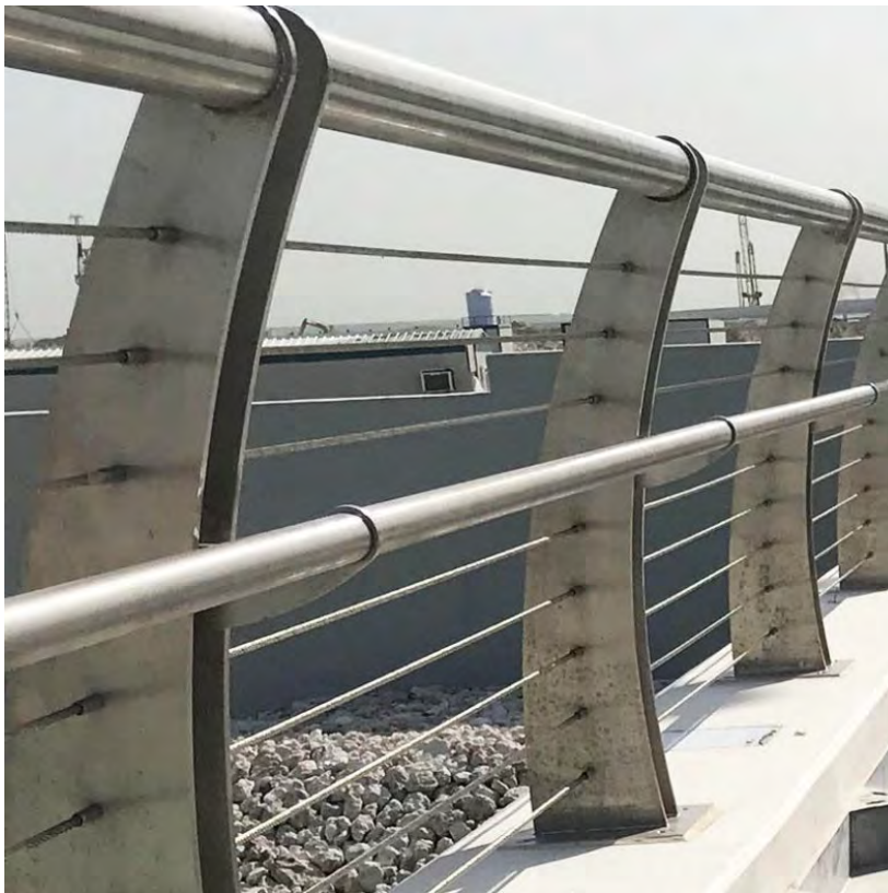
Figure 9-4 Stainless Steel Bridge Railing (Source: Unknown)
