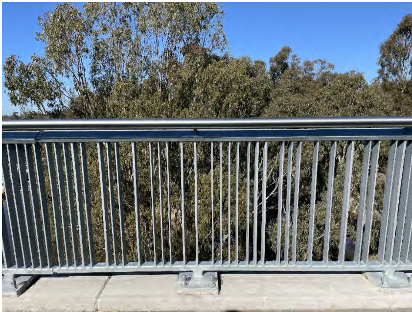
Figure 9-6 Pedestrian Balustrade Railing – Echuca over the Murray River (Source: TfNSW)
