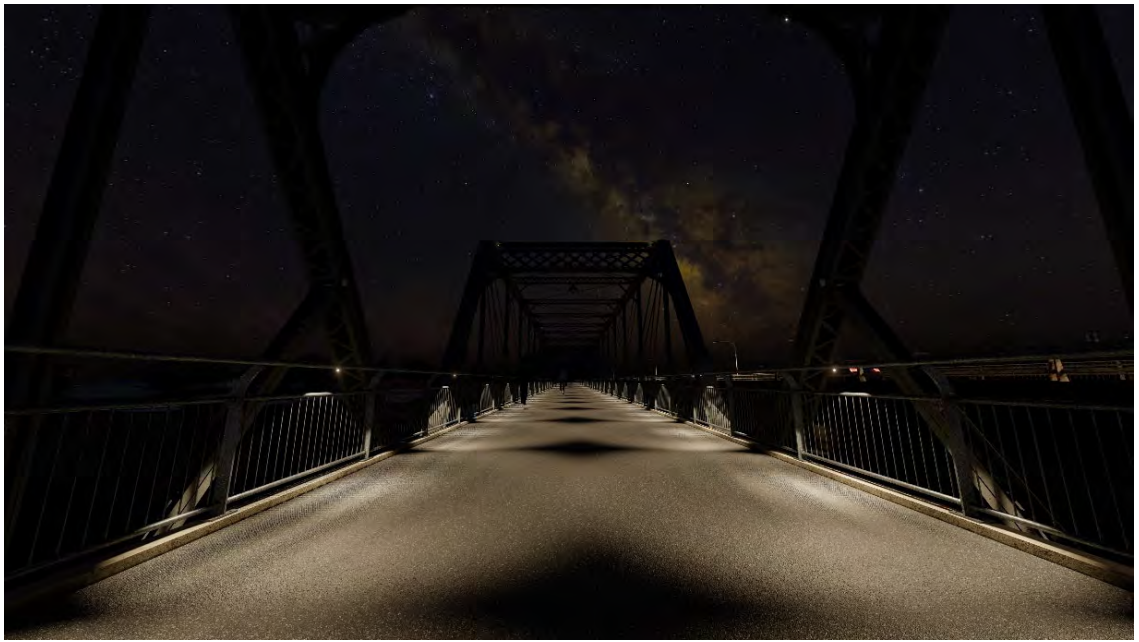
Figure 9-9 Handrail lighting without feature lighting (Source: FBE)
