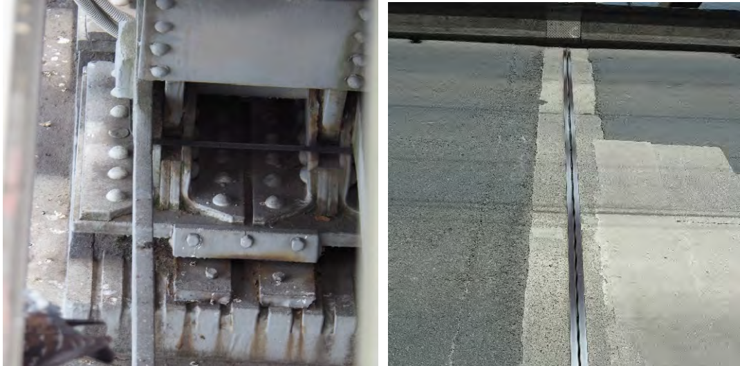
Figure 4-21 LHS: Bridge Bearing RHS Bridge Joints (Source: FBE)
