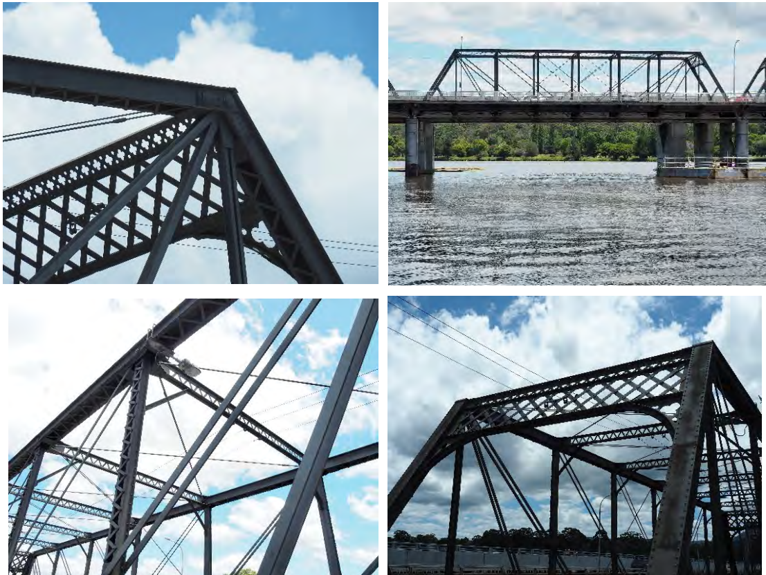
Figure 3-7 Various Views of the Nowra Bridge Whipple Truss (Source: FBE)
