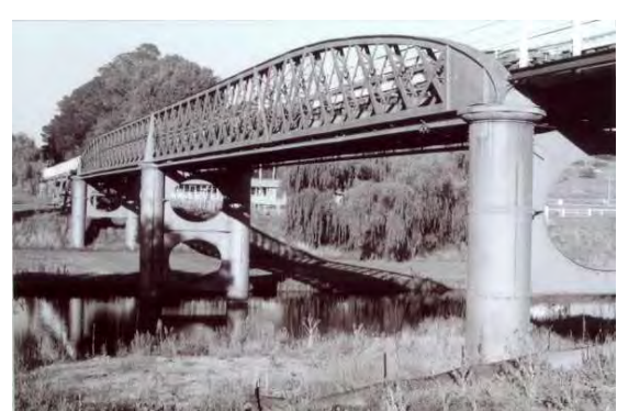
Figure 4-1 The Albury Arch and typical lattice truss (Source: TfNSW)
