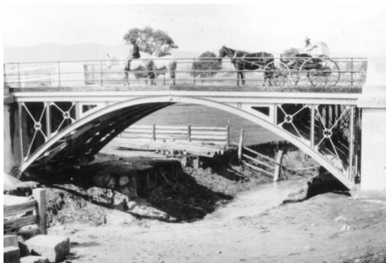
Figure 4-1 The Albury Arch and typical lattice truss (Source: TfNSW)
