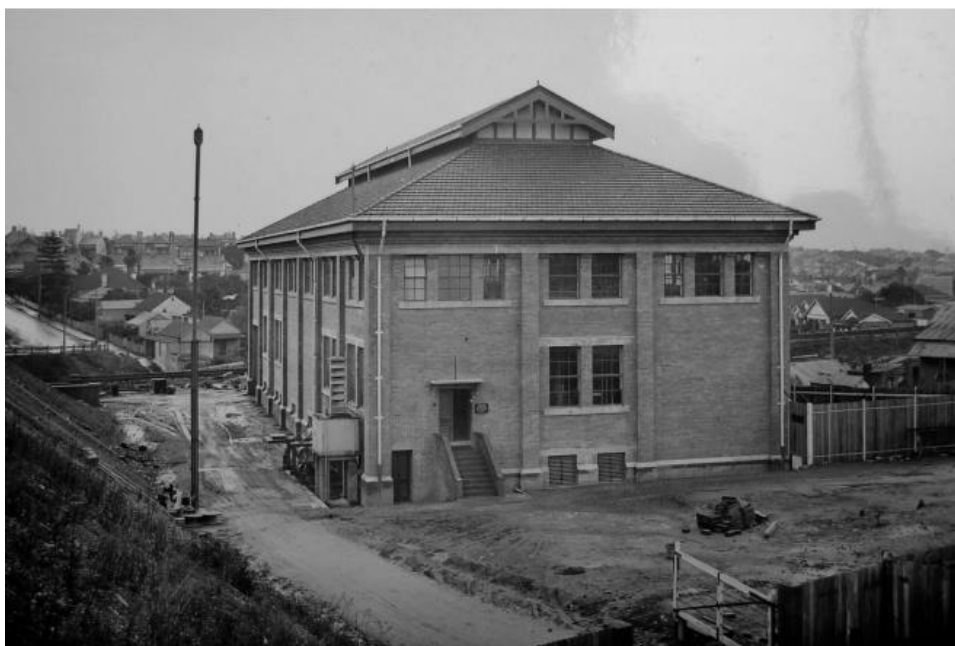
Figure 6-14: Exterior of the Lewisham Substation around the time of opening c. 1928 (Source: (Whitworth & Wood, 2021))
