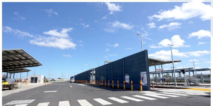
Noise walls at the maintenance centre
