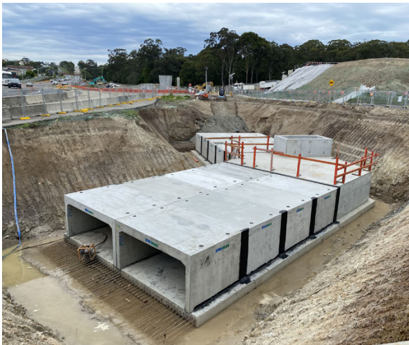
Dark Creek Culvert installation
