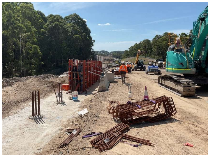
Image 5: Construction of noise wall at the mainline.
