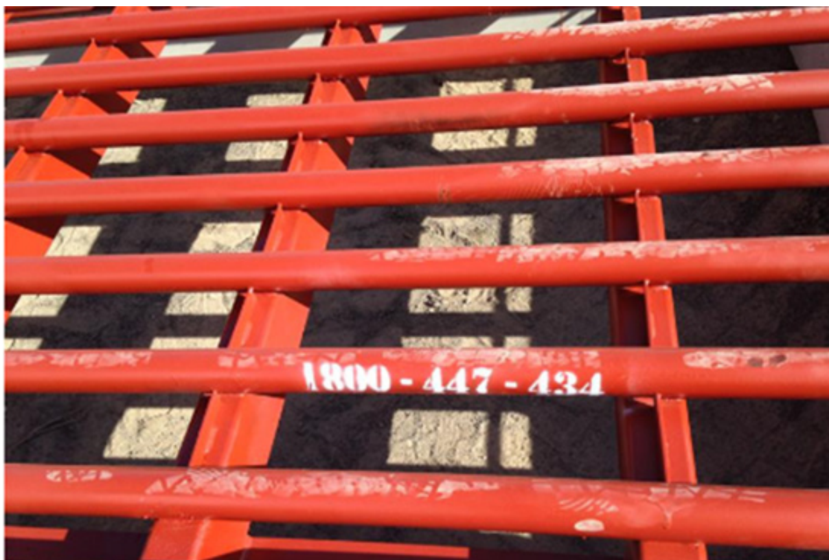
Figure 3-2 Example of grids to be installed across existing driveways and Brian Road with vertical bar on the bearers to discourage access
