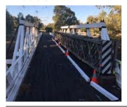
A Bailey bridge has been used at Paytens Bridge at least three times since 2000, most recently in 2017 (pictured) following overloading issues which required the bridge to be closed for a month.
