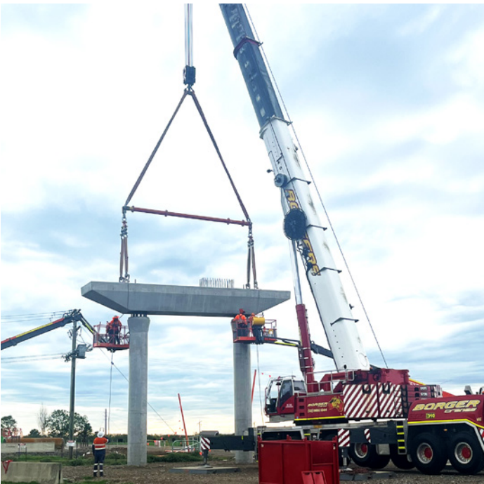
First headstock arriving on site for the bridge over the Doughboy Hollow floodplain
