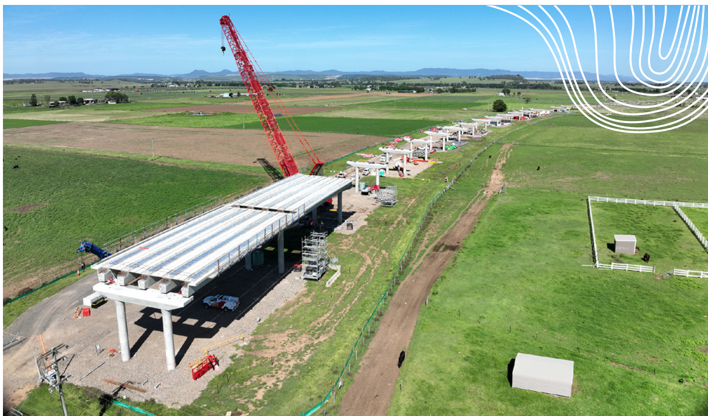
First girders on Doughboy Hollow floodplain bridge, looking towards Army Camp Road
