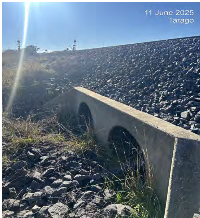
Photo 18: Upgradient of northernmost culvert with no surface water. No sediment build up was noted on rock armoury.
