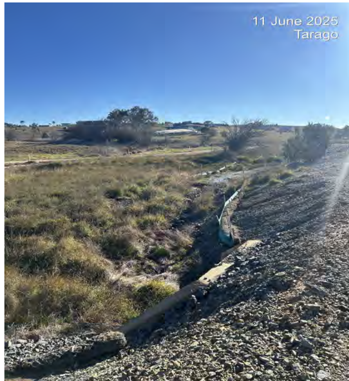
Photo 15: Sediment controls at the middle culvert upgradient of the railway line in good condition. Sediment buildup in front of coir logs remains similar to previous inspection.
