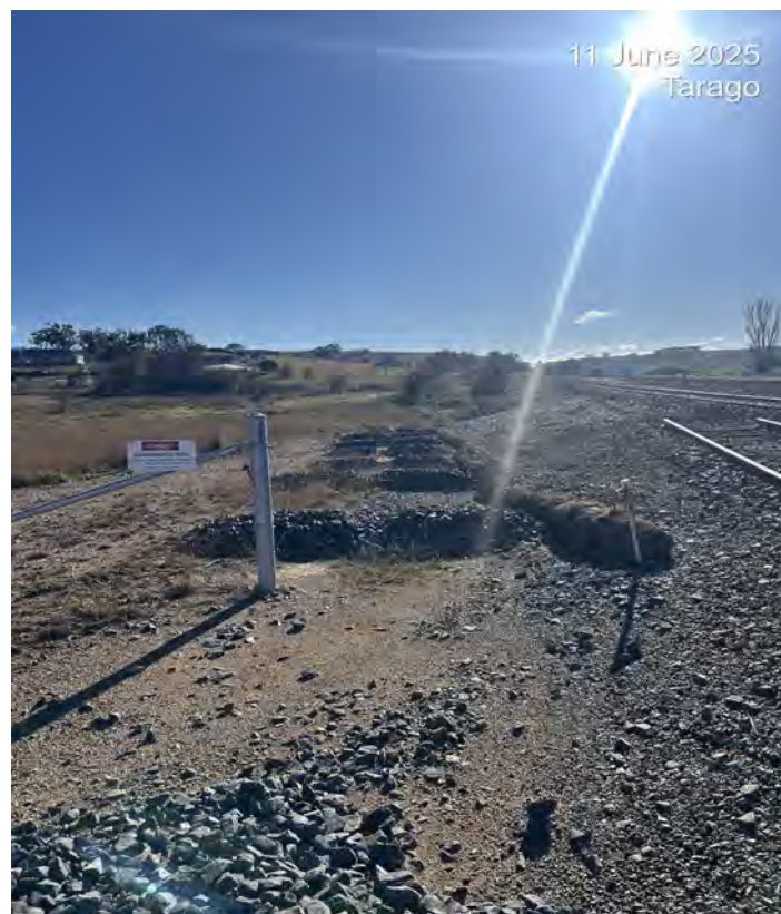
Photo 14: Rock armoury and sediment coir logs in drainage channel between southern and middle culverts appears to be in good condition.
