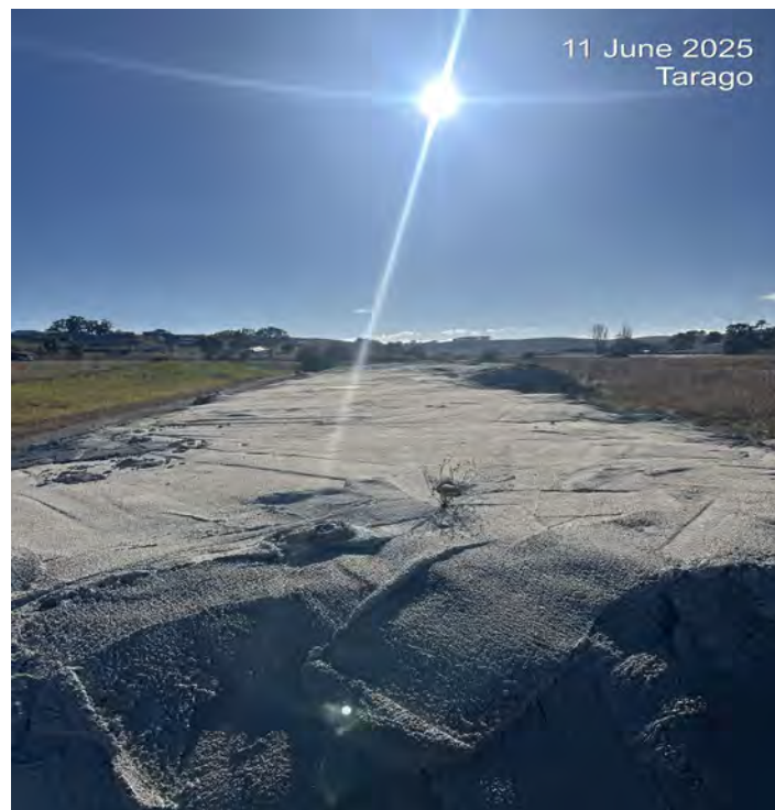
Photo 20: The concrete-capped stockpile is generally in good condition with no new exposure locations observed.
