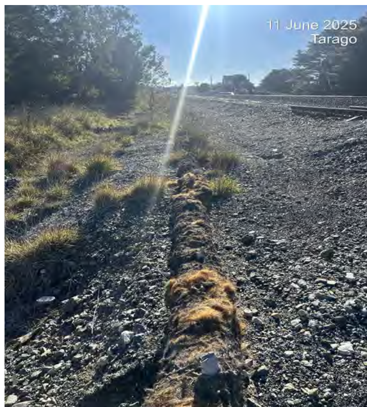
Photo 10: Sediment controls at southernmost culvert upgradient of the railway line.
