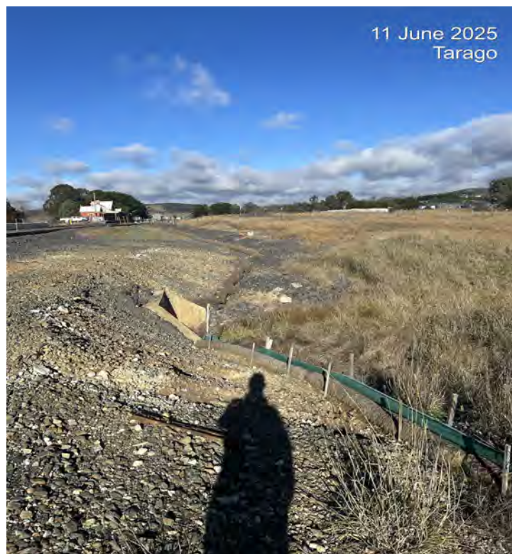
Photo 16: Sediment controls north of middle culvert, upgradient of railway line in good condition. Sediment buildup in front of coir logs remains similar to previous inspection.
