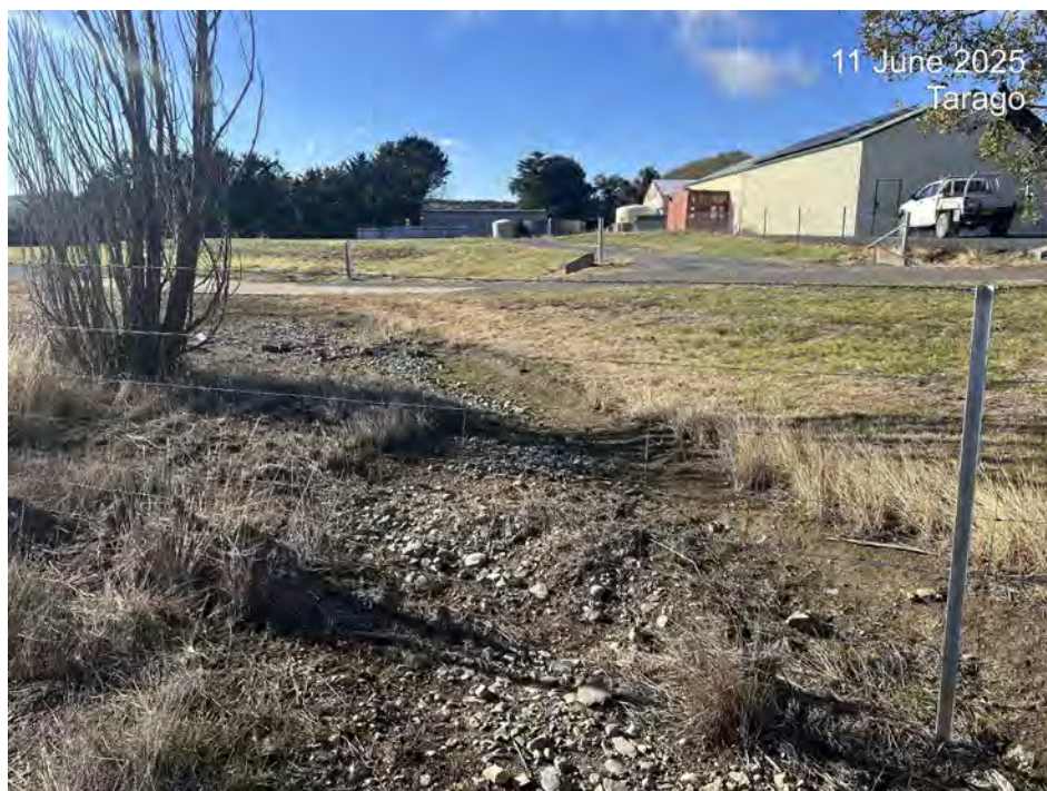
Photo 7: Downgradient of middle culvert. No water observed flowing offsite. No sediment observed on gravels.
