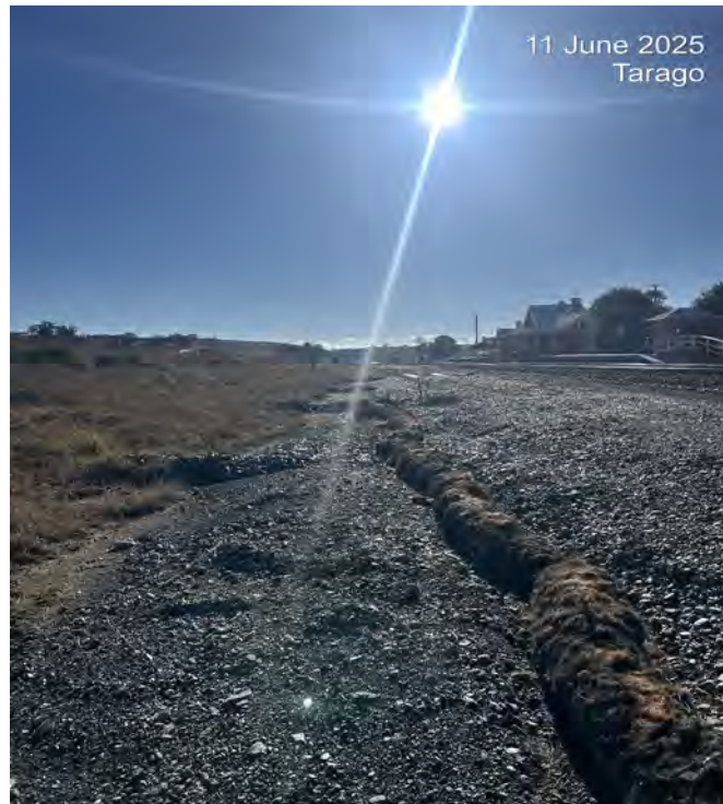
Photo 13: Rock armoury and sediment coir logs in drainage channel between southern and middle culverts appears to be in good condition.
