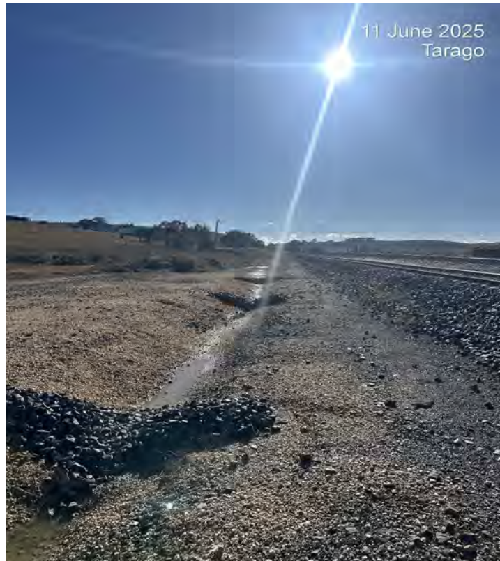
Photo 17: Sediment controls in drainage channel between middle and northern culverts appear to be in good condition. Minor surface water pooled on site.
