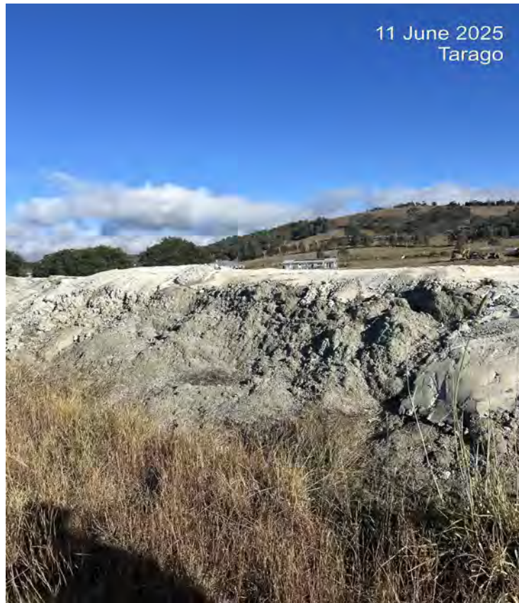
Photo 19: The concrete-capped stockpile is generally in good condition with no new exposure locations observed.
