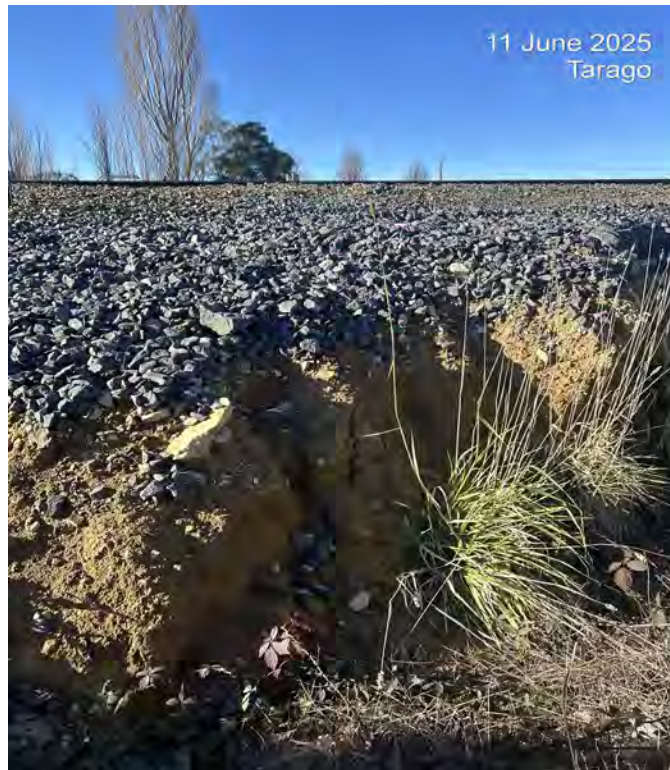
Photo 9: Southernmost culvert upgradient of the railway line. The erosion due to lack of ground cover observed during multiple previous inspections is still present.
