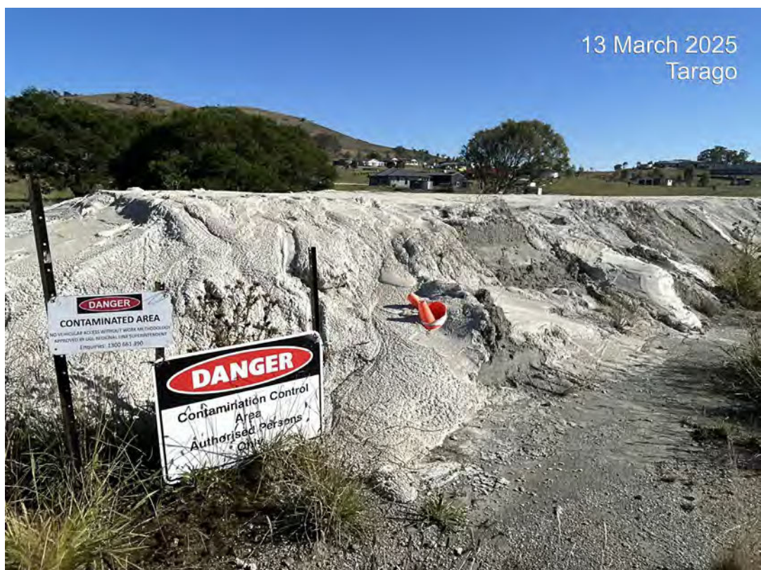
Photo 18: The concrete-capped stockpile is generally in good condition with no new exposure locations observed.
