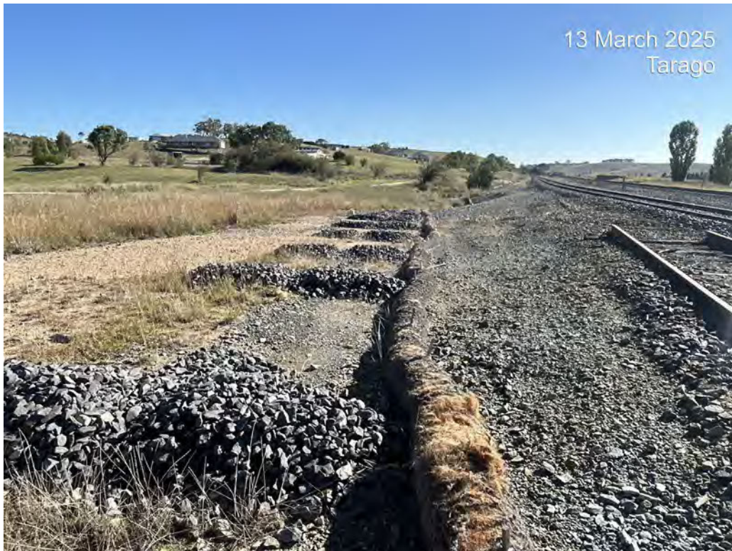
Photo 13: Rock armour and sediment coir logs in drainage channel between southern and middle culverts appears to be in good condition.
