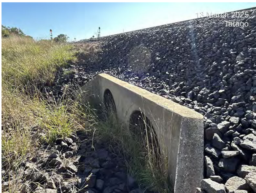
Photo 17: Upgradient of northernmost culvert with no surface water. No sediment build up was noted on rock armoury.
