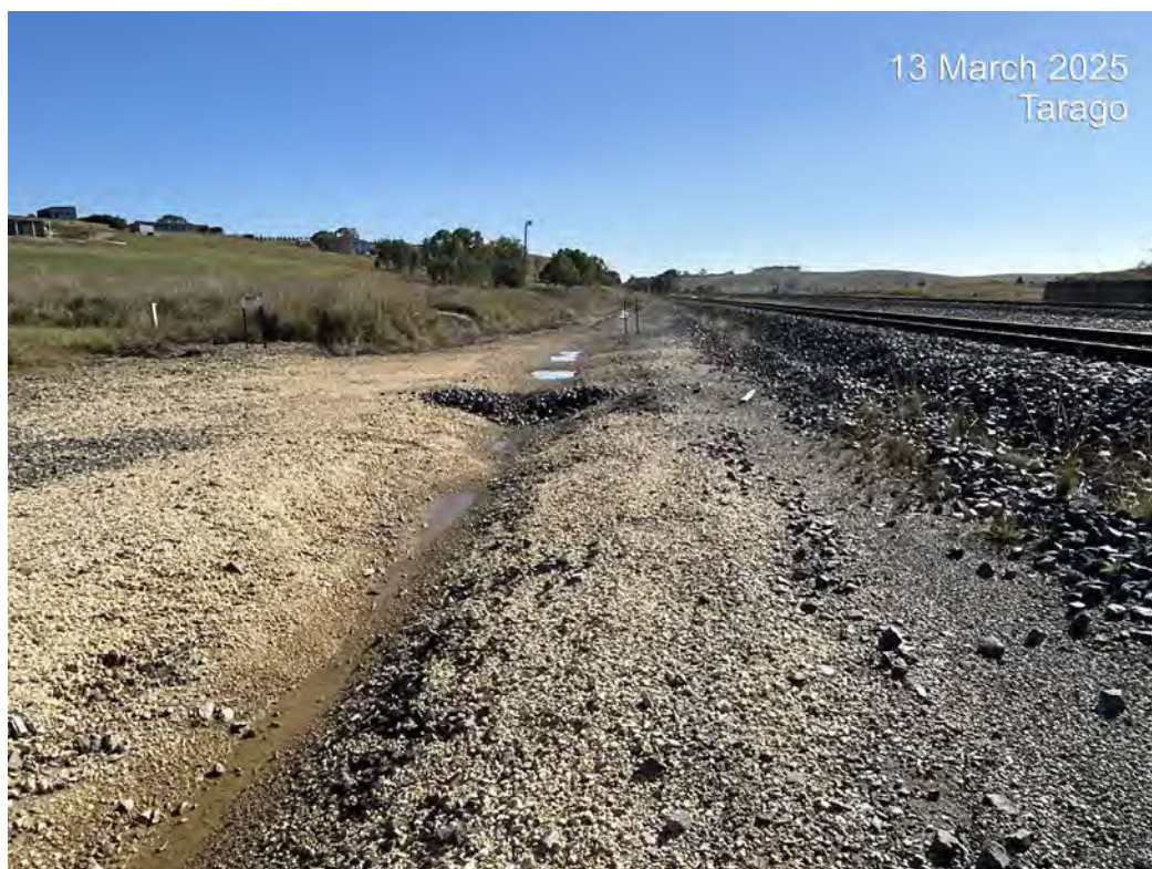
Photo 16: Sediment controls in drainage channel between middle and northern culverts appear to be in good condition.
