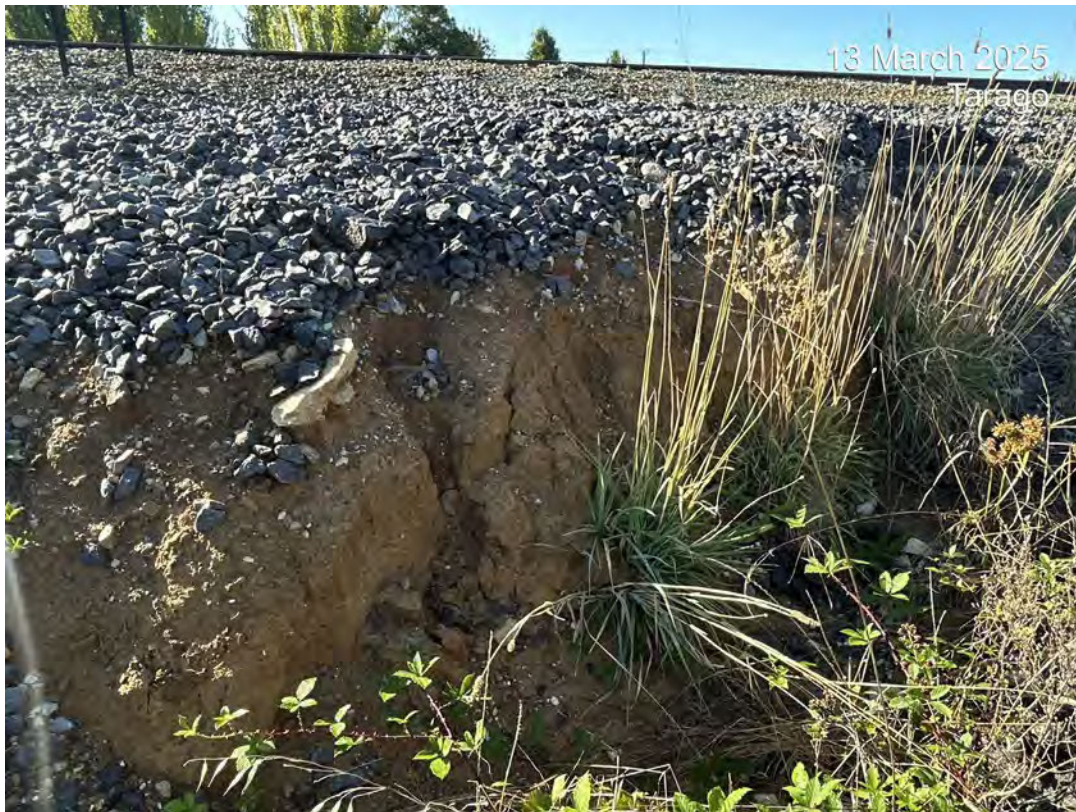
Photo 9: Southernmost culvert upgradient of the railway line. The erosion due to lack of ground cover observed during multiple previous inspections is still present.
