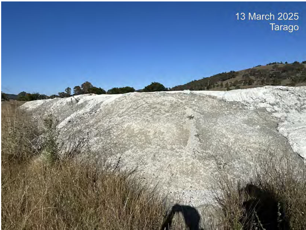
Photo 19: The concrete-capped stockpile is generally in good condition with no new exposure locations observed.
