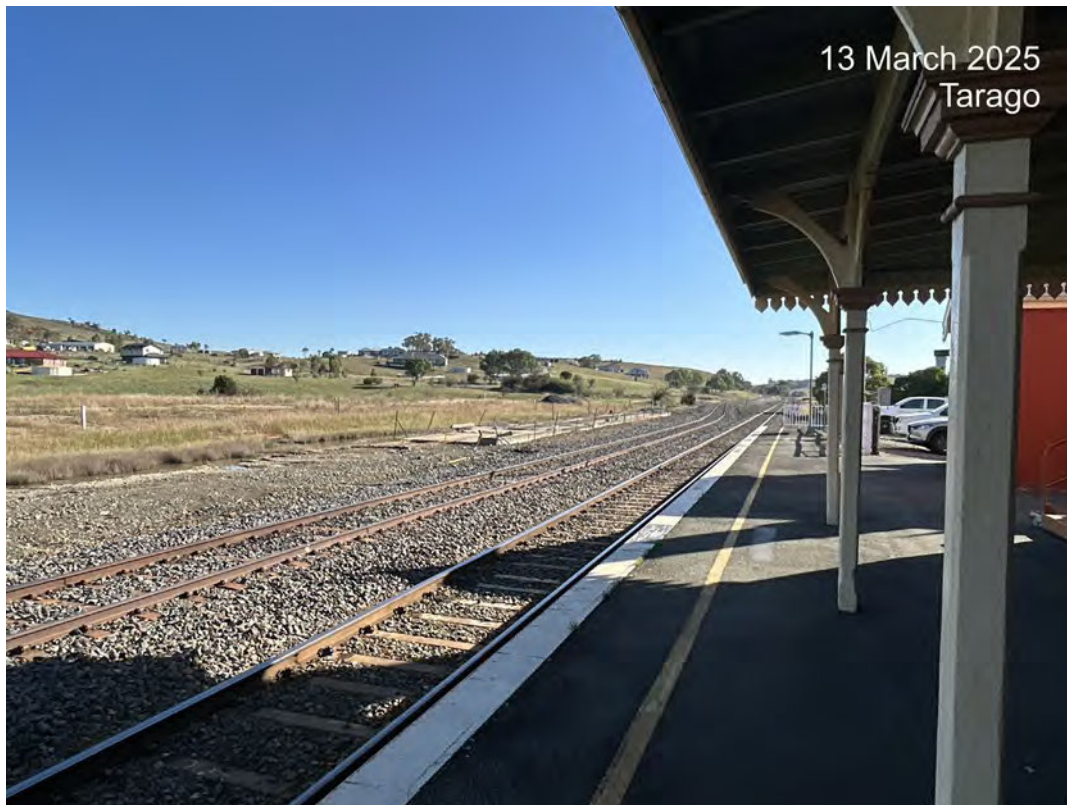
Photo 2: Picture facing northeast towards Tarago railway station, no airborne dust visible.
