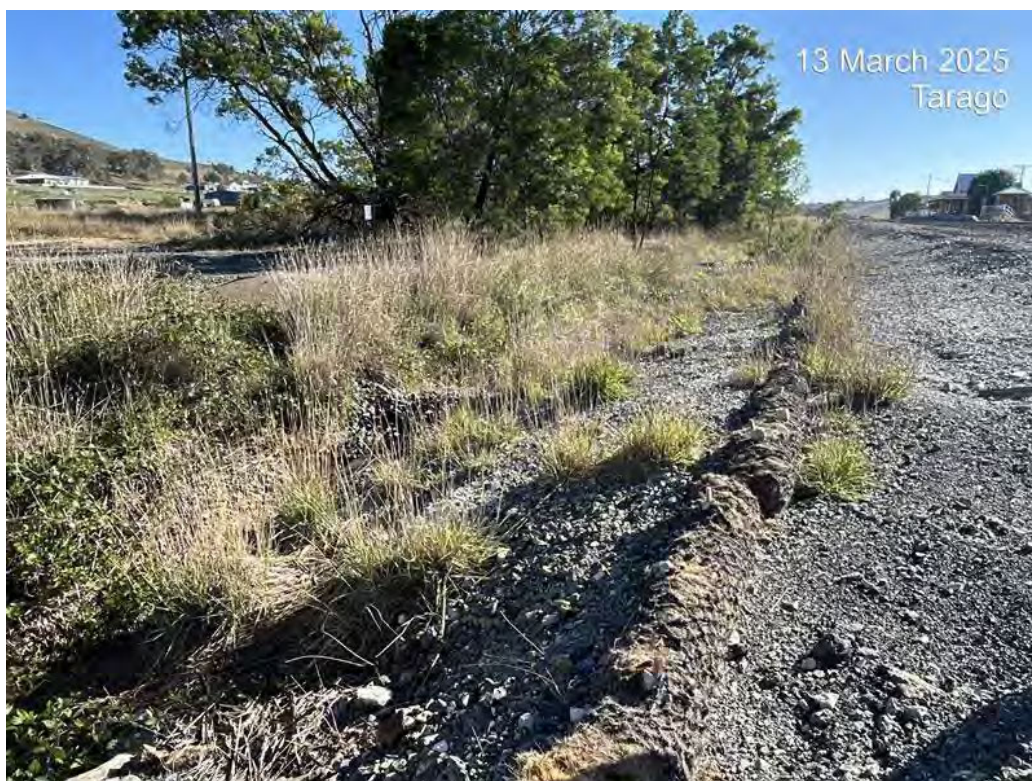
Photo 10: Sediment controls at southernmost culvert upgradient of the railway line.
