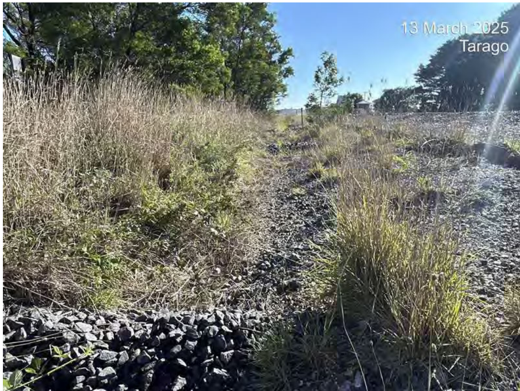
Photo 11: Rock armoury in drainage channel between southern and middle culverts. Minor sediment and vegetation buildup within drainage line.
