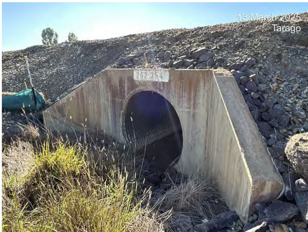
Photo 14: Sediment controls at the middle culvert upgradient of the railway line in good condition. Sediment buildup in front of coir logs remains similar to previous inspection.
