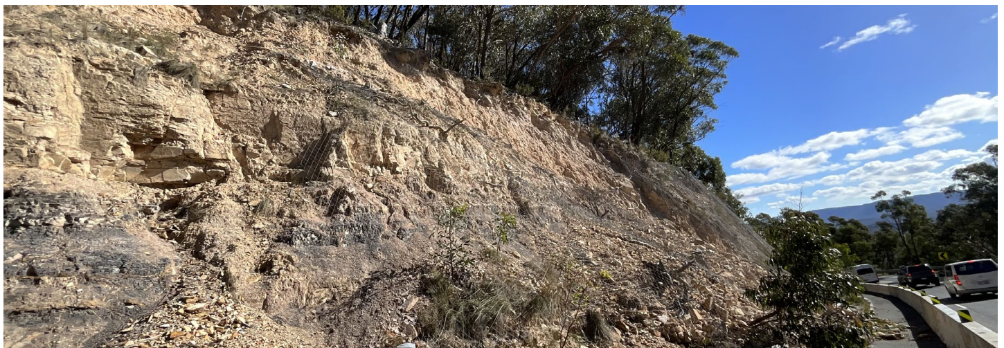
Failed slope on the Great Western Highway at Victoria Pass
