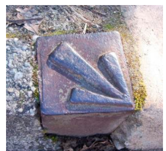
Alignment Pin references road alignment
