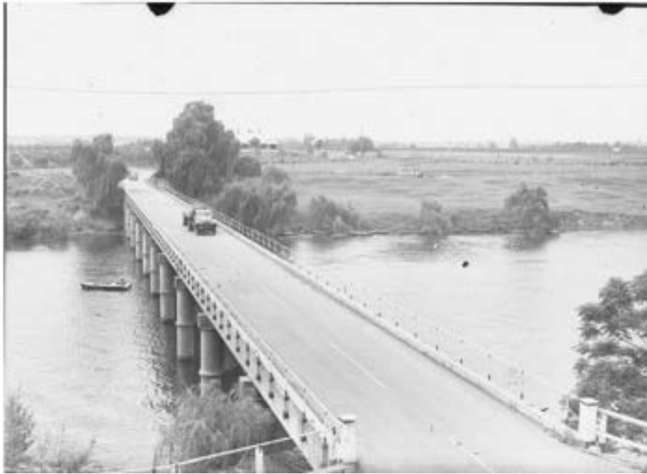
Figure 2-38 Windsor Bridge, 1947 (Source: SLNSW, Mitchell Library. GPO 1-40931, 1_40931r).
