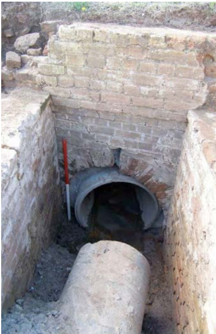
Figure 11 - Headwall pit of the Port Macquarie barrel drain (Source: E. A Higginbotham and Associates (2009))
