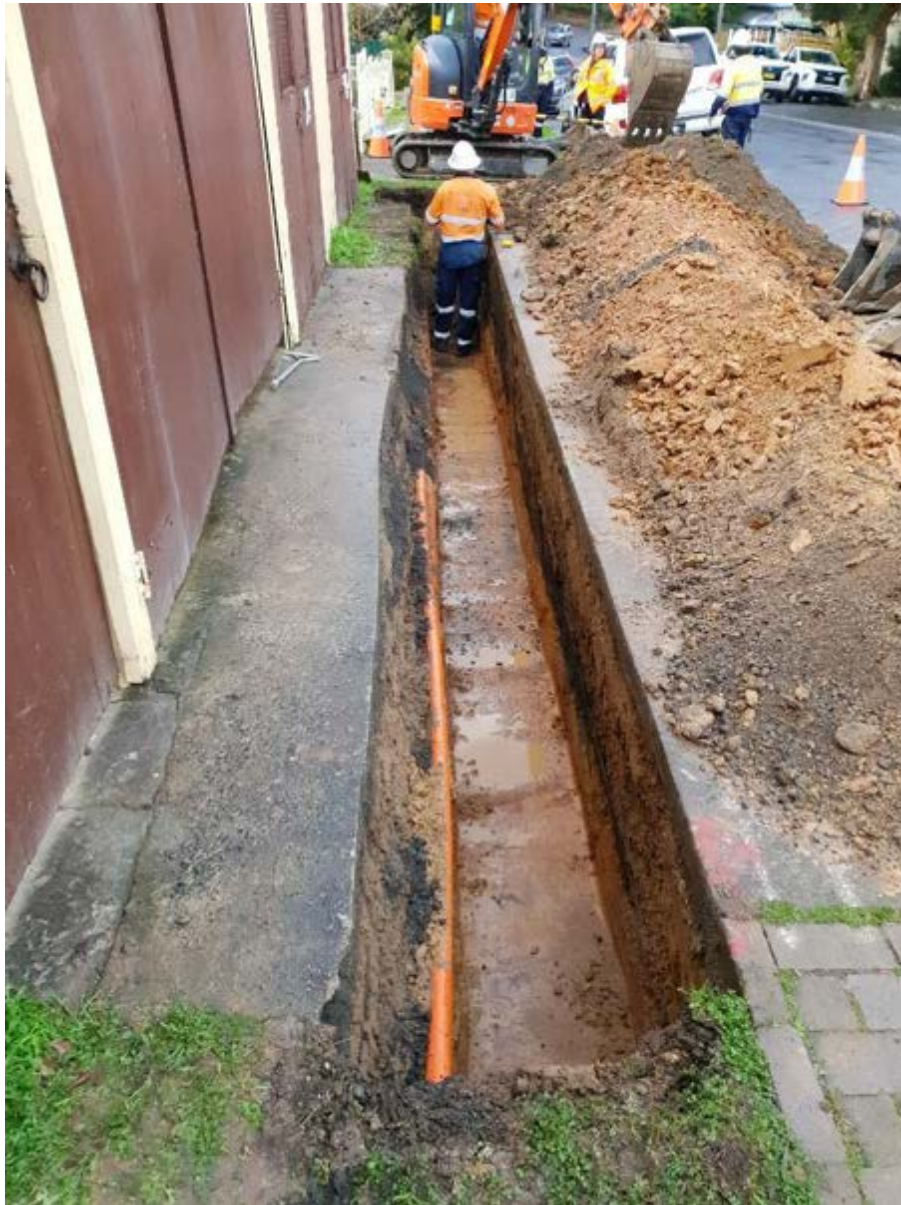
Figure 4-60 East facing view on completion of the service trench.
