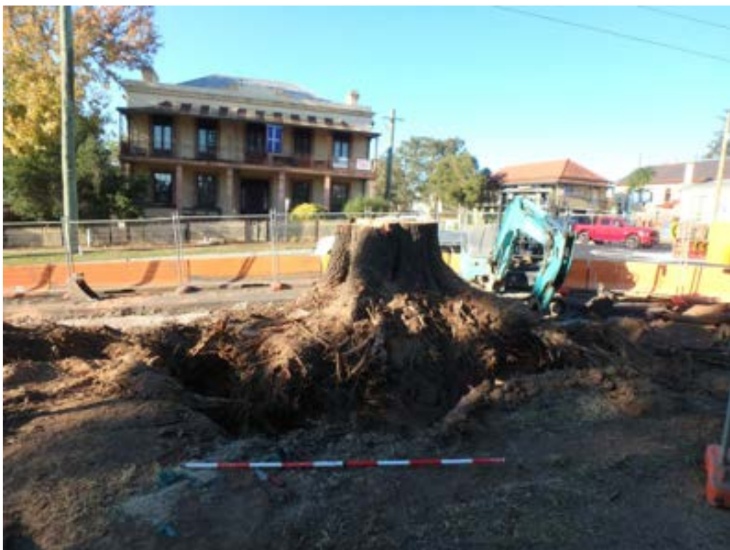
Figure 4-119 Tree stump during removal, looking southeast.
