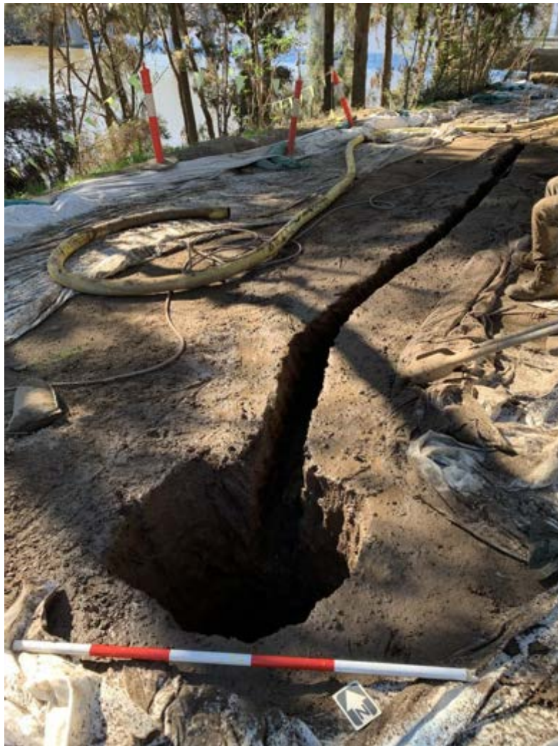
Figure 4-125 Trench excavated for a power cable and pit for new light pole, looking northeast.
