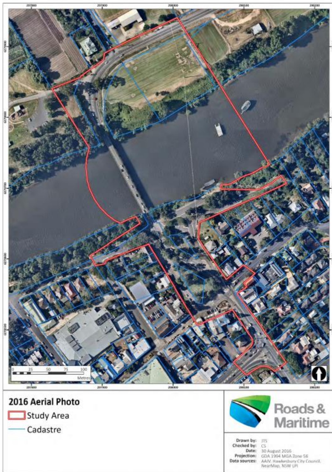
Figure 2-46 2016 aerial image of the study area. The current cadastre is shown in blue (Source: LPI, Overlay by Tom Sapienza, 2016).
