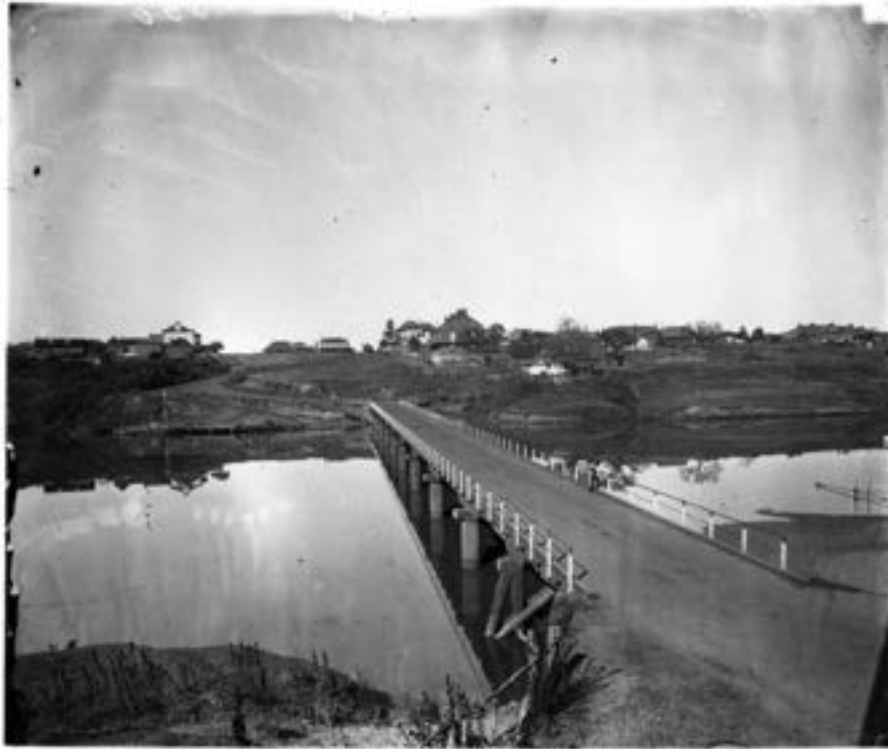
Figure 2-26 Windsor Bridge, Windsor, 1900 (sic), c.1879. View shows the bridge in its pre-1897 form. (Source: NRS-4481-3-[7/16220]-Sh1652 - Government Printing Office 1 – 06263).
