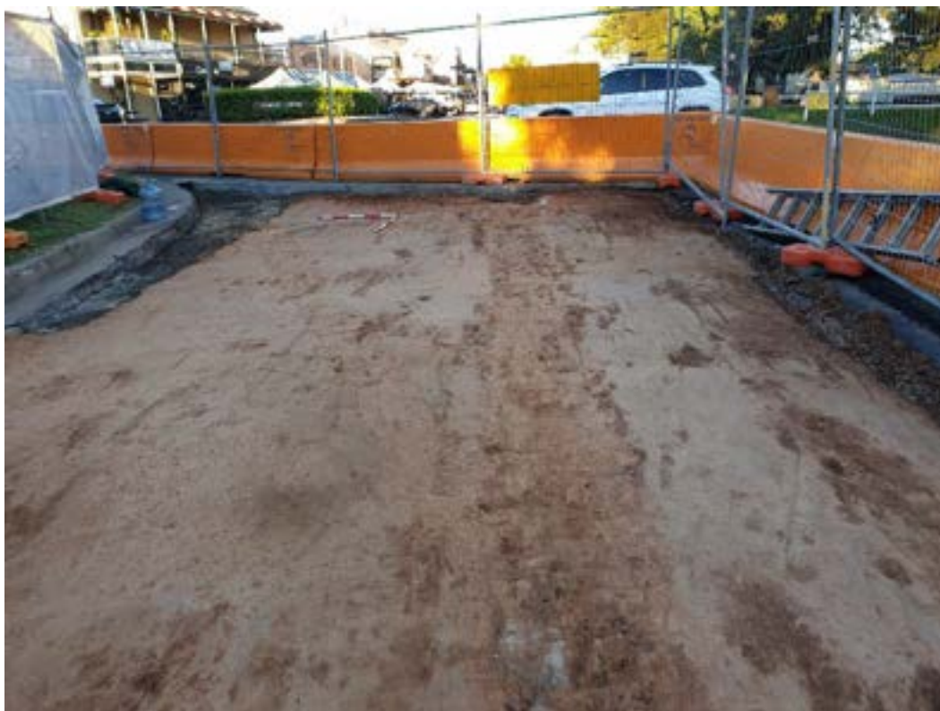
Figure 4-70 West facing view showing service cuts [403] on the right and [405] on the left, with service cut [403] cutting the wall [409] in the distance.
