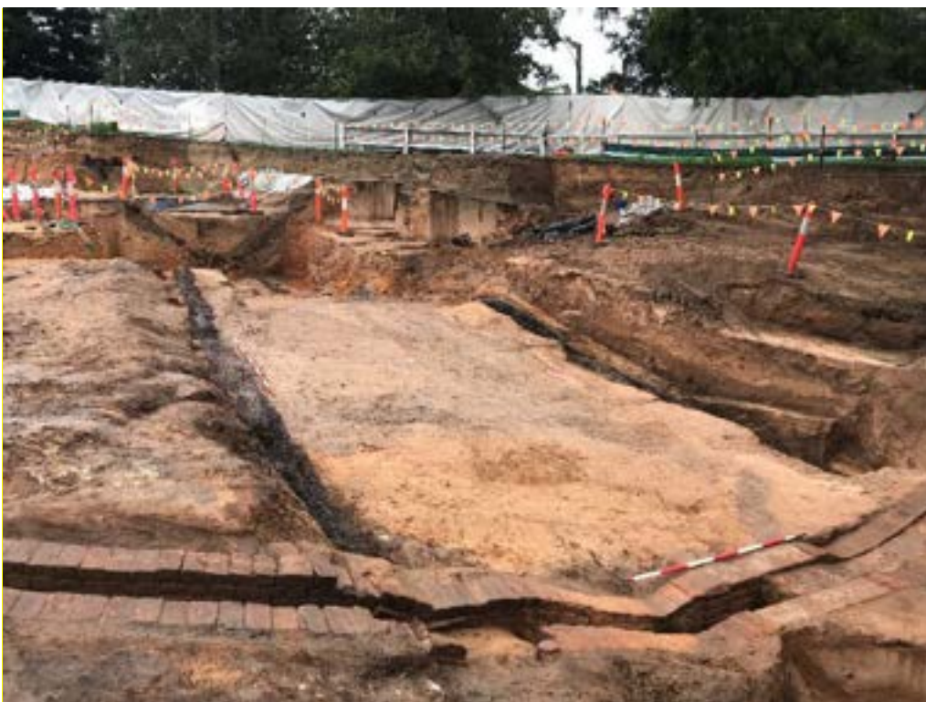
Figure 1-7 View looking south-west showing the northernmost of three brick box drains (foreground) that emptied into the main oviform drain.
