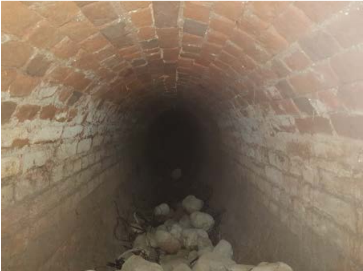
Figure 4-5. View within the oviform drain following removal of internal fill.
