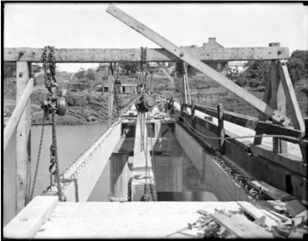
Figure 2-29 Windsor Bridge, 28 November 1921. Beam replacement, looking east (Source: SRNSW NRS-4481-4-88-[AF00184635] Department of Public Works).
