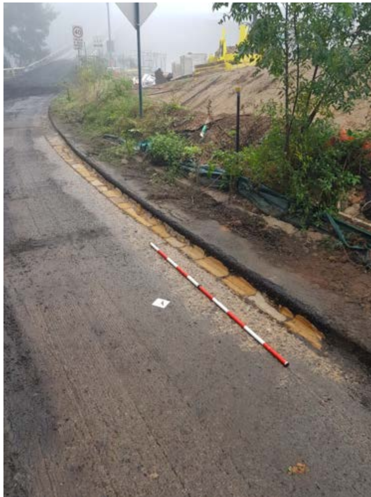
Figure 4-105 Bridge Street upgrade showing extent of exposed long gutter blocks, looking south.
