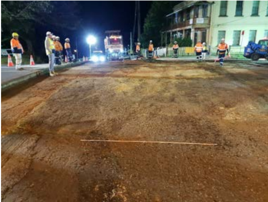
Figure 4-75 View showing completion of works on south-bound lane, looking north.
