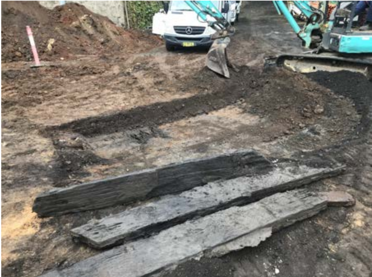
Figure 4-128 Timber boards following removal and scrape across site, looking southwest.
