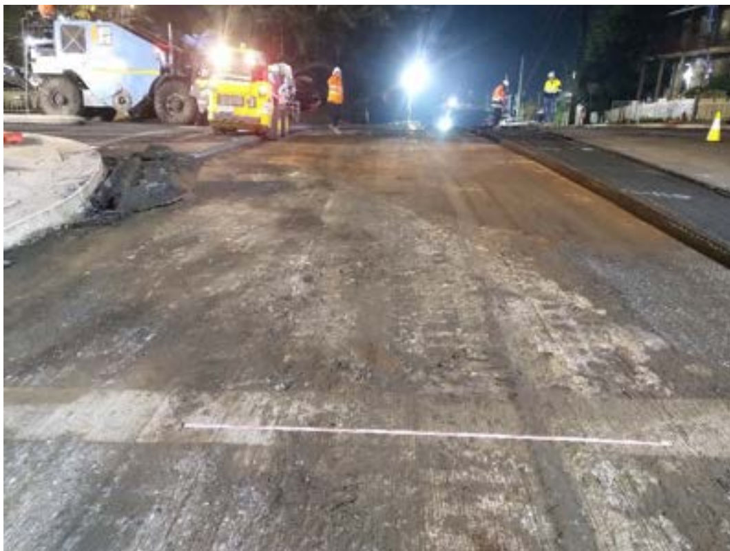
Figure 4-74 Northwest facing view across the Bridge Street/George Street intersection showing depth of excavation at completion of works in Area 3iii. Note the limit of the Macadam roadbed (right) along Bridge Street (foreground), discussed further below.
