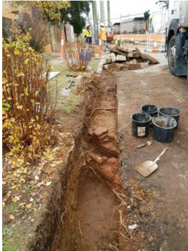
Figure 4-19 Box Drain 1 [2234] during excavation within alignment of Telstra trench, looking south.
