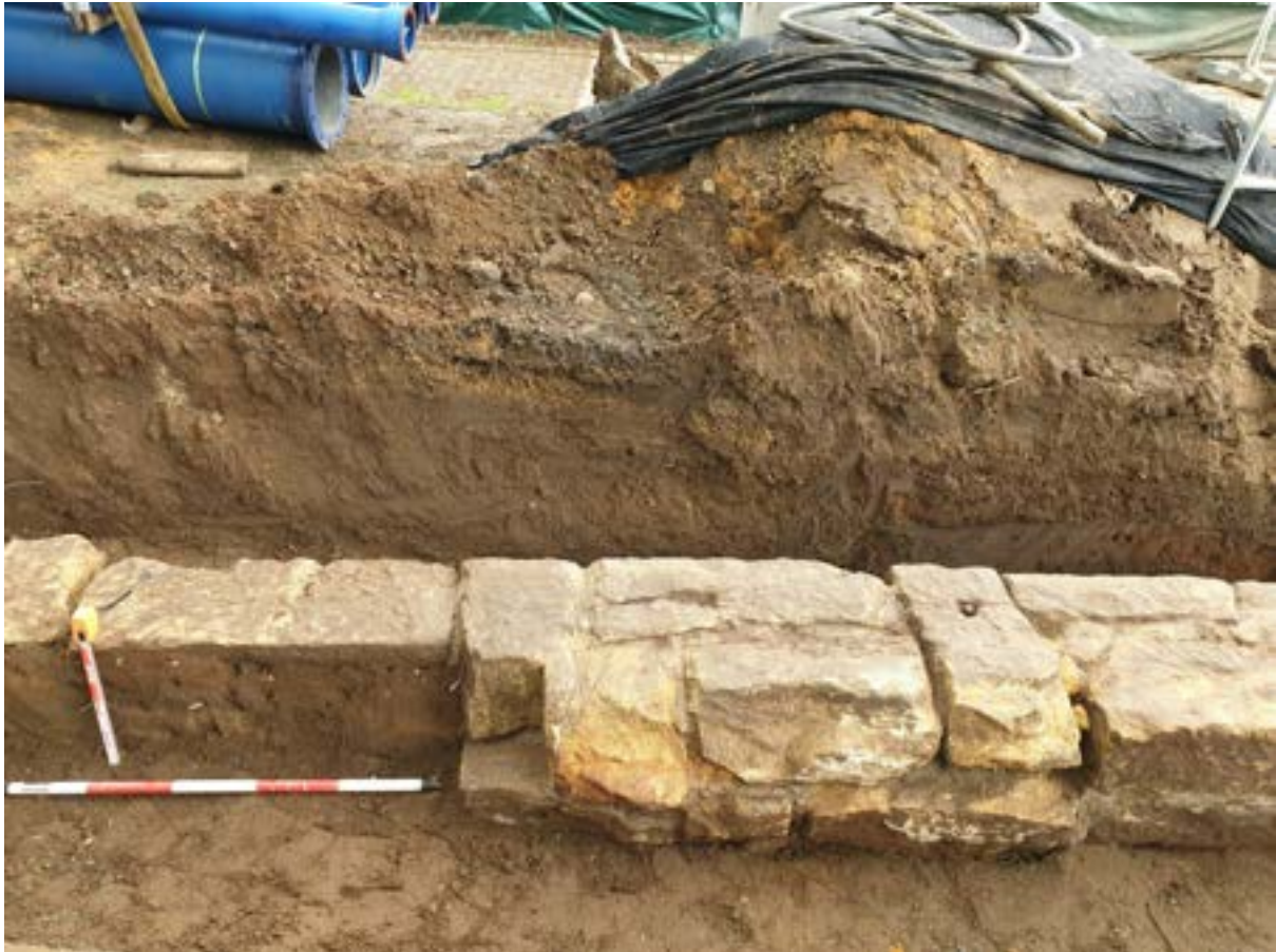
Figure 4-115 North facing view showing abrupt western end of wall, with additional stones laid on underlying silt to the west.
