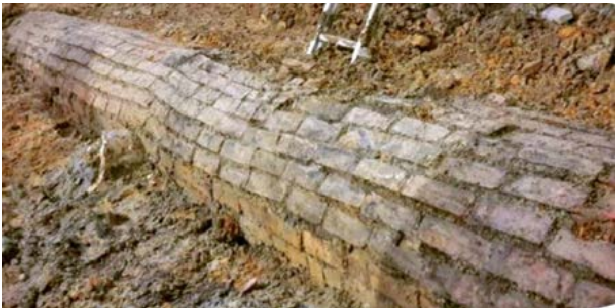
Figure 16 - Oviform brick drain (circa 500x700mm) found in Auckland, NZ, dating from c1865. ( https://www.cityraillink.co.nz/crl-heritage/ )
