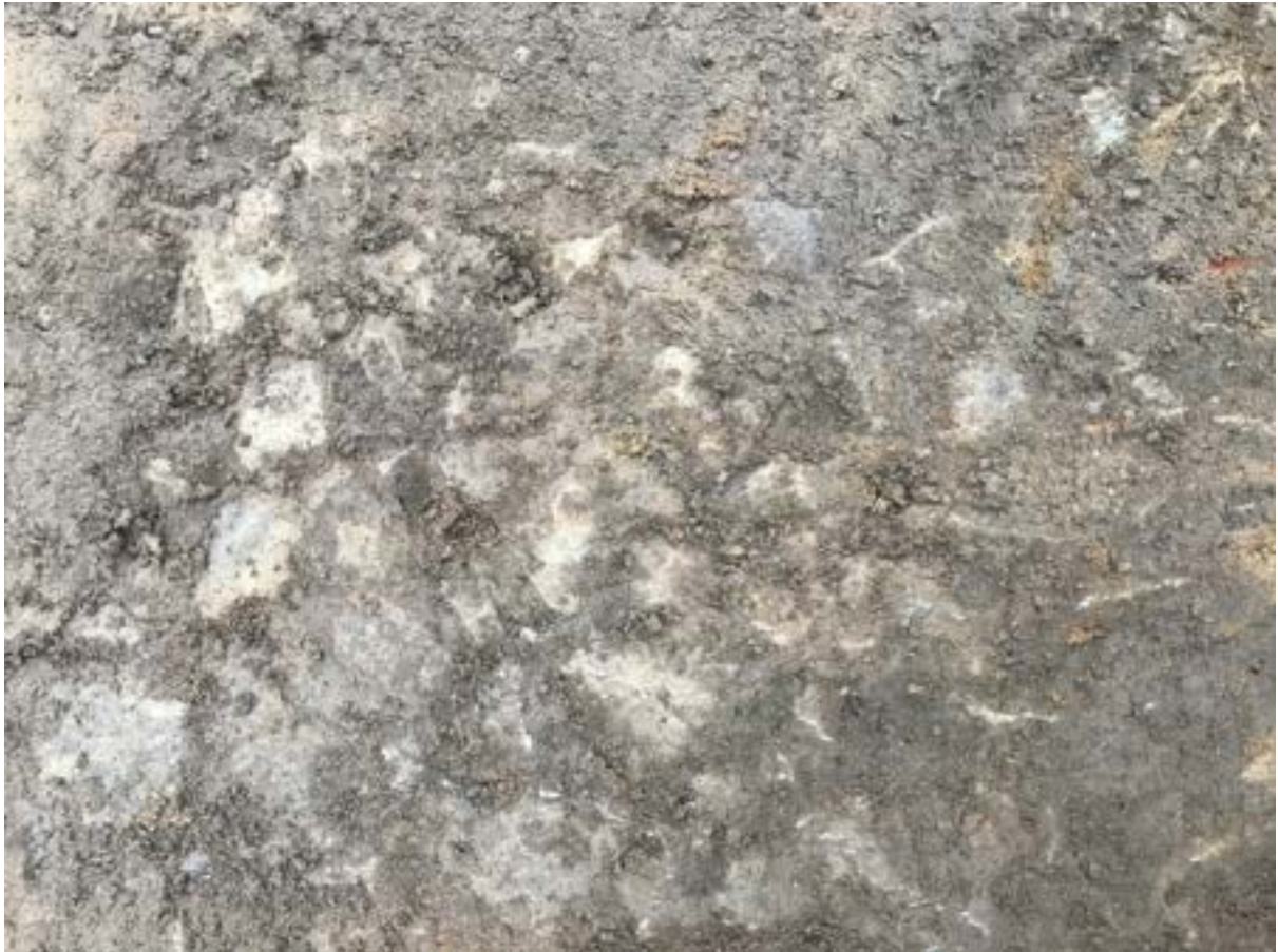
Figure 4-129 Detail of surviving patch of gravel roadbed.
