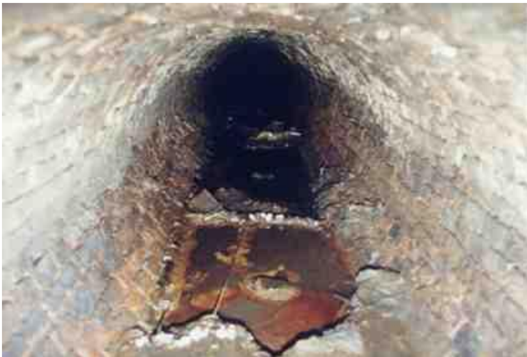
Figure 10 - Intact section of the Port Macquarie barrel drain (Source: E. A Higginbotham and Associates (2009))
