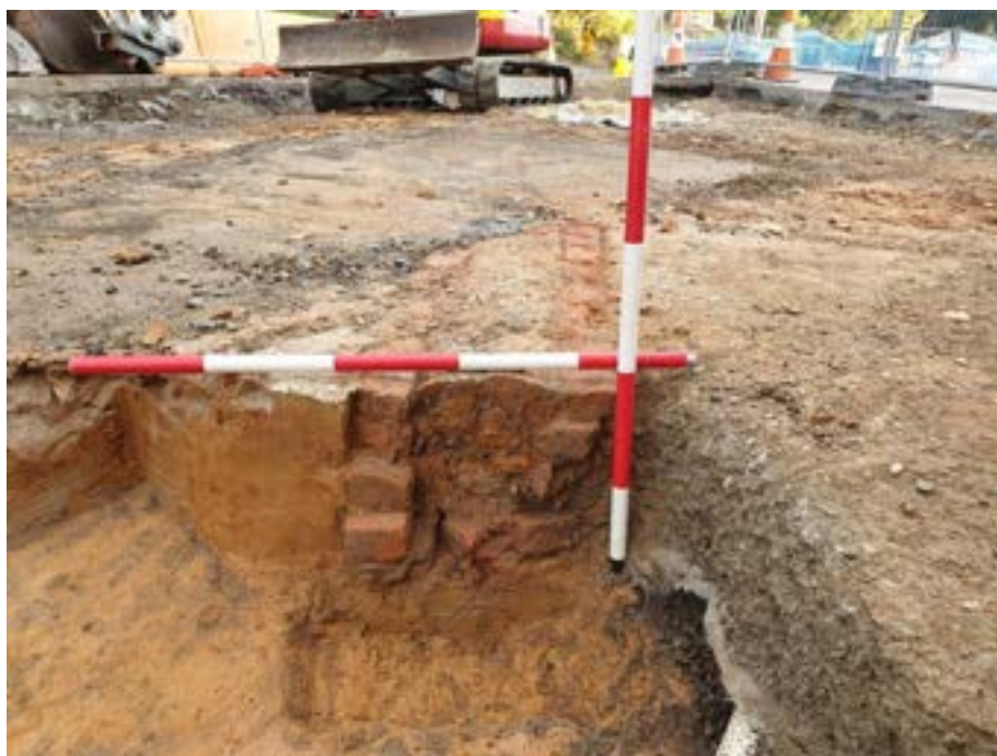
Figure 4-33 View showing cross section of Box Drain A following removal of gravel [2211], looking northwest.
