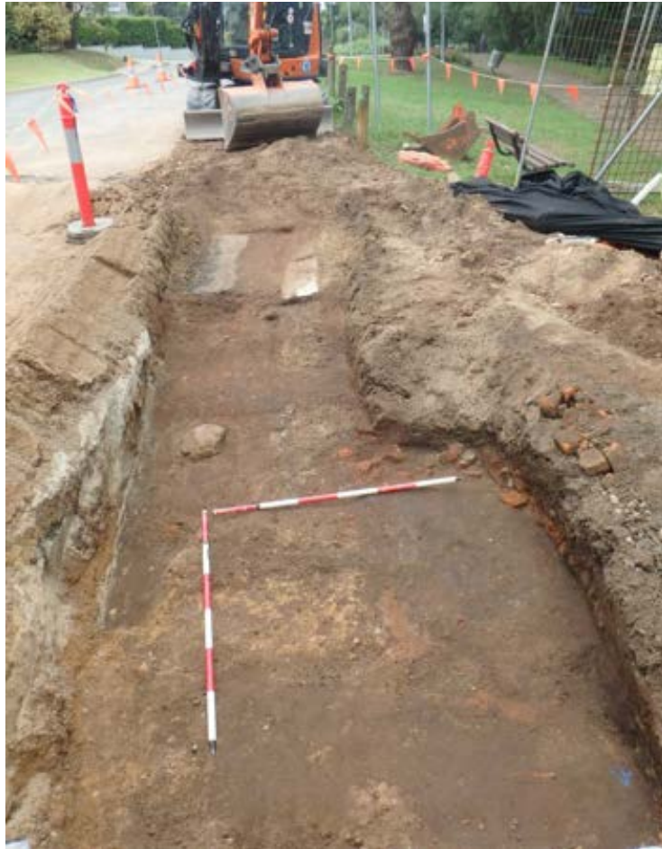
Figure 4-122 View of archaeological remains identified during service installation on the lower Terrace, looking west.
