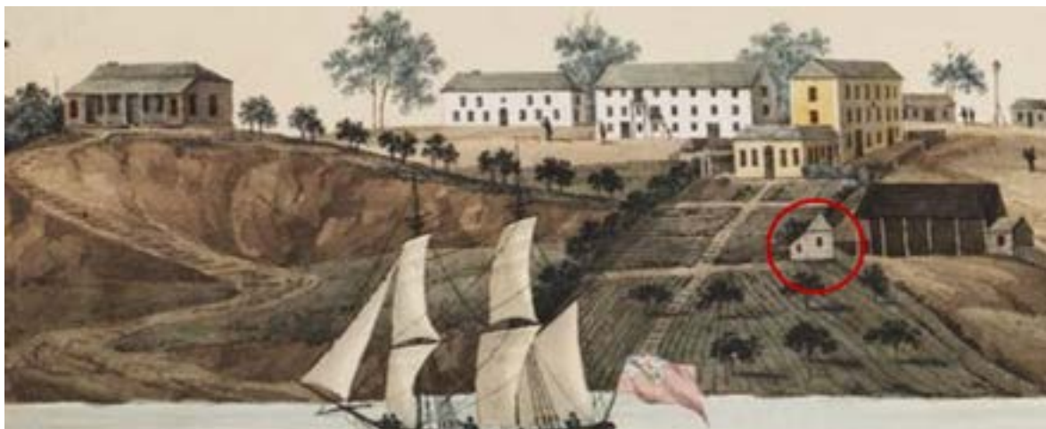
Figure 2-6 Detail of GW Evans' 1809 painting showing the eastern side of the government precinct. From left to right: the 1798 Government Cottage, 1803 Schoolhouse & Church, 1803 Government Granary, and Thompson's buildings and garden are seen bordering the open ground of what would become Thompson Square to the right. Thompson's small cottage (circled) that he occupied as constable is shown next to the obsolete 1798 granary and attached guardhouse. (Source. GW Evans, watercolour, 1809, 'Settlement on the Green Hills', State Library of NSW, Mitchell Library, PXD 388, vol. 3, fol. 7).
