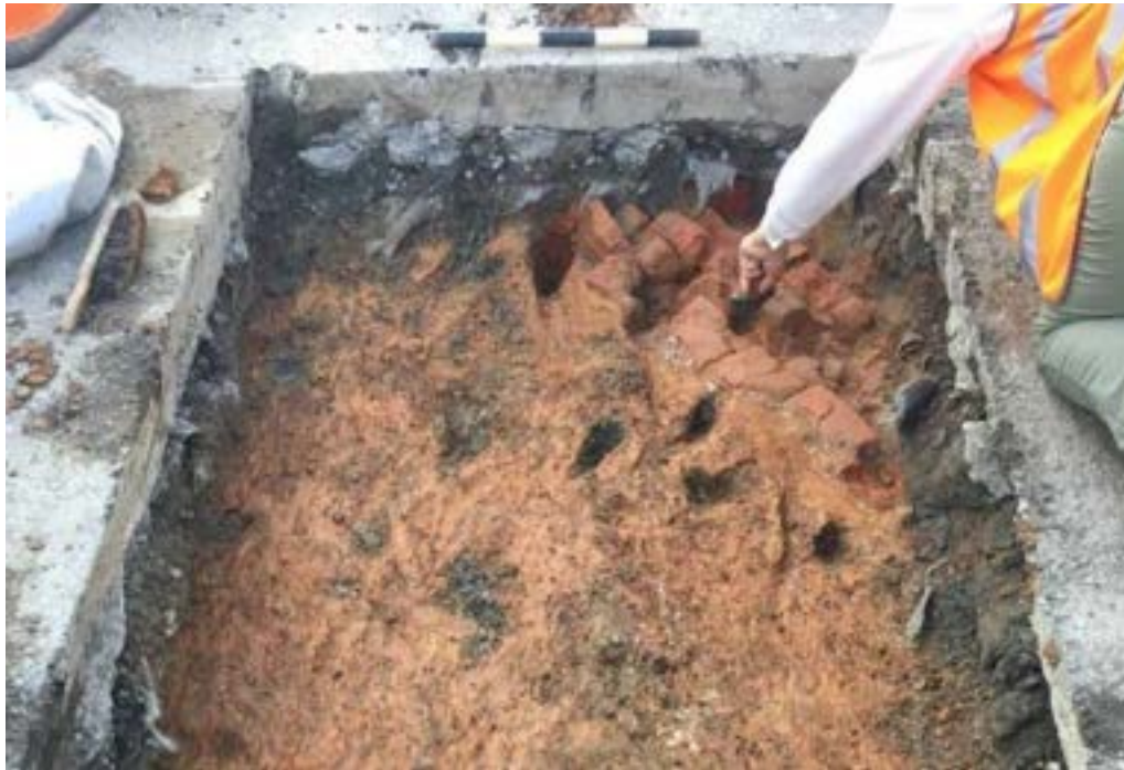
Figure 1-4 Early-nineteenth century box drain identified beneath Old Bridge Street (test pit SA 26).
