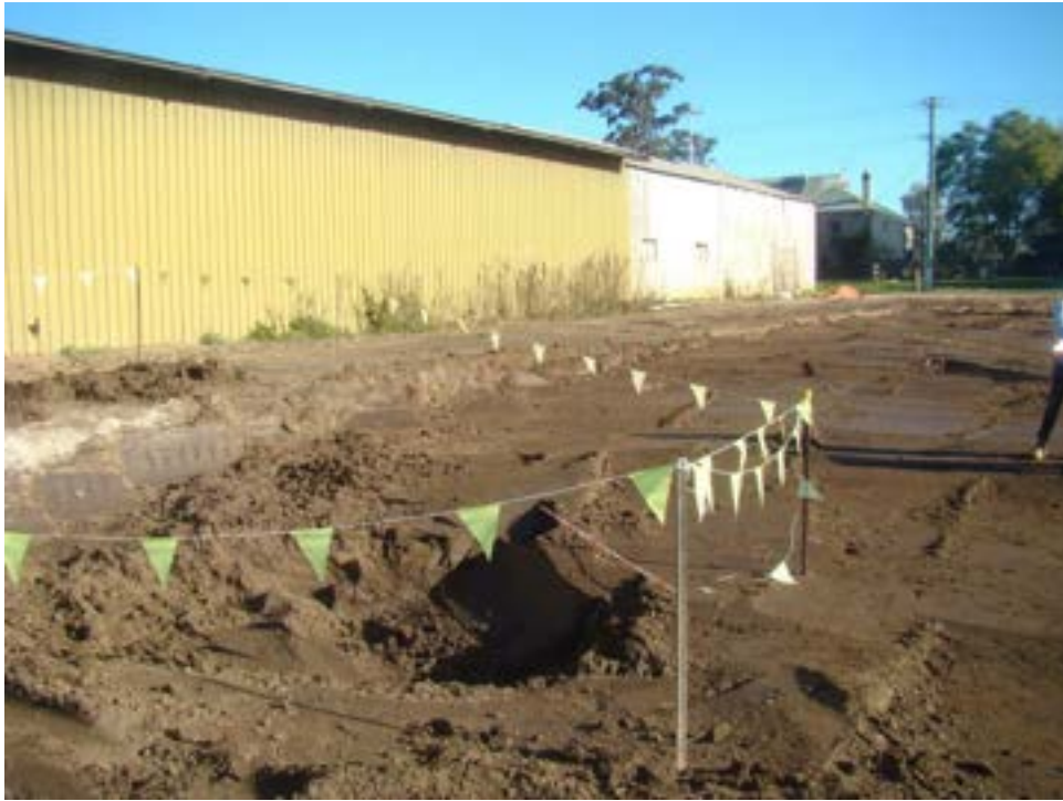
Figure 4-101 View looking southwest showing the fenced off location of the rubbish dump post excavation.
