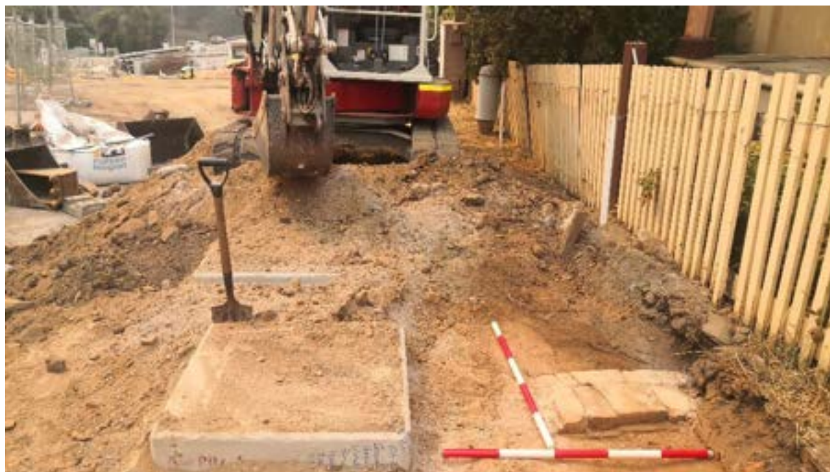
Figure 4-41 North facing view showing the location of wall [5030] at right in relation to prior excavation works.
