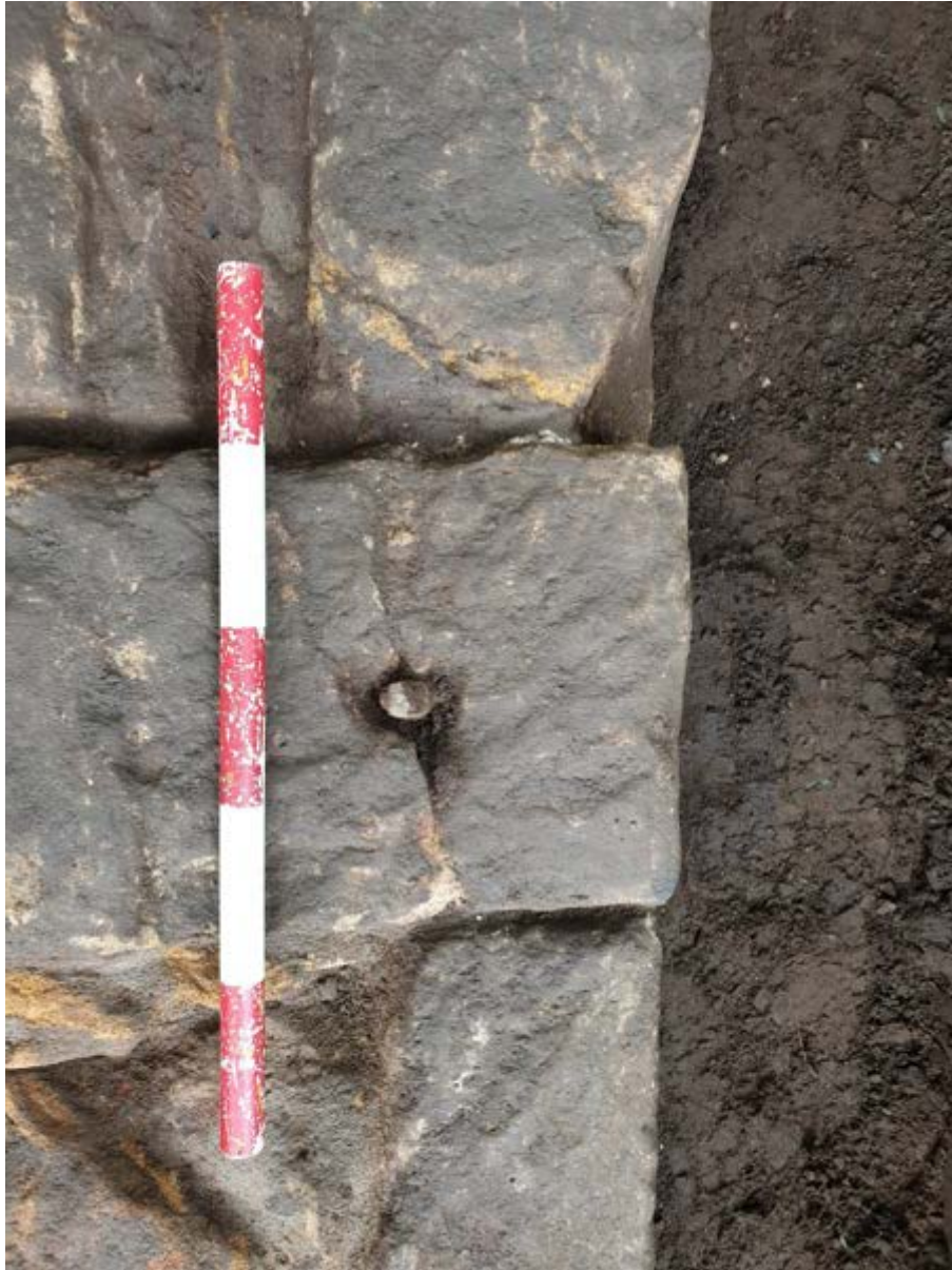
Figure 4-114 Detail of metal bolt inserted into the upper face of the wall.
