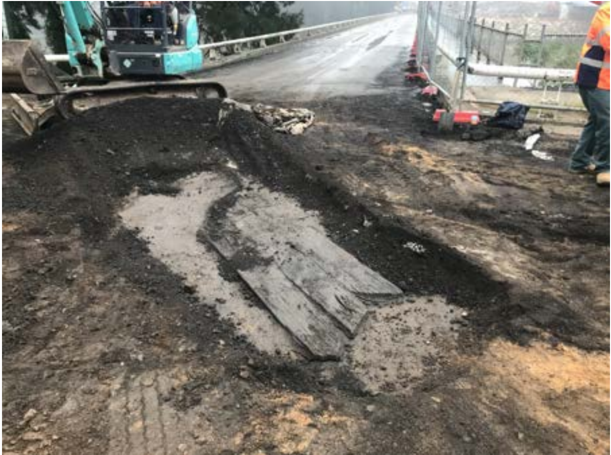
Figure 4-127 Timber boards in situ , looking north.
