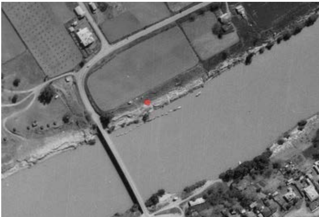
Figure 4-98 A 1956 aerial image showing the location of the pumphouse (NSW Spatial Services).
