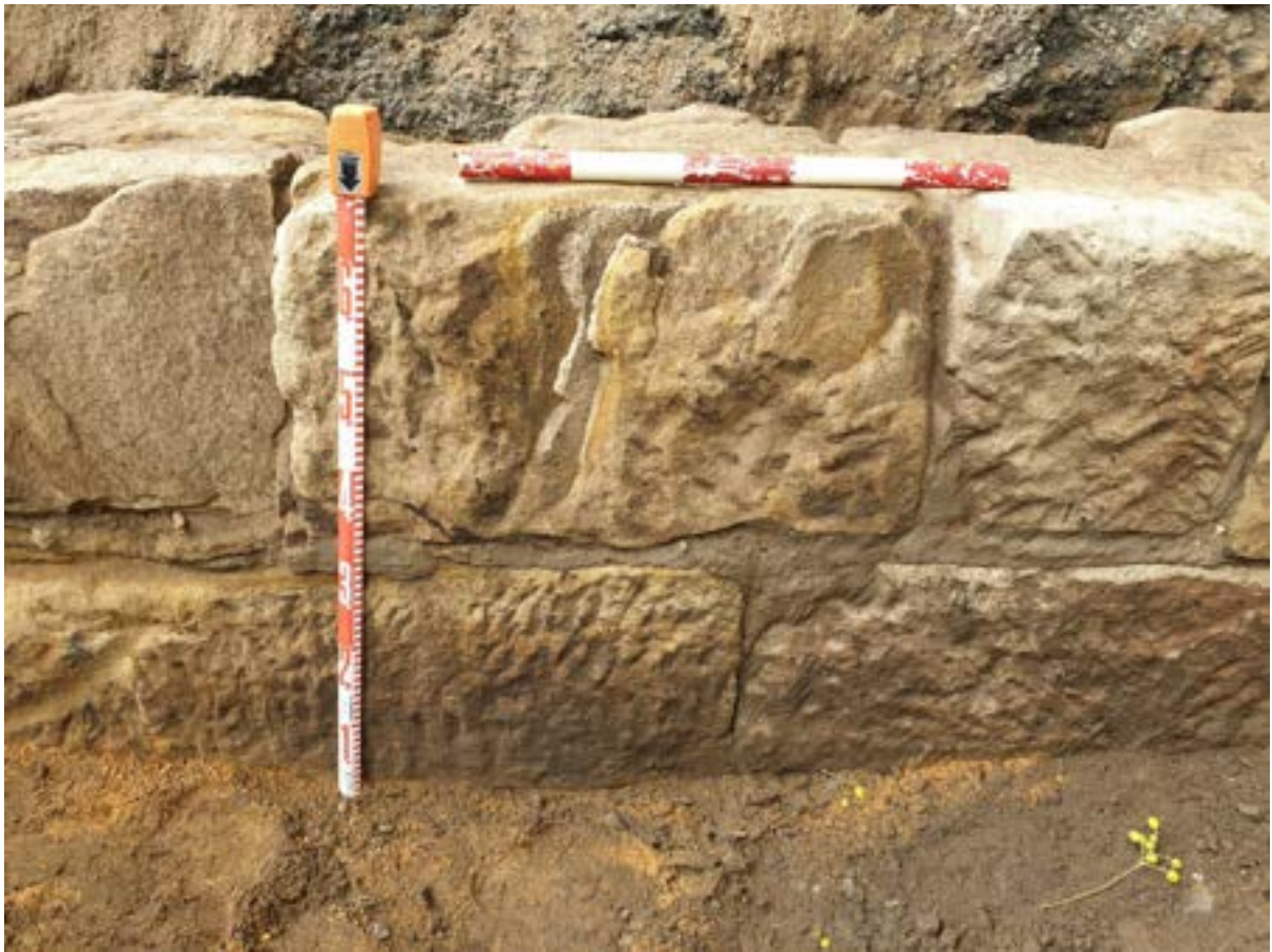
Figure 4-113 Detail of north face of wall.
