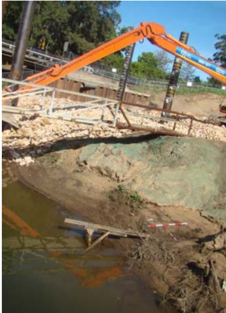
Figure 4-99 View looking west showing remnant timber frame of the former jetty.
