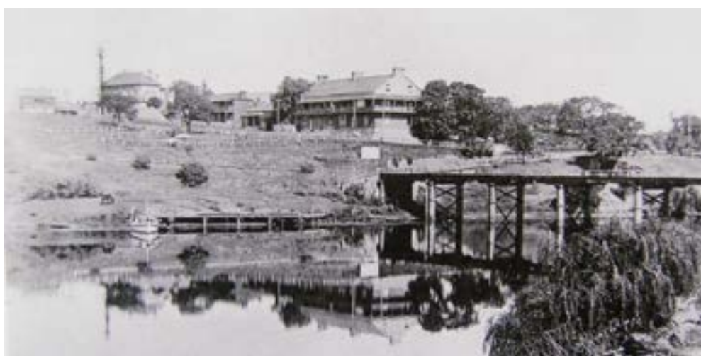
Figure 2-28 Thompson Square, the wharf and Windsor Bridge after 1904. The view shows the elevated bridge deck and the cutting for Terrace Road at right. (Source: State Library of NSW, Mitchell Library, Small Picture File).
