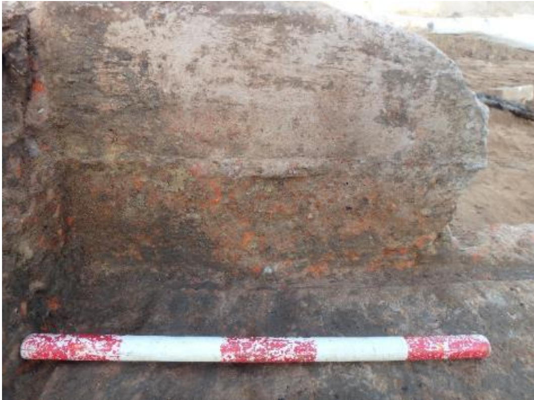
Figure 4-94 Interior elevation of concrete feature [601] showing evidence of timber formwork.
