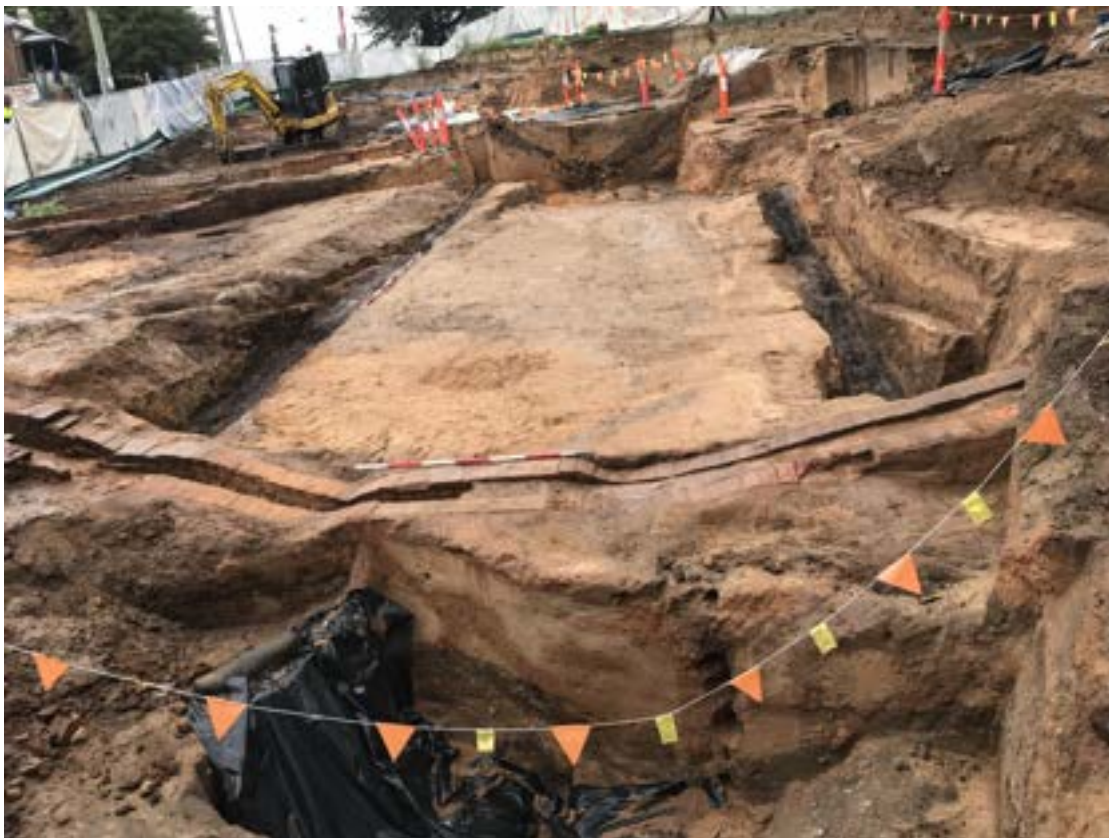
Figure 34 - Feeder line (foreground) crossing main drain showing slumping of the box drain above the shoulders of the main drain (Source: AAJV 2018)
