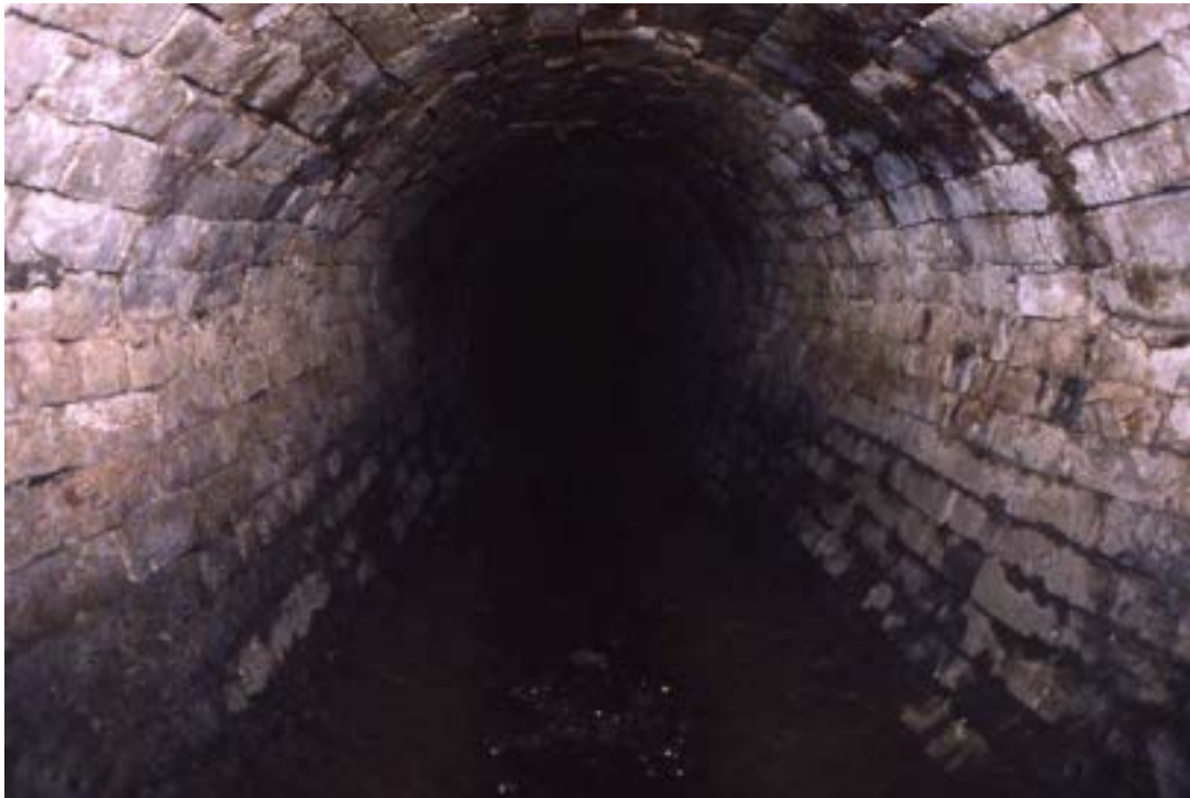
Figure 9 - A complete section of the brick barrel drain, 1822-27, Parramatta, NSW in 1981. (Source: E. A Higginbotham and Associates (1981))
