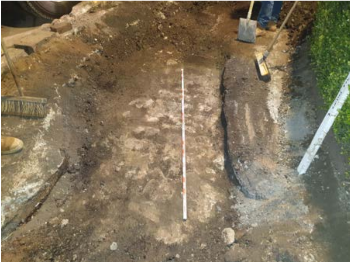
Figure 4-108 South facing view of Macadam roadbed identified during nightworks on the northbound shoulder land of Bridge Street.
