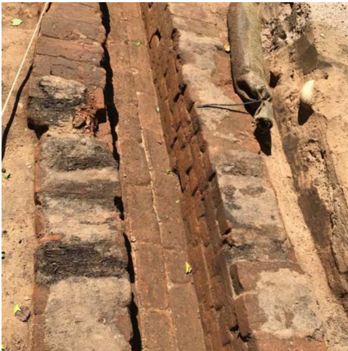
Figure 50 - A section of one of the box culverts with evidence of former timber coverings. (AAJV March 2018)
