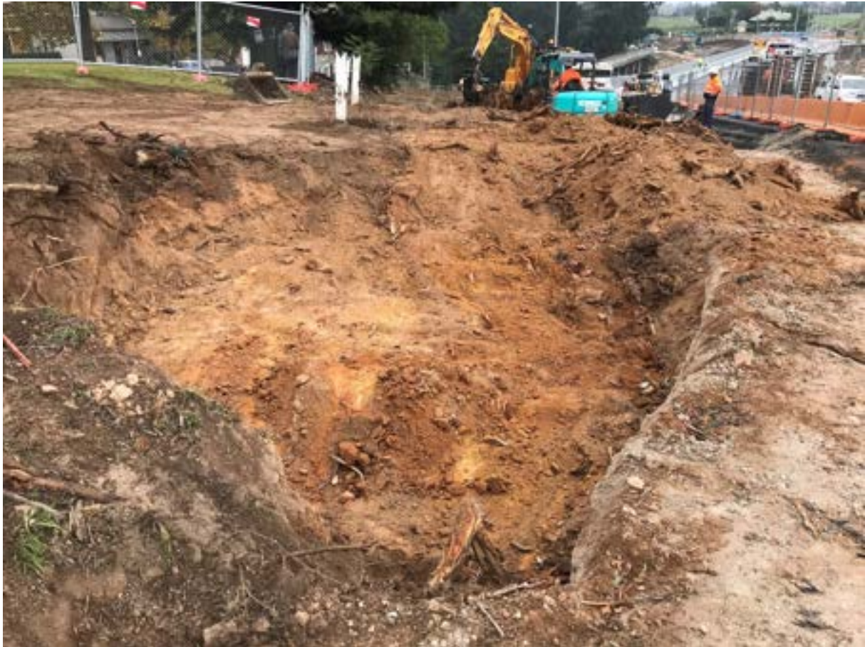
Figure 4-121 Site following removal of stump and roots, looking north.
