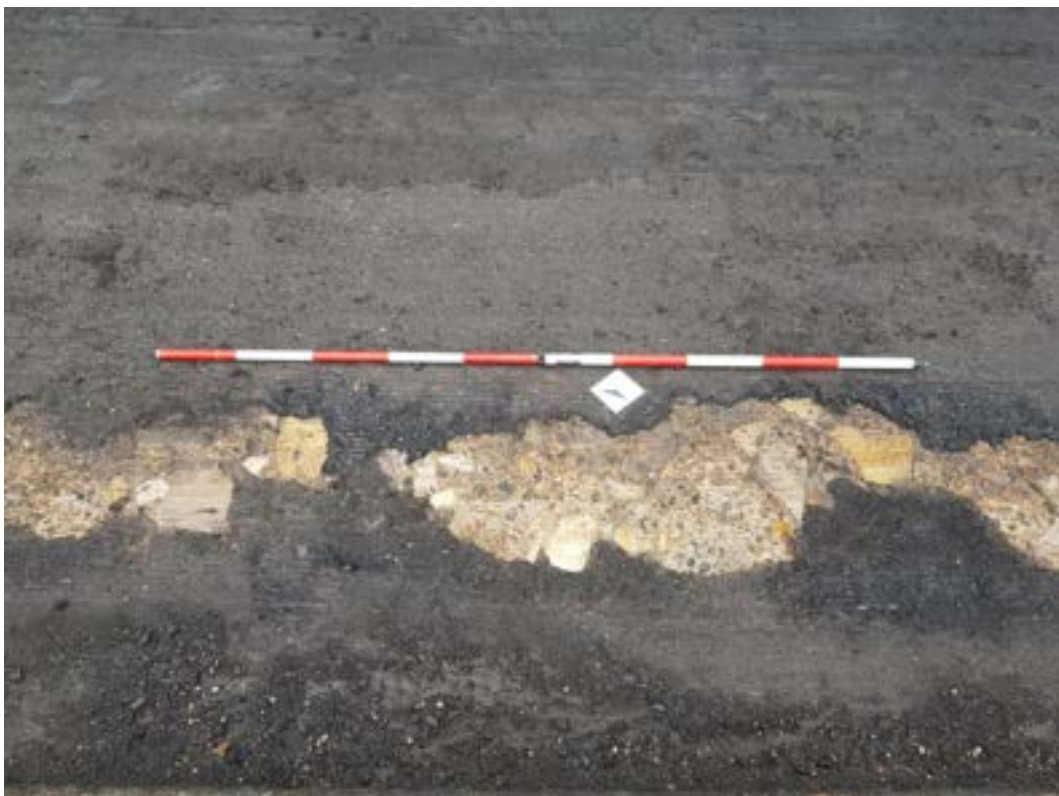
Figure 4-107 Detail of Macadam roadbed beneath the current asphalt surface mixed with later concrete bedding.
