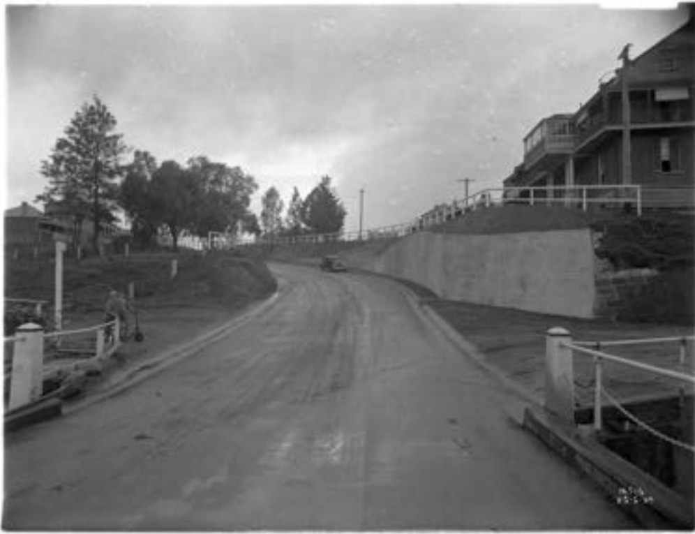
Figure 2-36 Windsor Bridge approach looking east, Hawkesbury River, 25 May 1934 (SRNSW NRS-4481-3-[7/16032]-St16516 - NSW Government Printer series: Main Roads: Main Road 165)).
