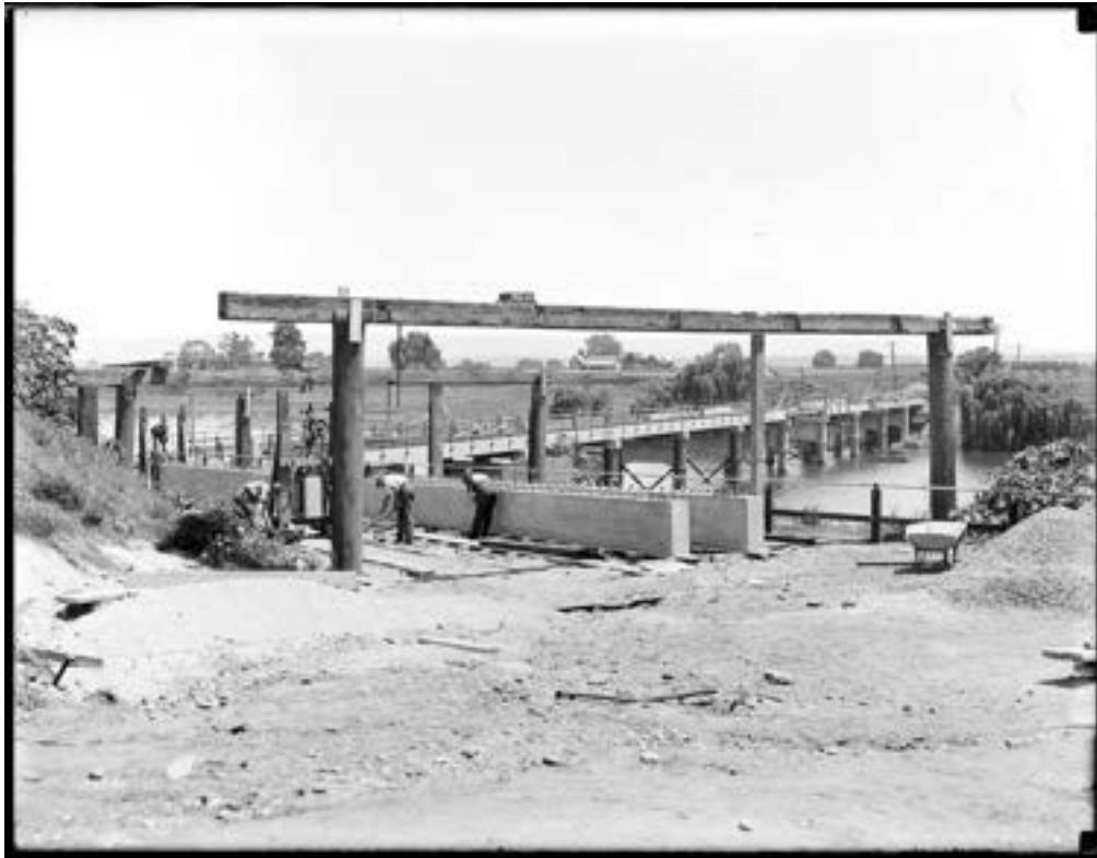
Figure 2-31 Windsor Bridge, 28 November 1921. Beam casting area (Source: SRNSW NRS-4481-4-88-[AF00196955] Department of Public Works).
