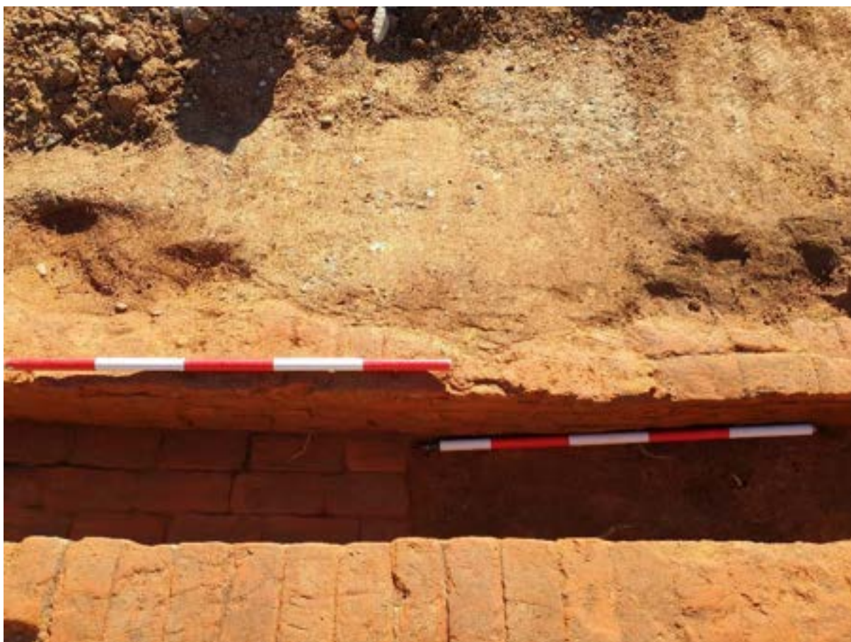
Figure 4-22 View of Box Drain 1 showing abrupt transition from brick-lined drain to clay lined base, looking north.
