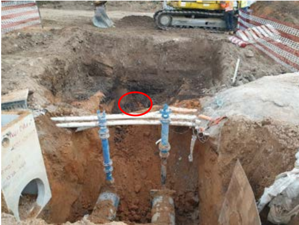
Figure 4-77 West facing view showing condition of trench upon arrival at site following activation of the UFP. Note brick fragments circled in red.
