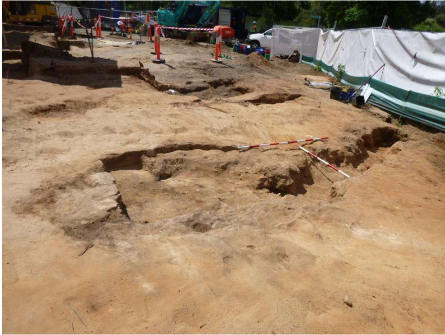
Figure 5.41 View north of one of several possible scoured out ruts within the lower eastern end of road surface 1046. Fill material is visible to the north in the background
