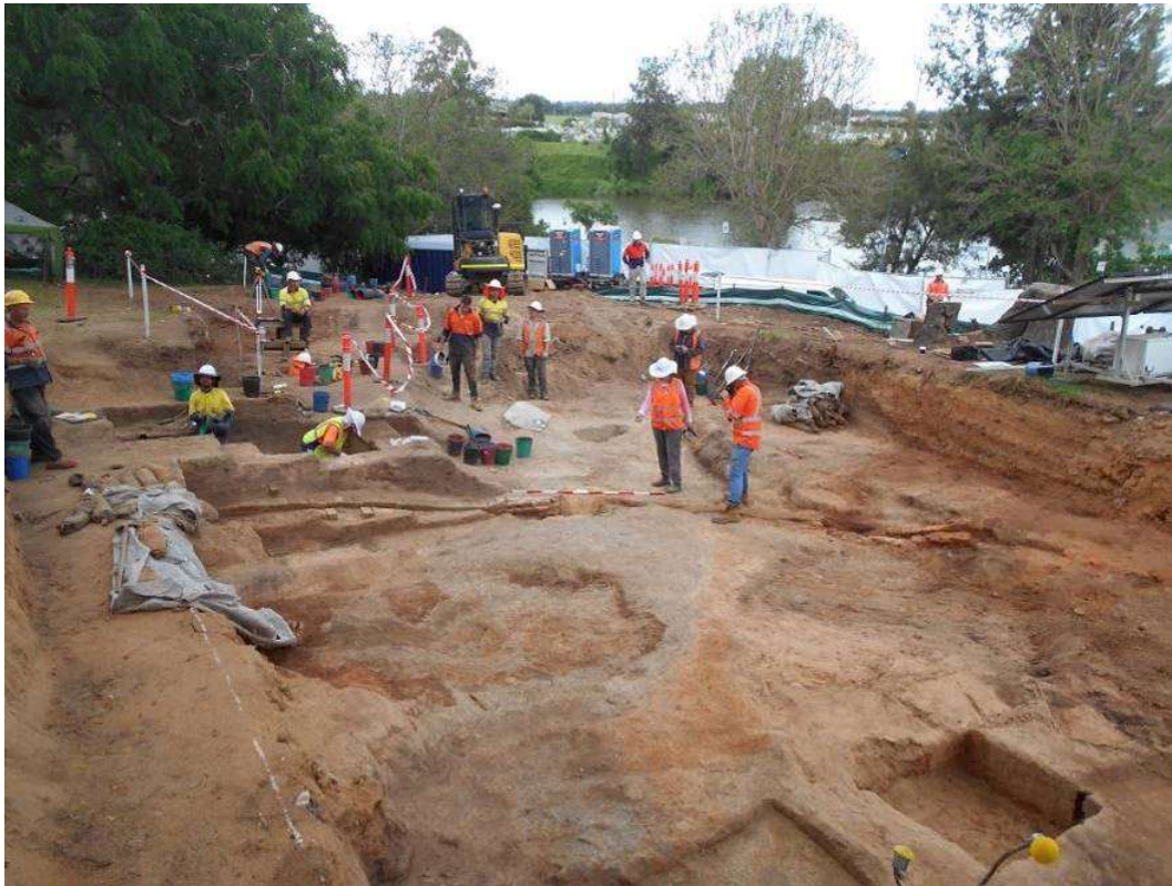
Figure 5.17 View north through the centre of the salvage excavation showing linear fill deposits running below box drain 2 (1047). The sump connecting the box drain with the oviform drain below is adjacent to the 1m metre scale at centre.
