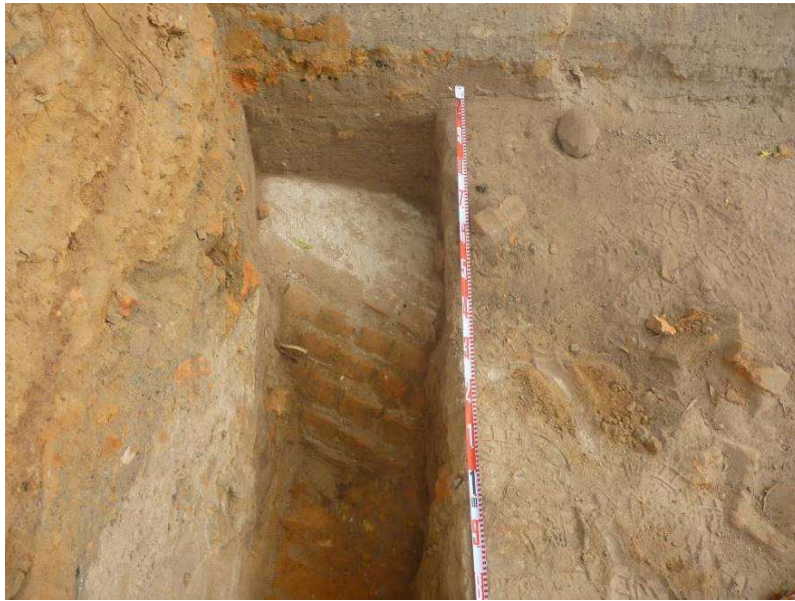
Figure 5.18 View west showing the crown of the c.1814 oviform drain (1115) exposed within Sondage 2.
