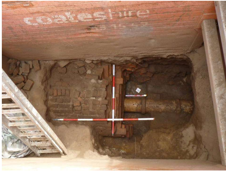
Figure 5.35 Oviform drain 1115 as seen in Sondage 6 from ground level. The inserted earthenware pipe and headwall are visible at the terminal point. The scale spanning the drain is 1.2 metres in length.
