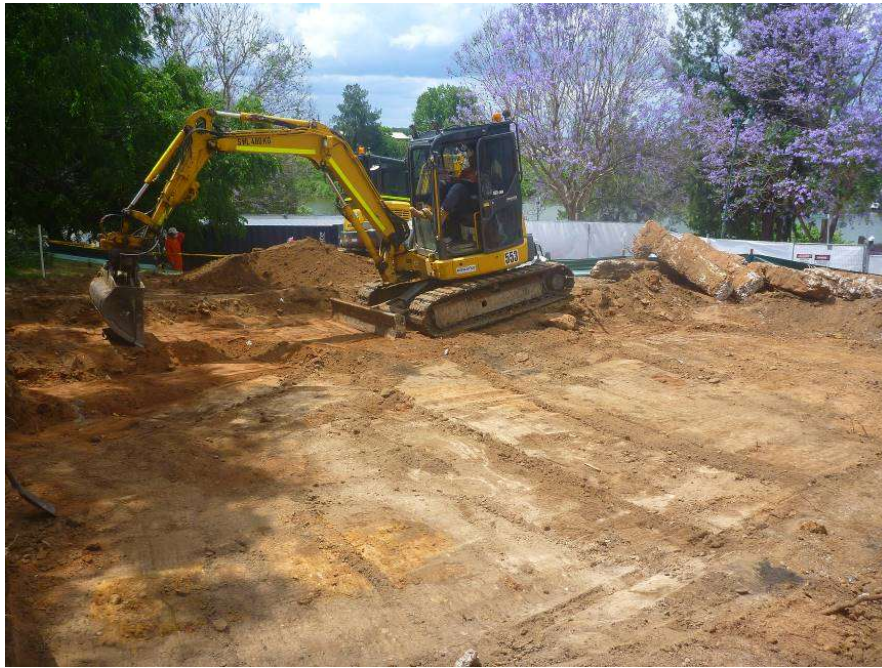
Figure 5.37 View north showing the initial exposure of the lighter grey-brown Phase 4 fill deposit 1014 that denoted the level of 19 th century lower Thompson Square.
