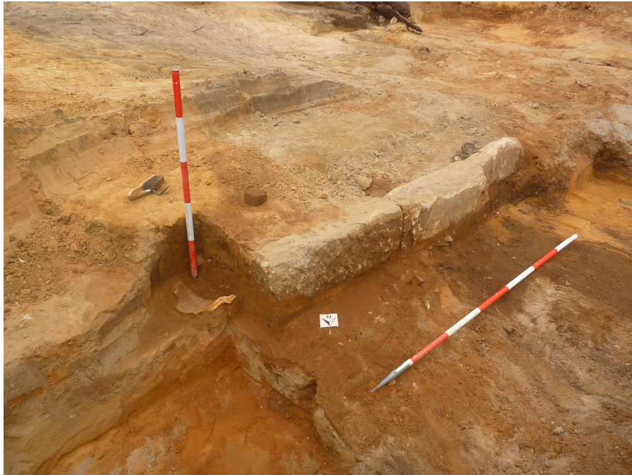
Figure 5.39 South facing view of sandstone kerbstones or trench lining blocks 1152 for vitreous ceramic pipe 1153.
