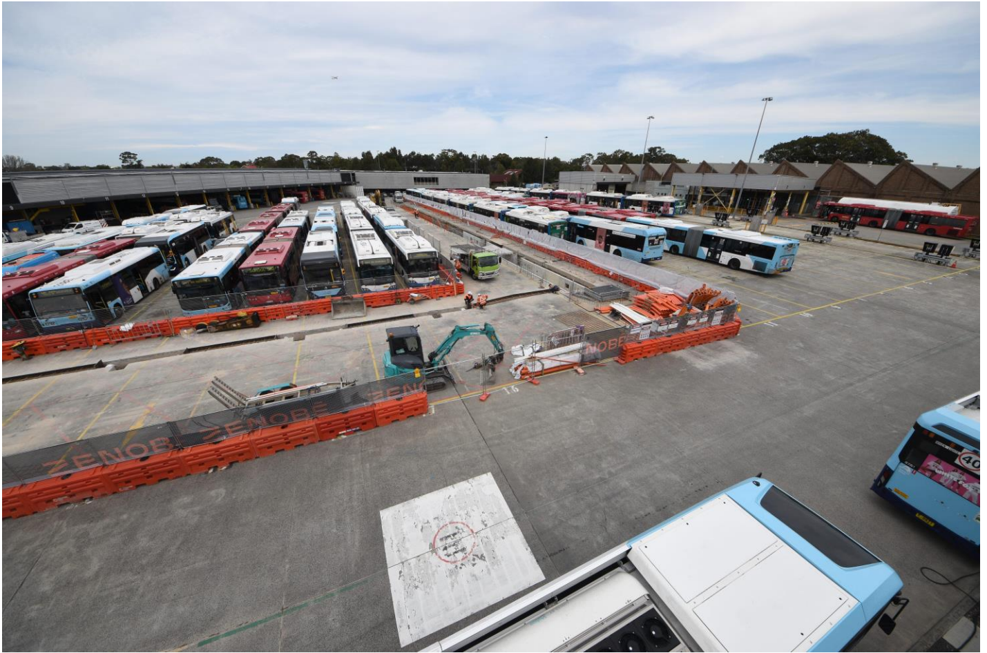
Caption: Electrical upgrades in progress within Leichhardt depot
