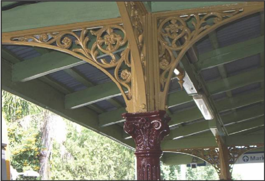
Figure 28 - Richmond Railway Station
