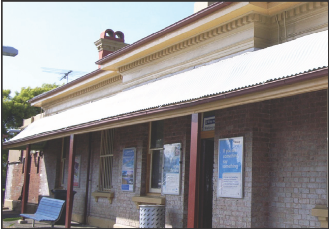
Figure 26 - Richmond Railway Station
