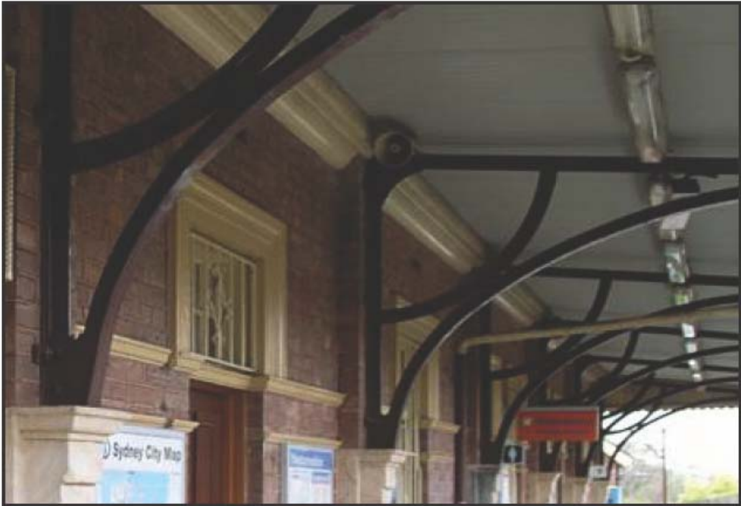
Figure 34 - Hazelbrook Railway Station – detail
