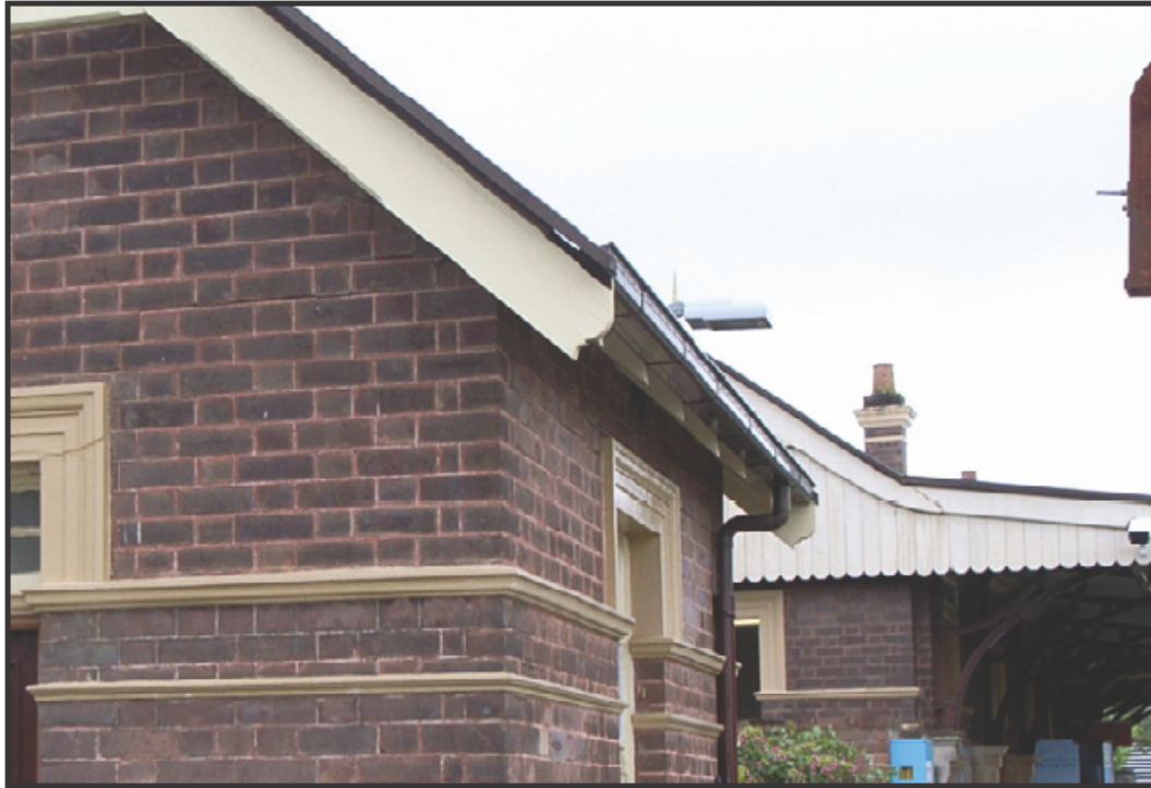
Figure 35 - Hazelbrook Railway Station – detail
