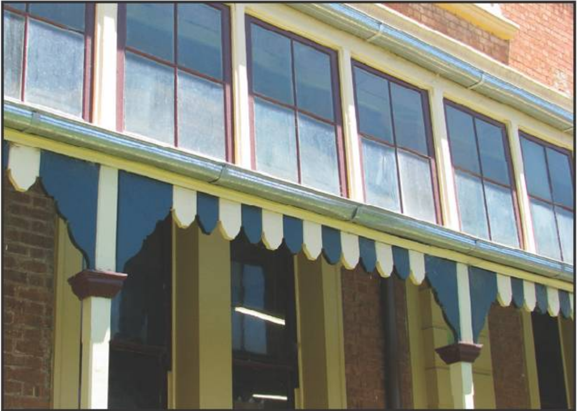
Figure 5 - Junee Railway Station detail
