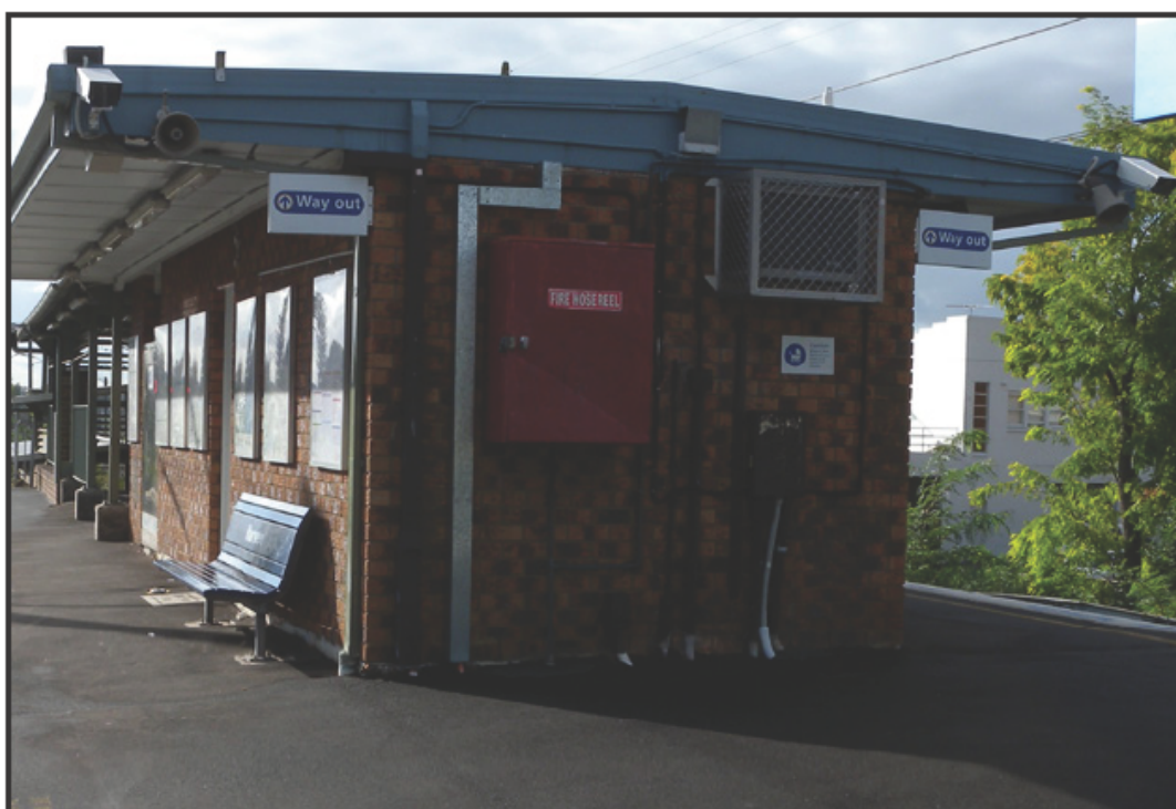
Figure 50 - Narwee Railway Station
