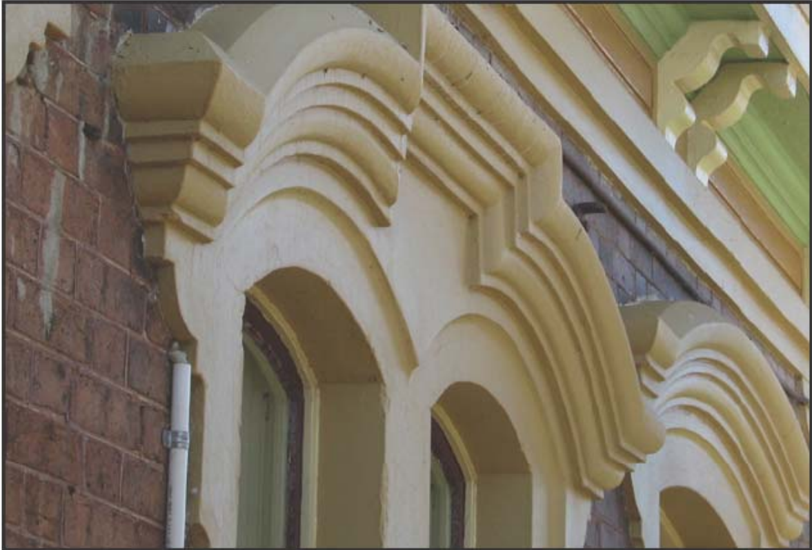
Figure 4 - Junee Railway Station detail
