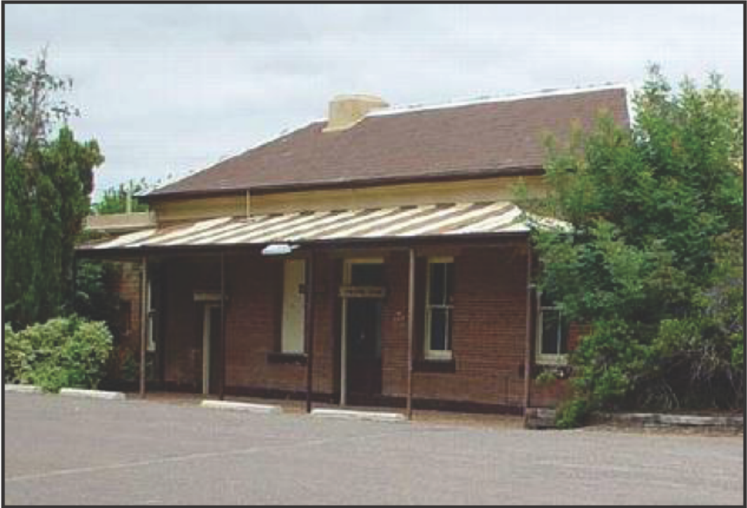
Figure 14 Scone Railway Station
