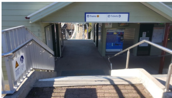
Stairs providing station access from The Strand/Meta Street
