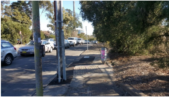
Poor pedestrian connection along northern side of Paisley Road
