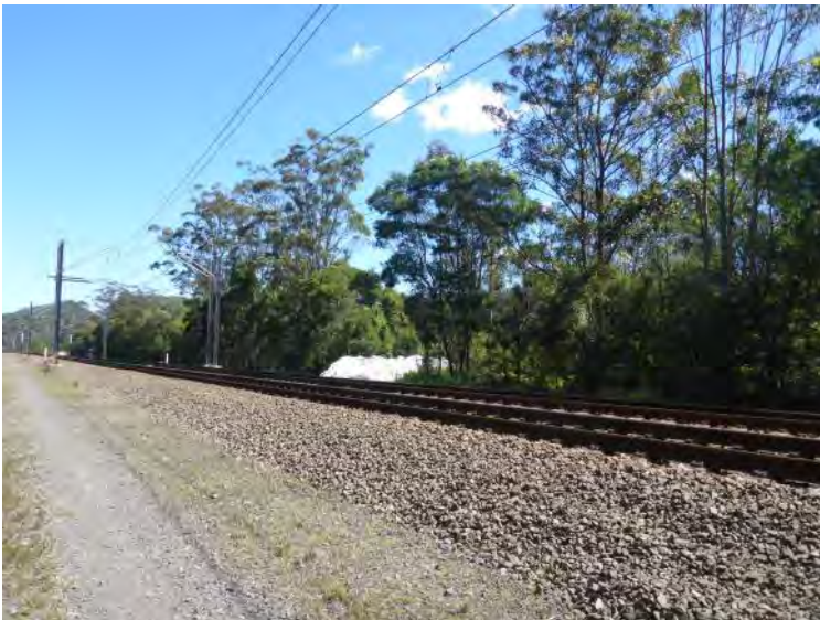
Plate 5 Disturbance within the existing rail corridor, view west
