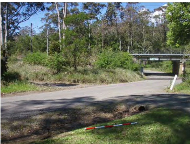
Plate 6 View of Turpentine Road railway underpass, view south-west, 1m scale
