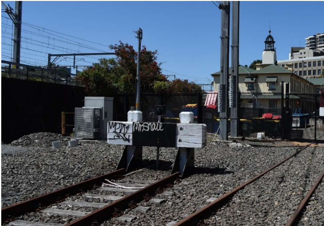
Figure 36 Hardwood buffer stop from west, Work Managers Office in background
