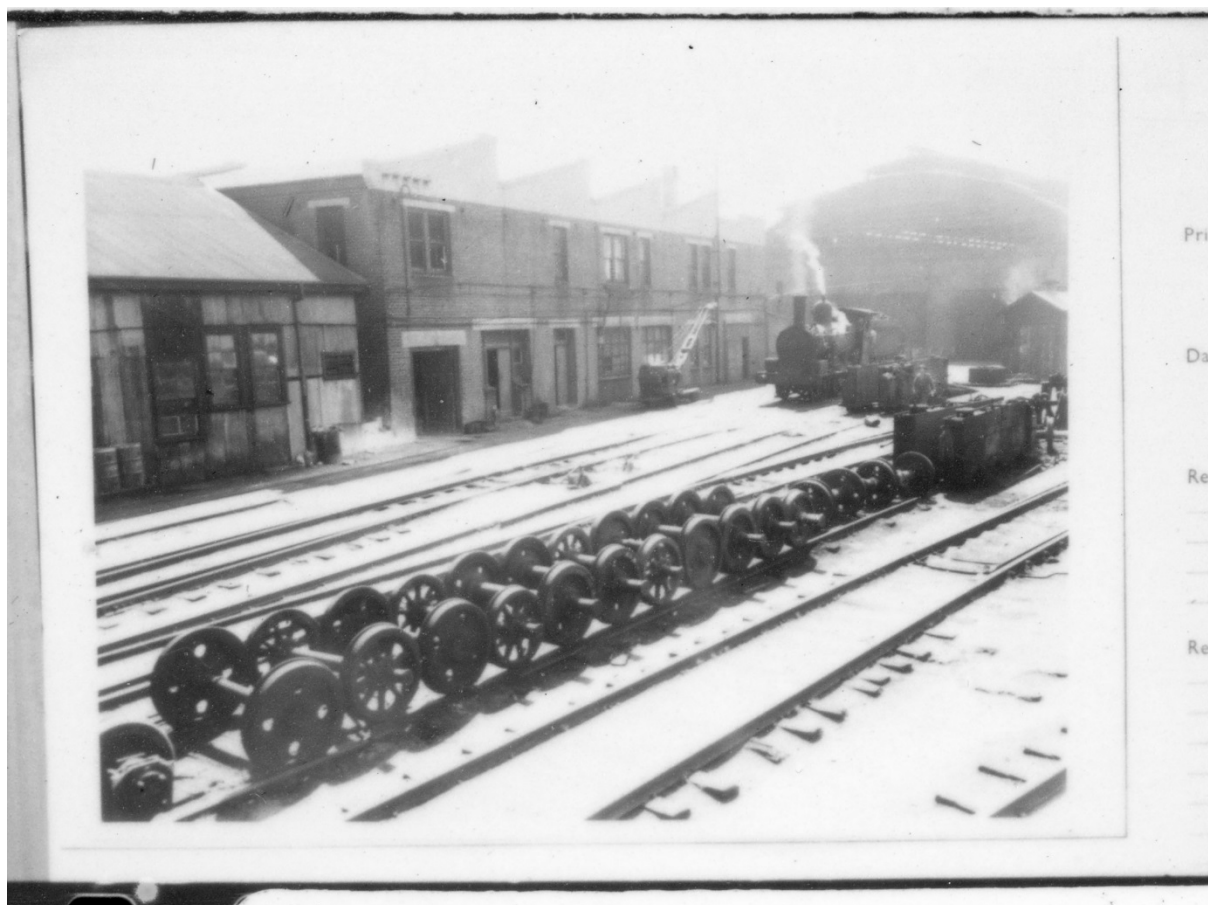
Former Engine Running Sheds – Subject Site 2
