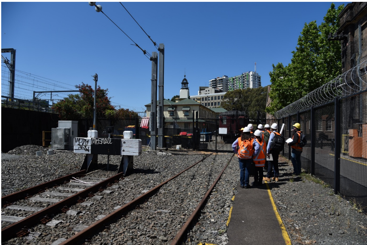
Figure 17: Rail siding north of Locomotive Workshops, with buffer stop and security fencing visible. East aspect.
