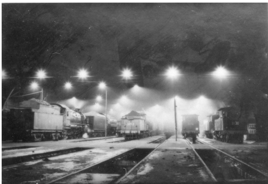
Figure 25: Photograph of the interior of the engine running sheds with train maintenance pits visible in foreground, 1930s, west aspect. (Source: Railway Resource Centre, Redfern)
