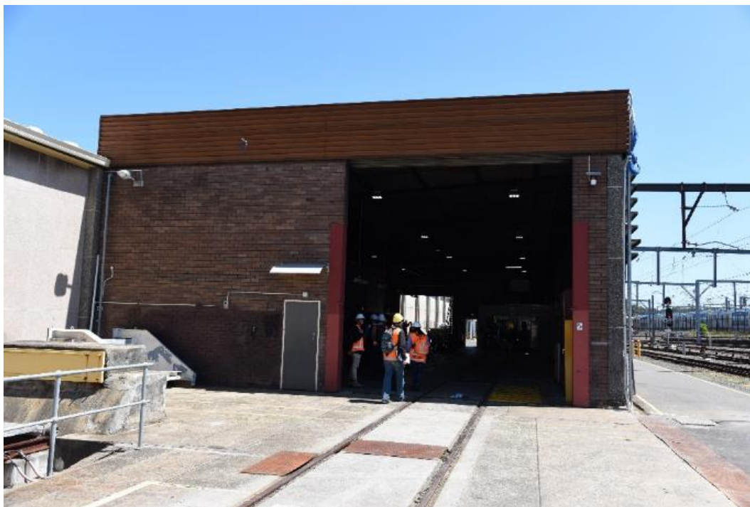
Figure 29: Welding Qualifications Centre, viewed from the east
