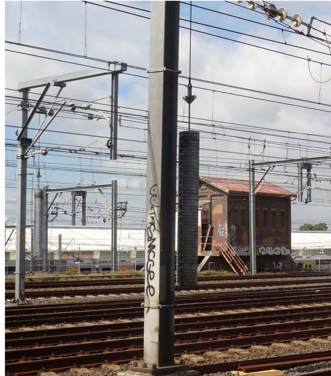
Rail tracks adjacent to the Project area
