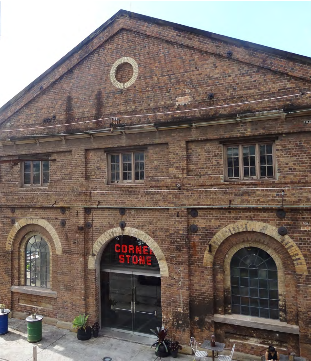
Cover: Historic train carriage at the Australian Technology Park This Page: The Carriageworks, Eveleigh
