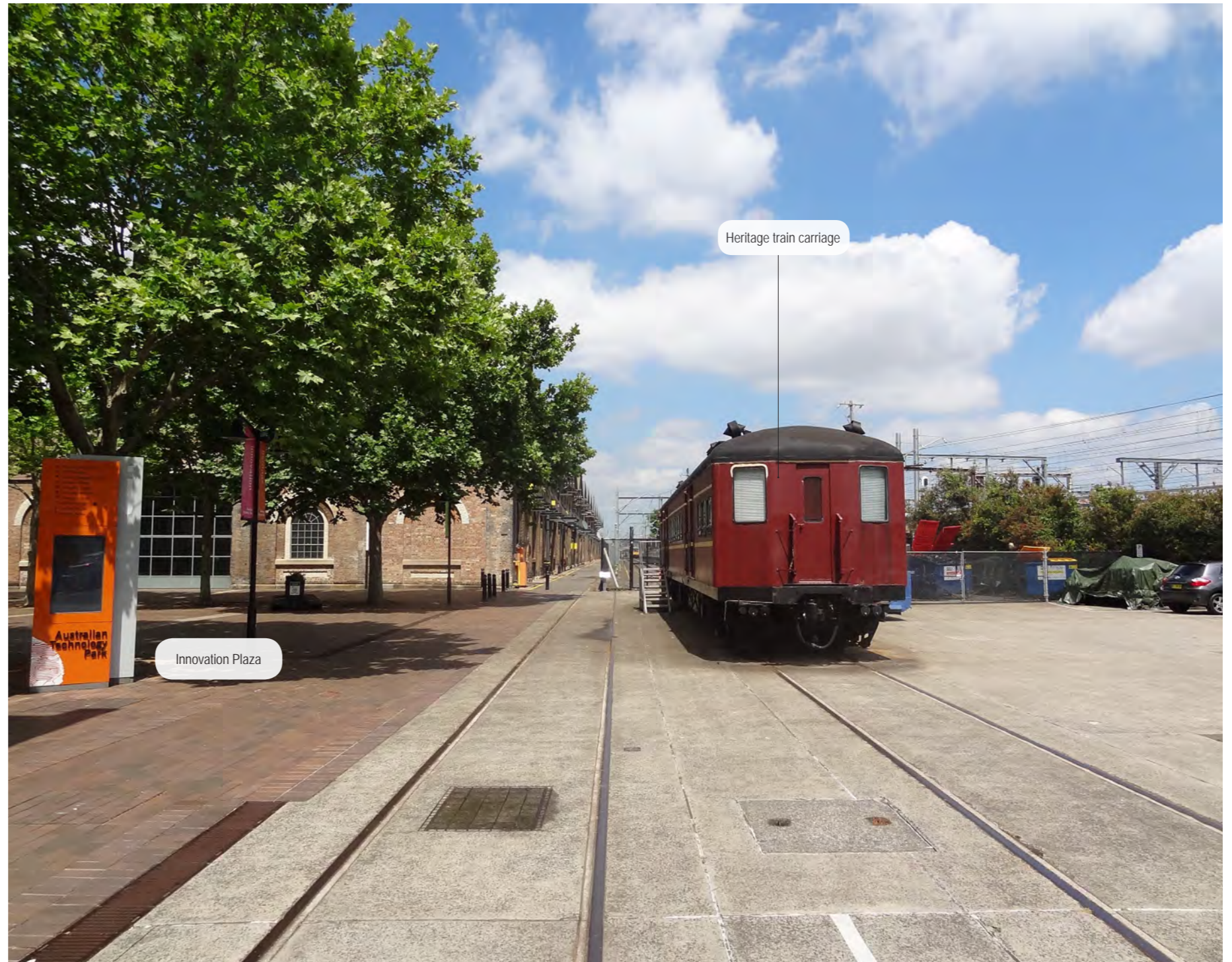
Viewpoint 5: Looking west to proposed extension of Eastern Siding, with the (Former) Locomotive Workshops at left and 'Red Rattler' heritage carriage in the centre of the view
