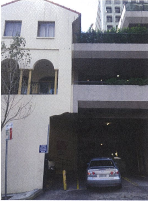
Figure 3-E Protective Screen location to 65 Berry Street, North Sydney – Ground & First Floor and Handrail to Level 2 along south boundary
