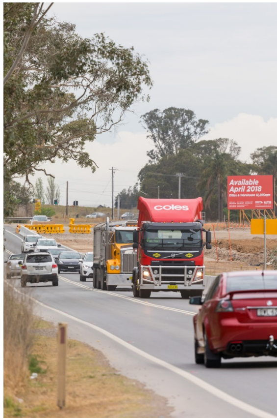
Development along Mamre Road
