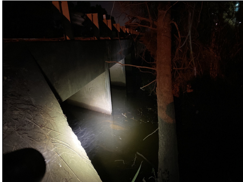
Photo 11. Potential microbat roosting habitat within culverts spanning a non-perennial stream north of the intersection of Mamre Road and Erskine Park Road
