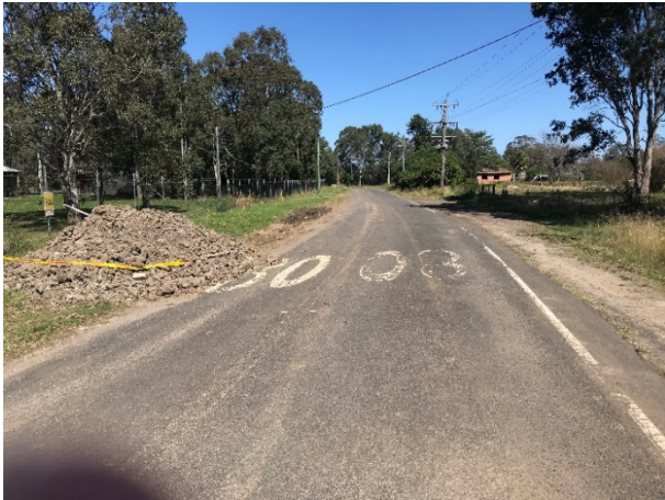
Figure 3-30 Former Luddenham Road alignment, facing south towards current alignment
