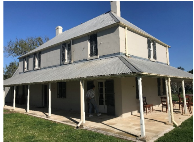
Figure 3-10 Rear and side Mamre House
