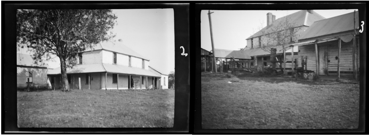
Figure 5-9 'Mamre' in 1930s including some of the infill rooms to the verandah, since demolished. Source: Shaw, E. G. Item 17: 'Mamre', St. Marys, 1933 / Photographer E.G. Shaw, 1933 (Source: State Library of NSW).
