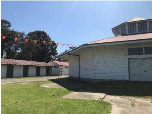
Figure 3-36 View of sheds beside the Rotunda, facing north
