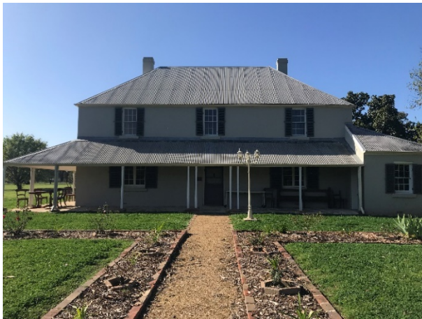
Figure 3-9 Front façade of Mamre House
