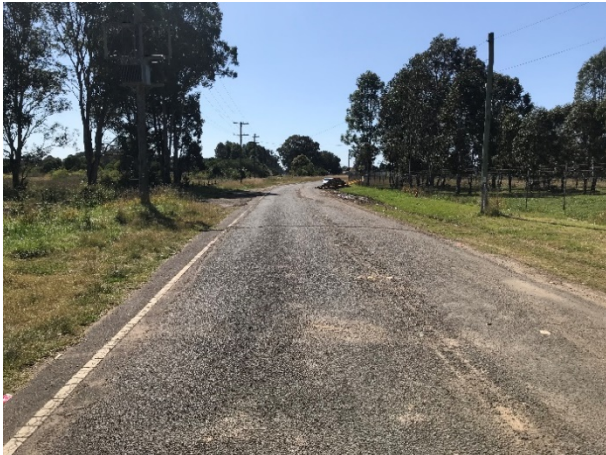
Figure 3-32 Former alignment, looking north
