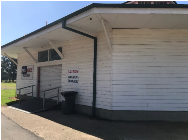
Figure 3-37 Shot of weatherboarding, awning and main entrance door of the Rotunda
