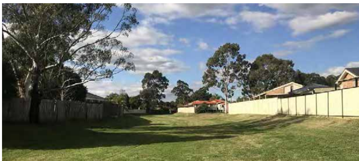
Plate 5-11: View of open grassed drainage channel within the residential zone
