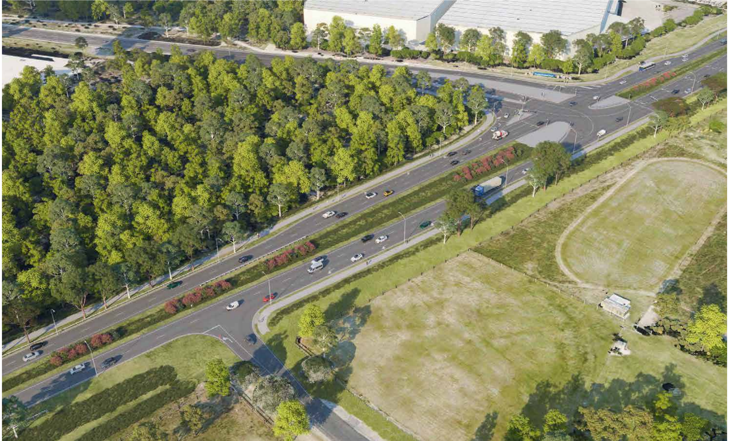
Plate 7-10: Aerial view looking south-east towards the Erskine Business Park
