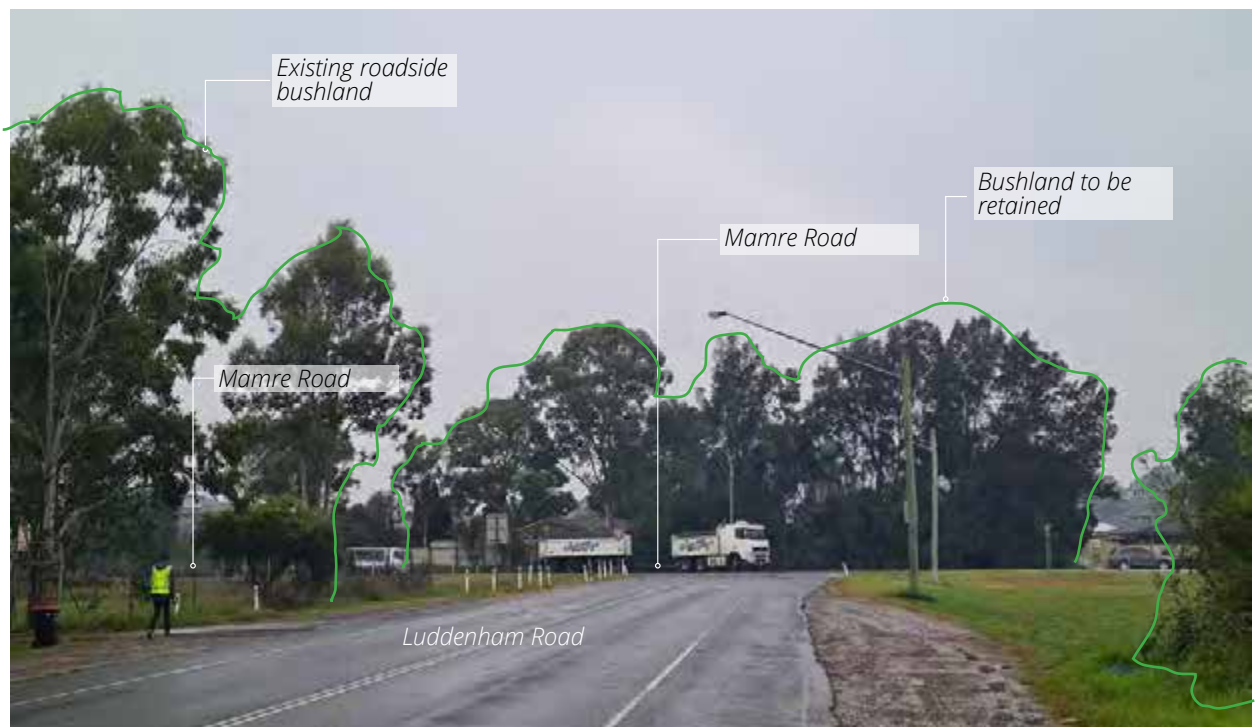
Figure 7-19: Viewpoint 6 - existing view looking east towards the main alignment
