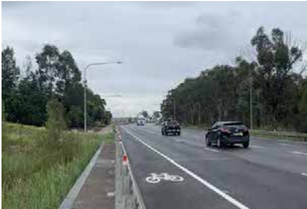
Plate 2-19: Erskine Park Road on approach to the project
