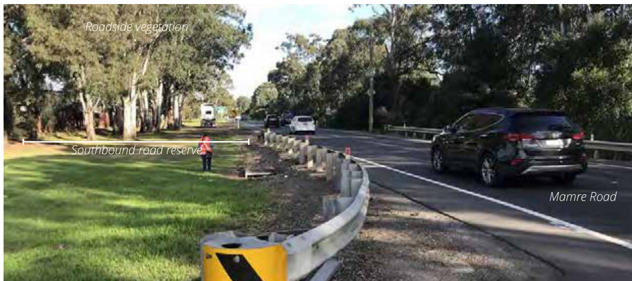
Plate 5-16: Looking south along Mamre Road from close to McIntyre Avenue
