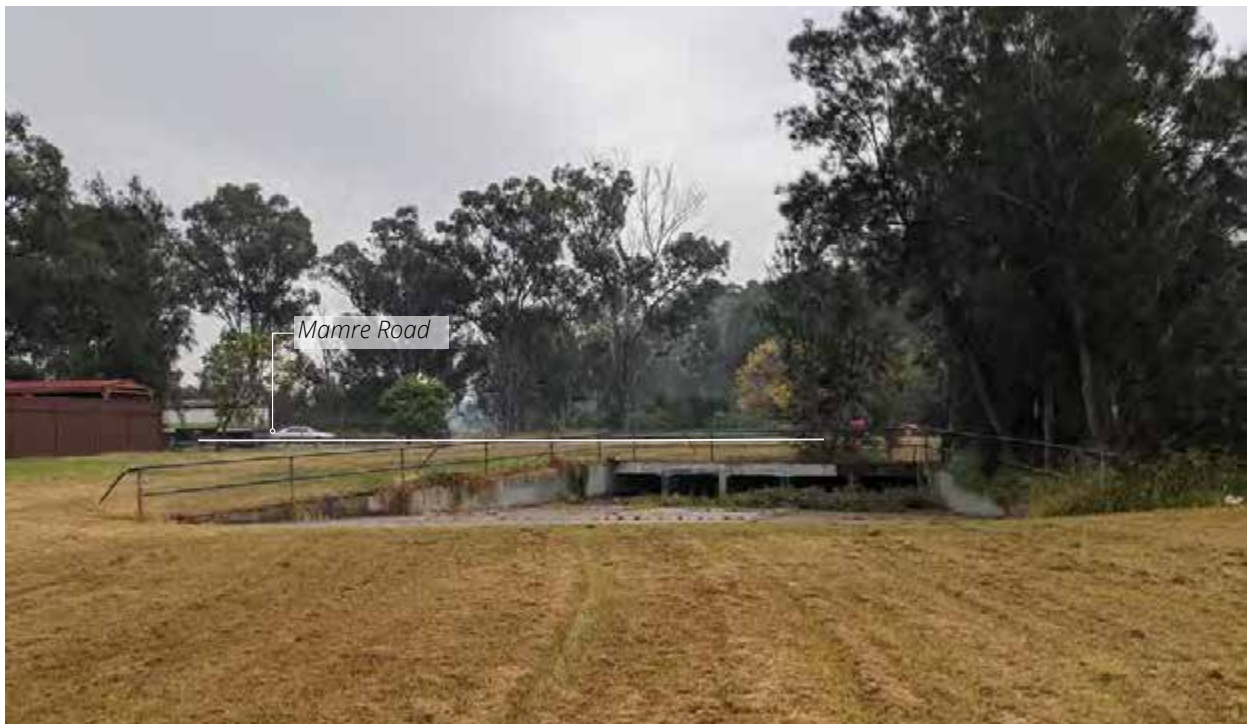
Figure 7-13: Viewpoint 4 - existing view looking west towards the upgrade from drainage channel (62 m from Mamre Road)
