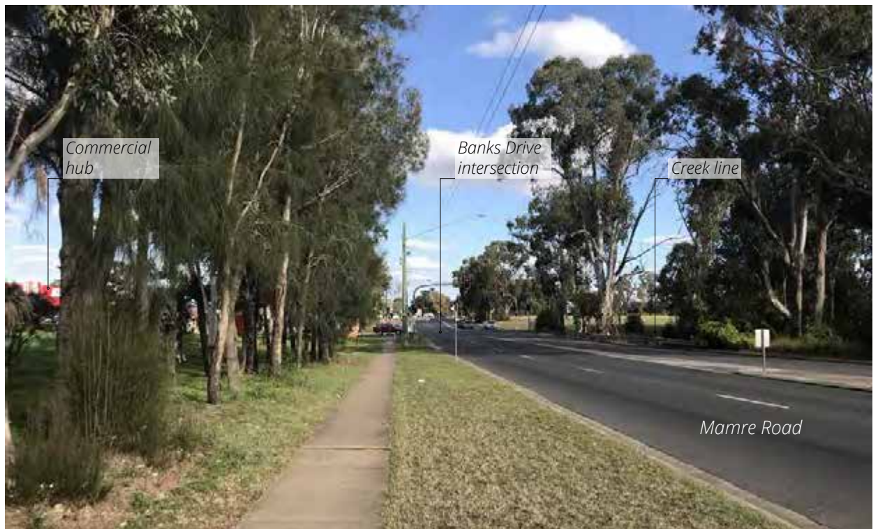
Plate 7-1: Looking south towards the Banks Drive intersection from the southbound setback
