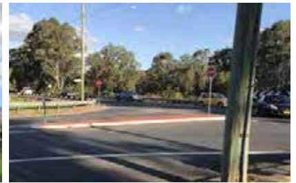
Plate 5-3: Existing road corridor
