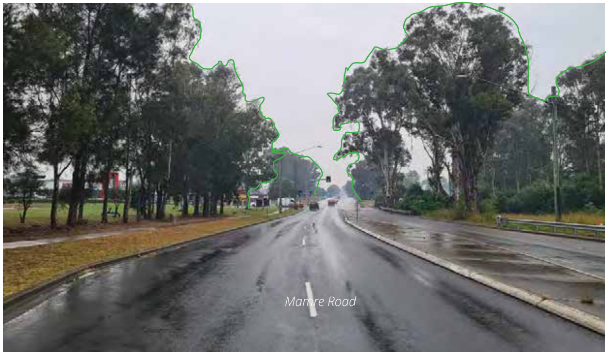
Figure 7-4: Viewpoint 1 - existing view looking south in the southbound travel lane
