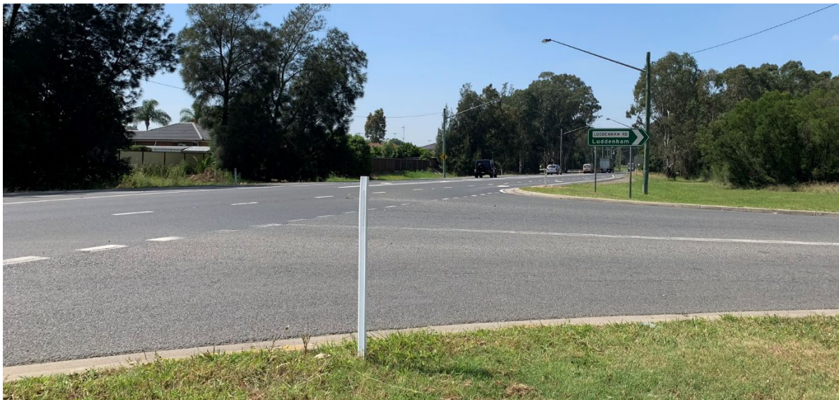
Figure 2-4: Photo of existing intersection of Mamre Road and Luddenham Road
