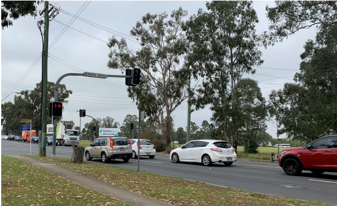
Figure 2-2: Photo of existing intersection of Mamre Road and Banks Drive looking south
