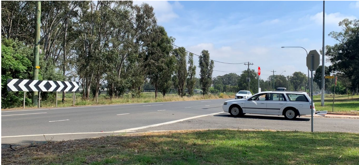
Figure 2-3: Photo of existing intersection of Mamre Road and Solander Drive
