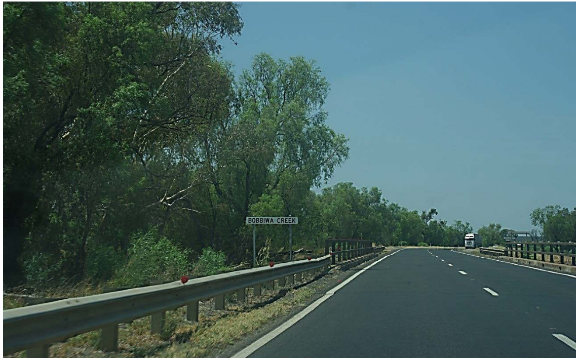
Figure 55 – Looking south from CH 2450.000 across Bobbiwaa Creek Bridge. The proposed works would potentially require removal of existing screening trees along eastern verge along left side of highway beyond the bridge.
