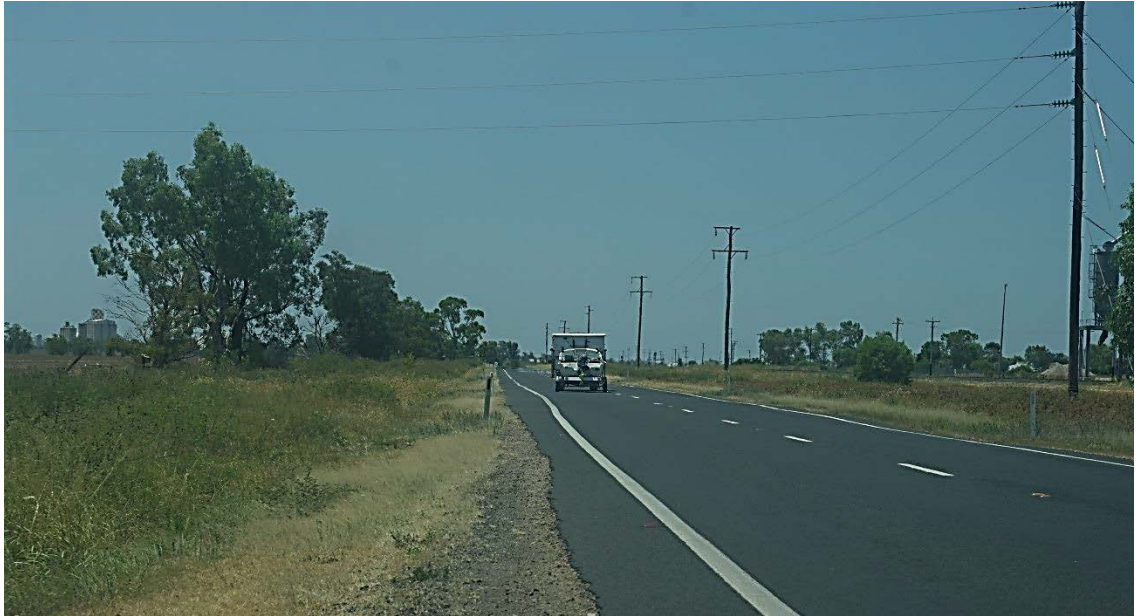
Figure 71 – Looking north from CH 4000.00. Proposed highway alignment deviates to the western verge from this point northwards, requiring removal of trees to the left side of image.
