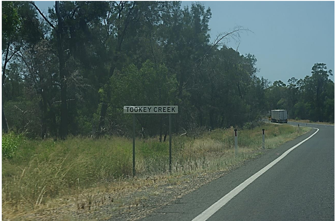
Figure 66 – Looking north from CH 200.000 at Tookey Creek culvert. Proposed highway alignment departs from existing and continues straight through existing vegetation at centre of image, requiring the removal of all trees along the western margin of the existing highway.
