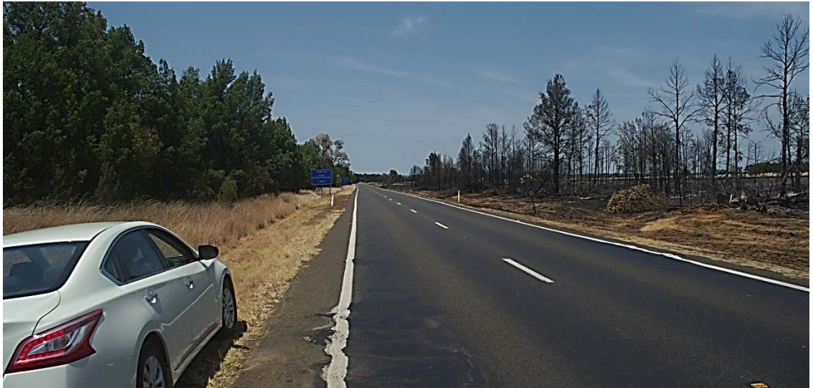
Figure 48 – Looking south from Private Access entry at N2MS1 – CH 2180.000. Broad scale agricultural land use both sides of the corridor. Proposed highway upgrade runs diagonally from left to the right of the existing carriageways through the trees and grass verge on the left of image.
