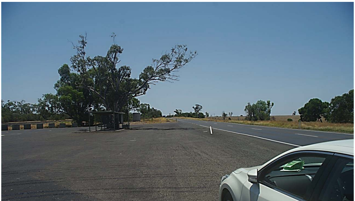
Figure 64 – Looking north from CH 2250.000 at Woolabrar Rest Area. Proposed highway embankments widened to accommodate swales along both verges, potentially requiring the removal of the trees along the eastern side to the right of image.
