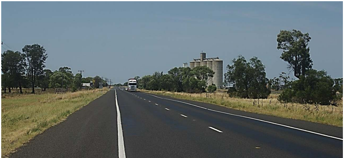
Figure 58 – Looking south from CH 10400.000. Proposed highway embankments potentially widened, requiring the removal of the trees along the western margins to the centre right of image.
