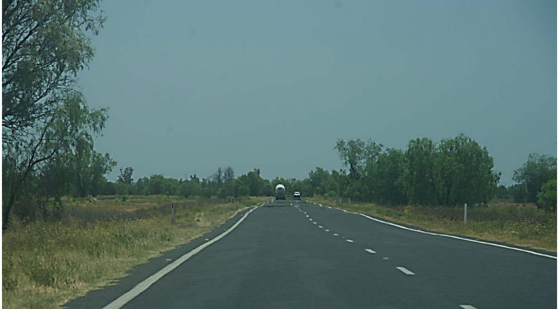
Figure 54 – Looking north from CH 800.000. Proposed carriageways situated to the right of existing potentially requiring the removal of the trees to right of image.
