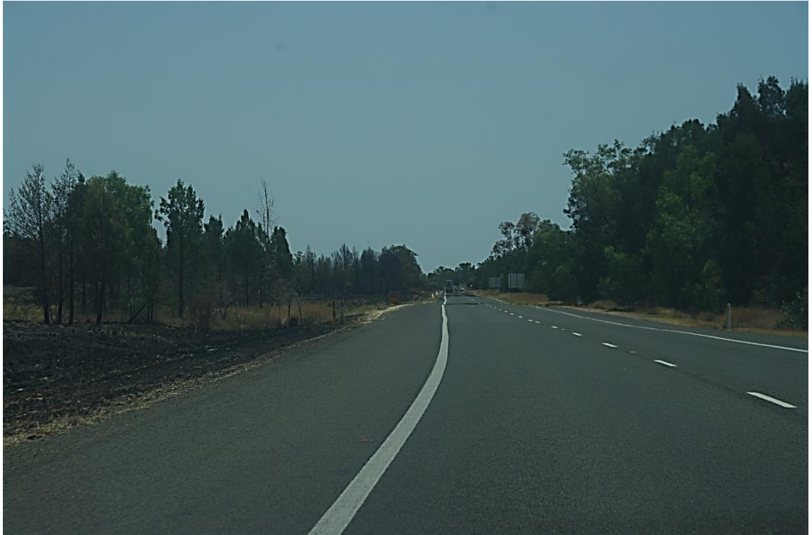
Figure 28 – Enclosed Vegetated Highway Corridor Landscape Character. N2MS1 – Looking north from CH1380.000.
