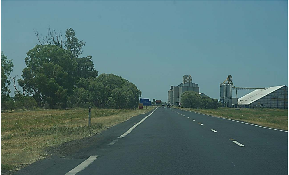
Figure 72 – Looking north from CH 6400.00. Proposed highway alignment deviates to the eastern verge from this point northwards, requiring removal of trees screening structures to the right side of image.
