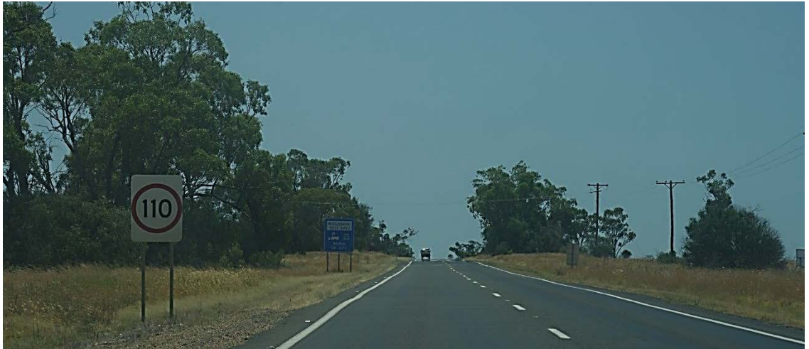
Figure 62 – Looking north from CH 1650.000. Proposed highway embankments widened to accommodate swales along both verges, potentially requiring the removal of the trees along both margins, particularly on the eastern side to the right of image.
