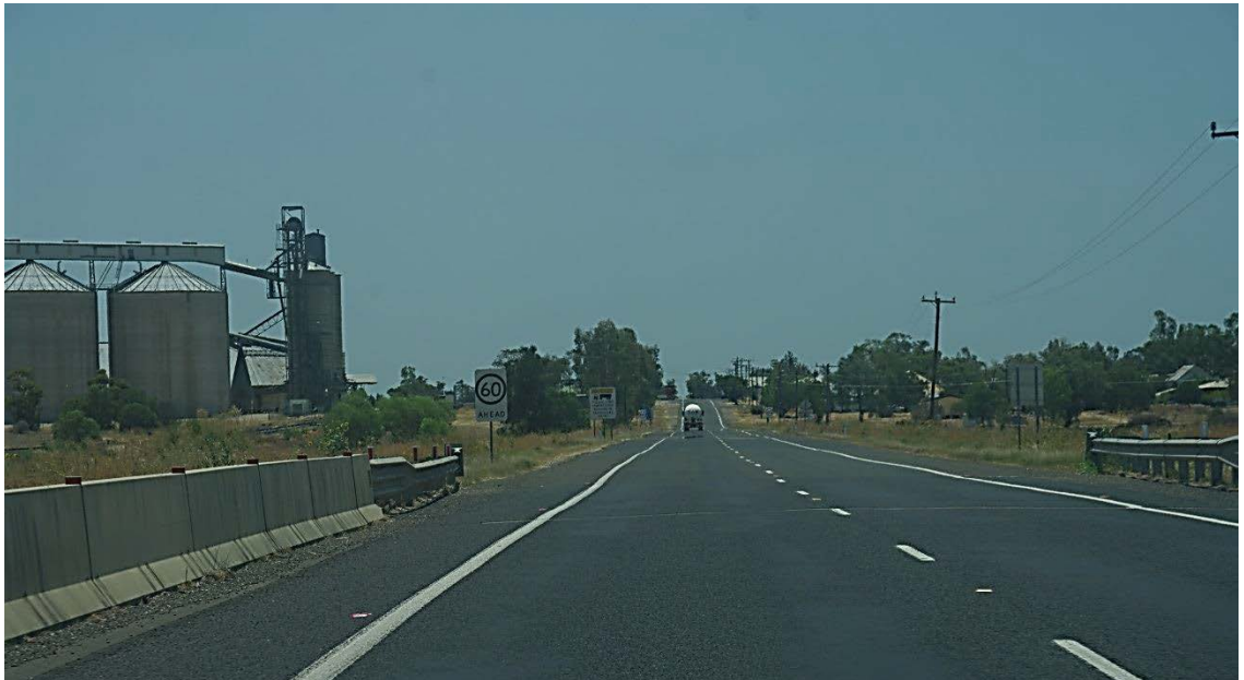
Figure 60 – Looking north from CH 0000.000. Proposed highway widens to accommodate right turning lane, requiring the removal of the avenue trees along the western margins to the centre left of image.
