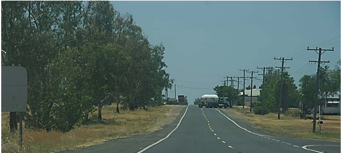
Figure 61 – Looking north from CH 300.000. Proposed highway widened to accommodate right turning lane, requiring the removal of the avenue trees along the western margins to the left of image.
