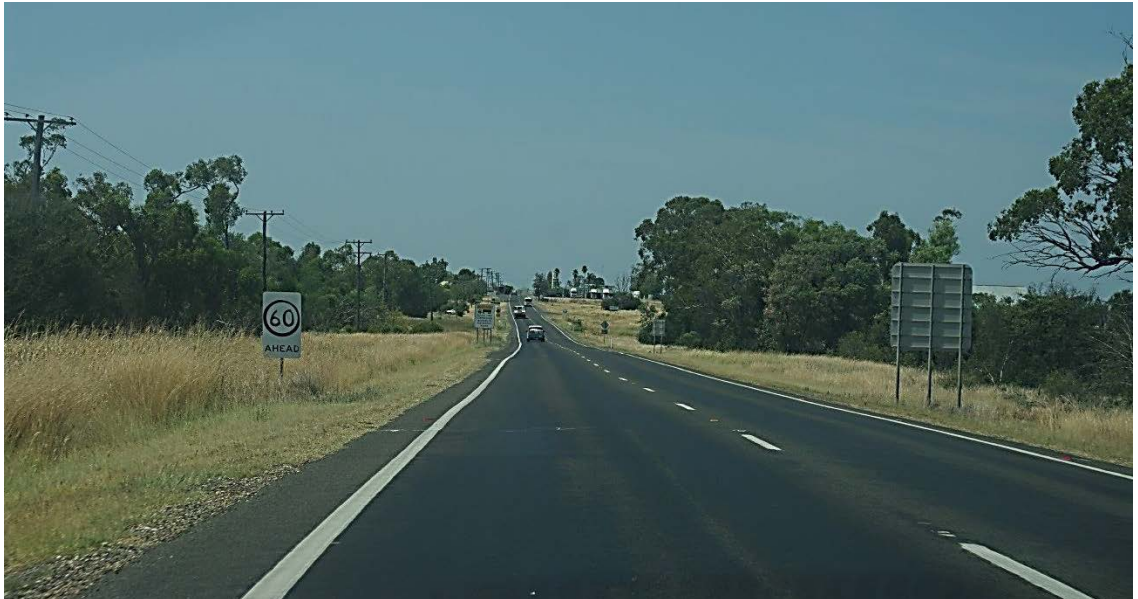
Figure 63 – Looking south from CH 1750.000. Proposed highway embankments widened to accommodate swales along both verges, potentially requiring the removal of the trees on the western side to the right of image.
