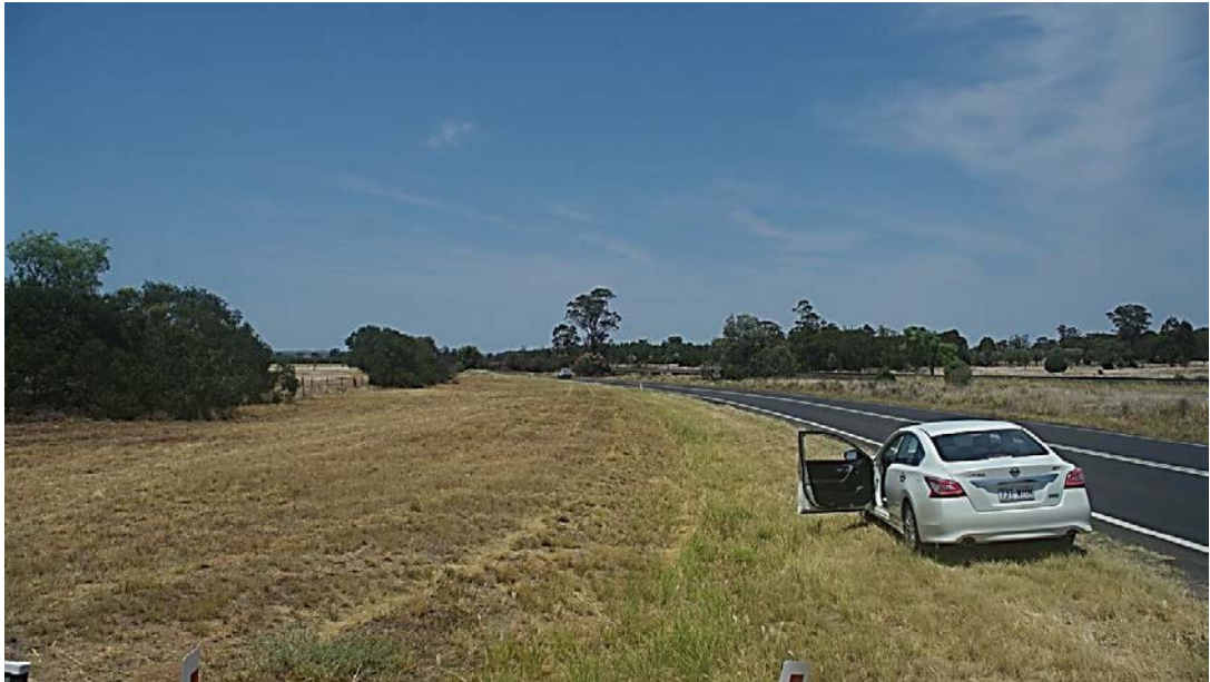
Figure 49 – Looking south from Private Access entry at N2MS1 – CH 2980.000. Broad scale agricultural land use both sides of the corridor. Proposed highway upgrade runs to the left of the existing carriageways through to the centre of the image.
