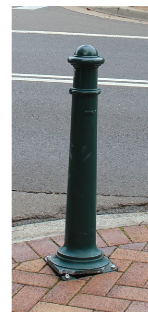
Figure 3-53 Federation style powder coated removable bollard to match existing.
