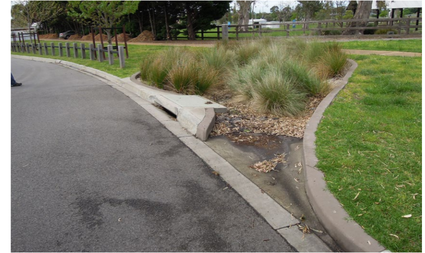
Figure 6-47 Example of a bioretention basin in a streetscape verge, Melbourne, Victoria
