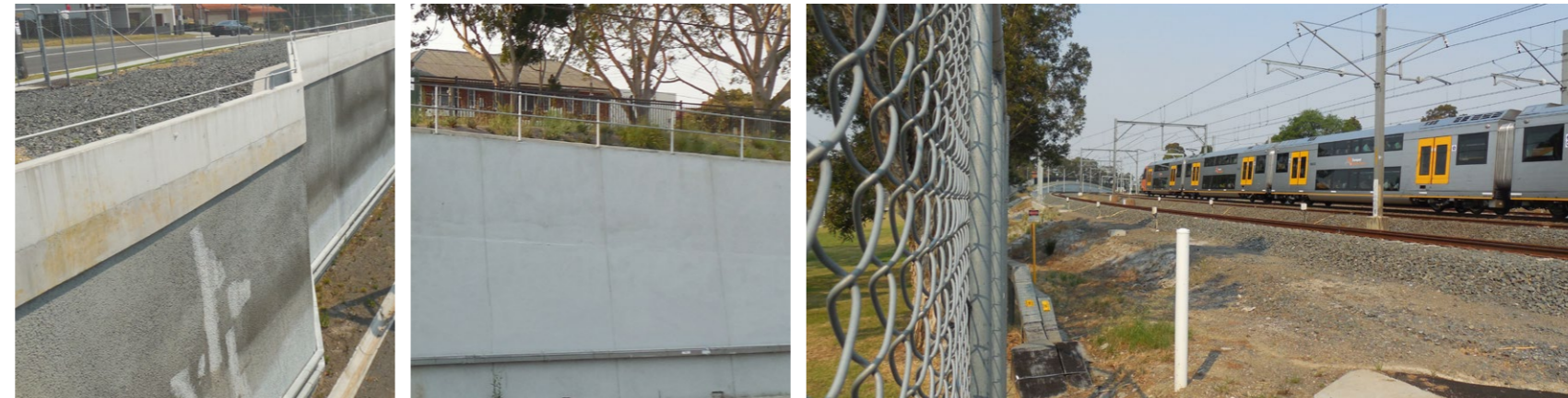
Shotcrete smooth finish
