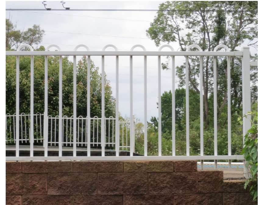
Figure 6-19 Existing Looped Palisade Fencing at Station Precincts
