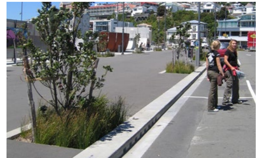
Figure 6-49 Example of a tree pit (small bioretention system) collecting water (via kerb inlet piping) from a carpark in New Zealand
