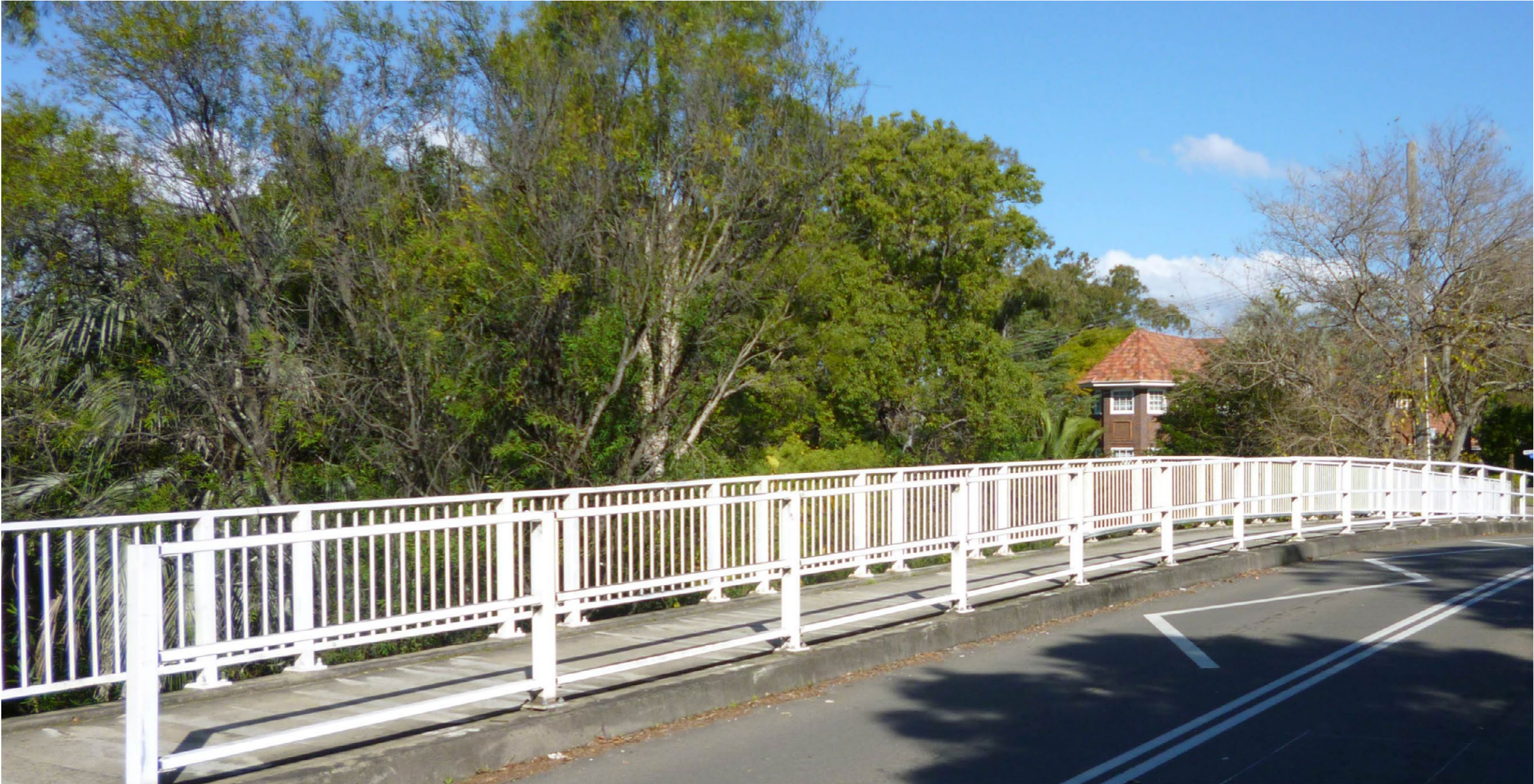
Figure 3-18 Pre-construction works view - looking south-west along Cheltenham Road
