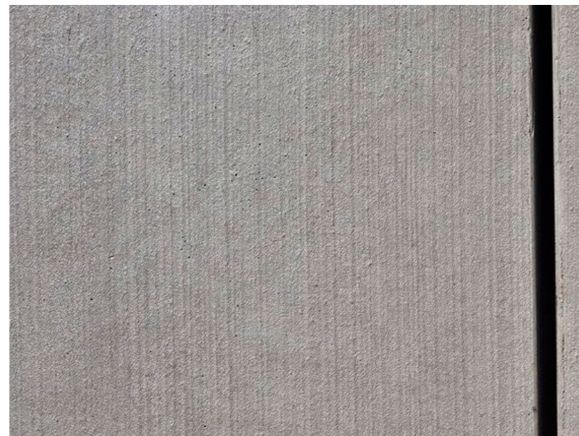
Figure 3-24 Broom finish concrete pedestrian pavement
