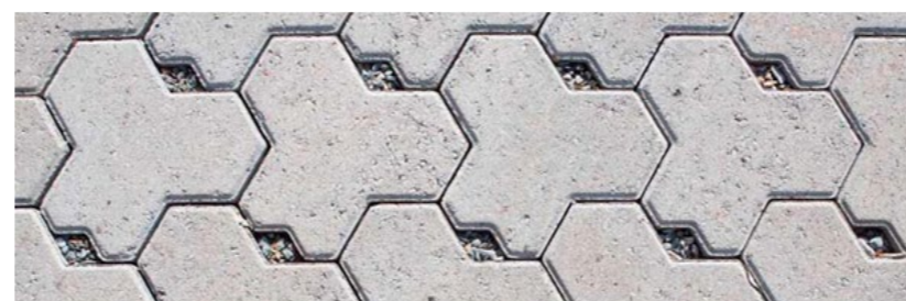
Figure 3-27 Permeable paving carpark ✓
