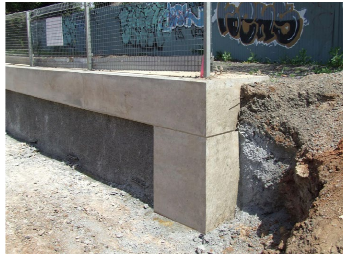
Figure 6-9 Example of Termination Wall
