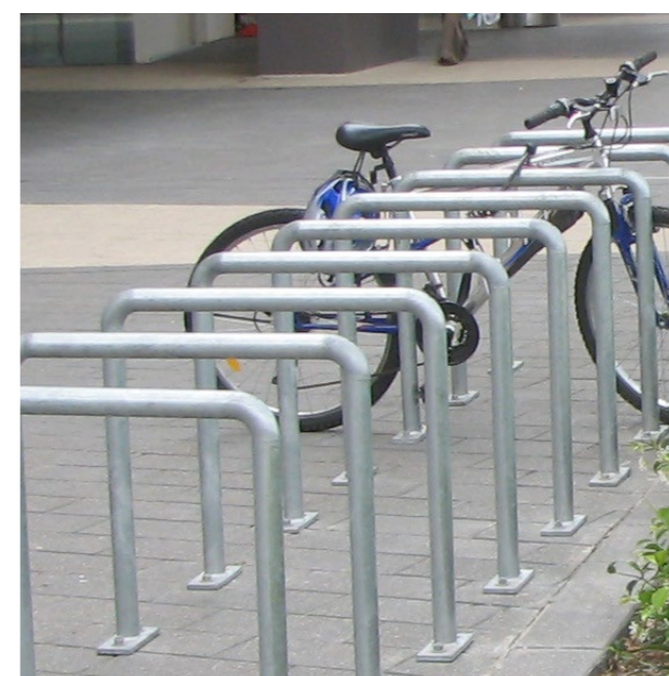
Figure 3-52 Galvanised Steel arc bike racks
