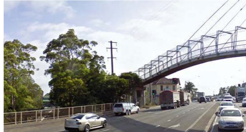
Figure 6-40 Existing Pennant Hills Road, Pennant Hills
