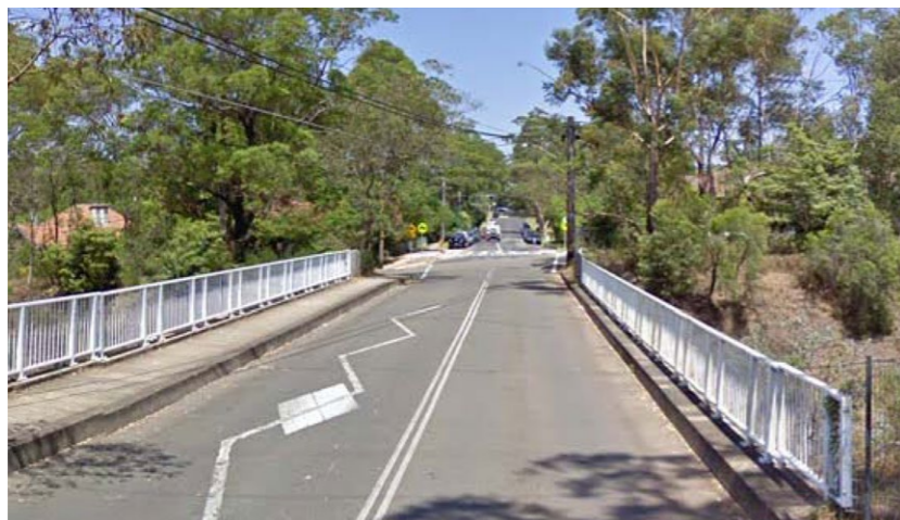
Figure 6-39 Existing Chapman Avenue bridge, Beecroft
