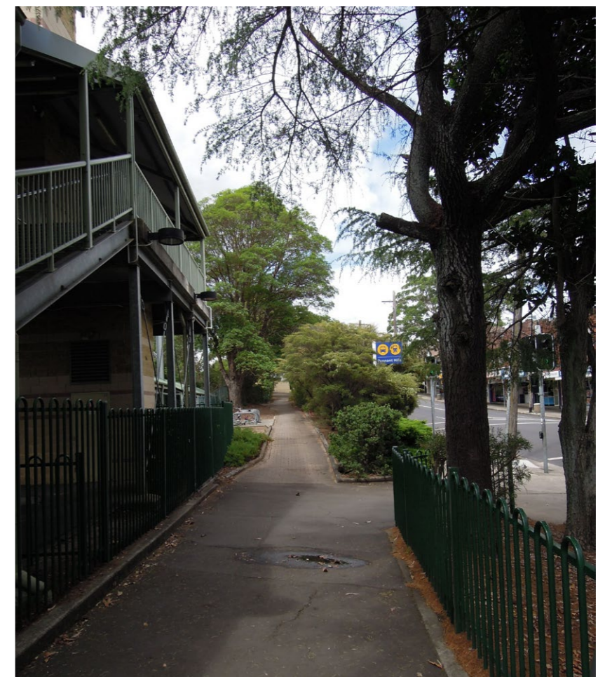
Figure 3-57 Existing western station entrance, verge landscape with formal pedestrian path and precinct fencing
