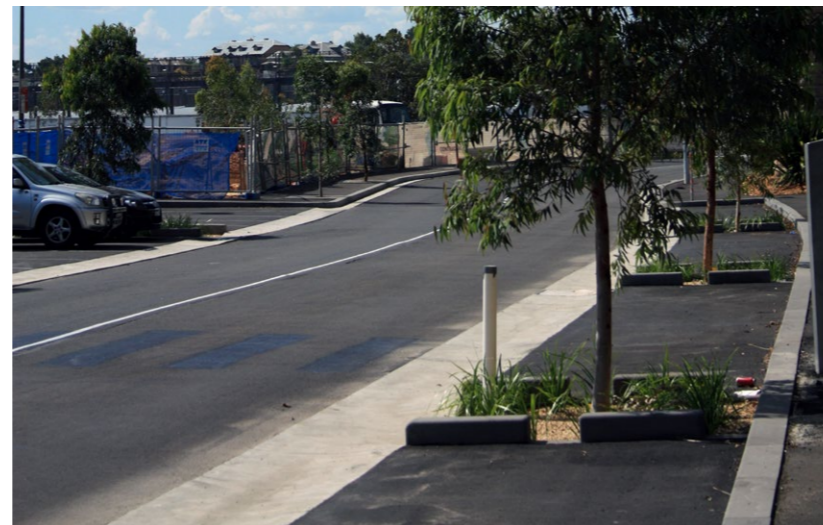
Figure 6-48 Example of a tree pit (small bioretention system) separating carparking spaces in a streetscape at Pyrmont, NSW
