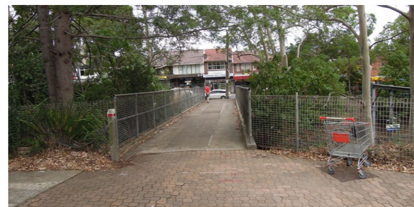
Figure 3-55 Existing pedestrian bridge linking village to bus interchange
