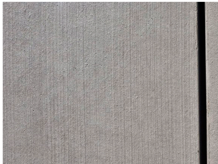
Figure 3-47 Broom finish concrete paths to high pedestrian areas
