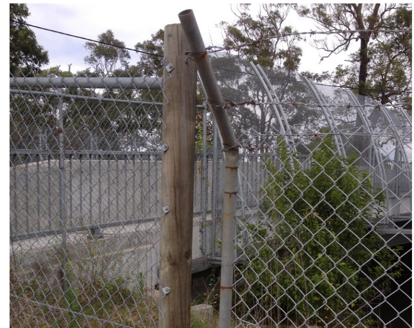
Figure 6-20 Existing Perimeter Fencing Junctions
