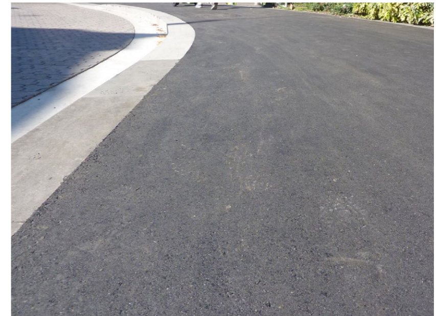
Figure 3-25 Asphalt pedestrian pavement with concrete edge
