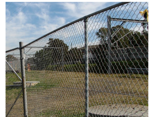
Figure 6-23 Type 1 Perimeter / Security Fencing
