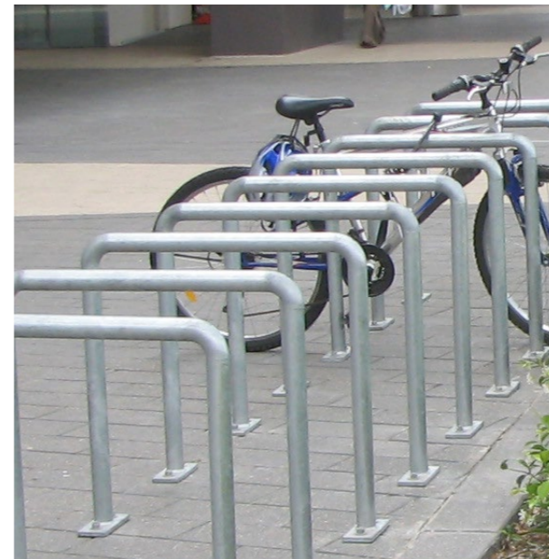
Figure 3-68 Galvanised Steel arc bike racks
