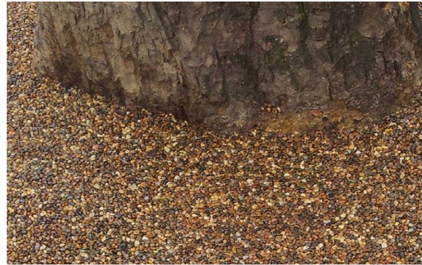
Figure 3-63 Resin-bound gravel to base of trees in pavement
