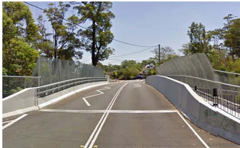
Figure 6-38 Existing Copeland Road Bridge, Beecroft
