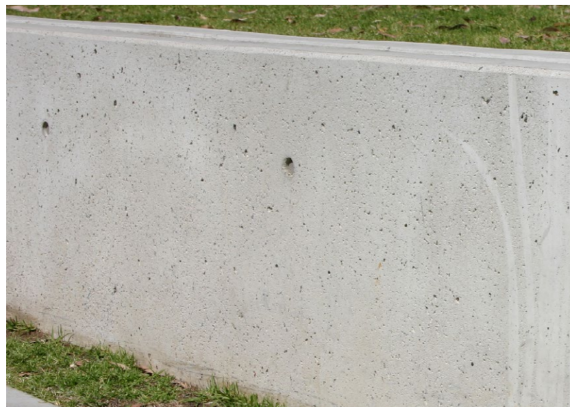
Figure 3-26 Class 2 concrete retaining walls within station precinct
