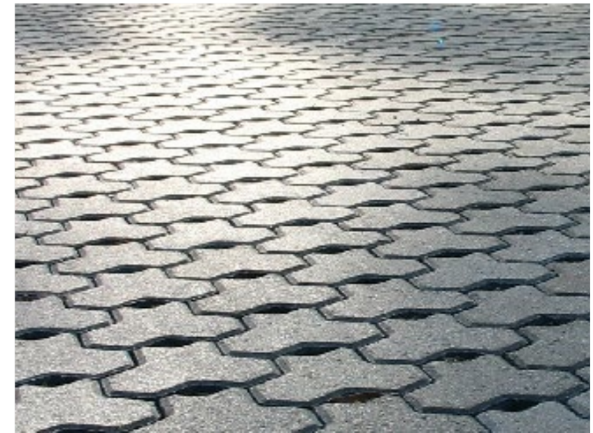
Figure 3-48 Permeable paving to carpark to encourage passive irrigation of tree planting and support root growth through structural soils below.
