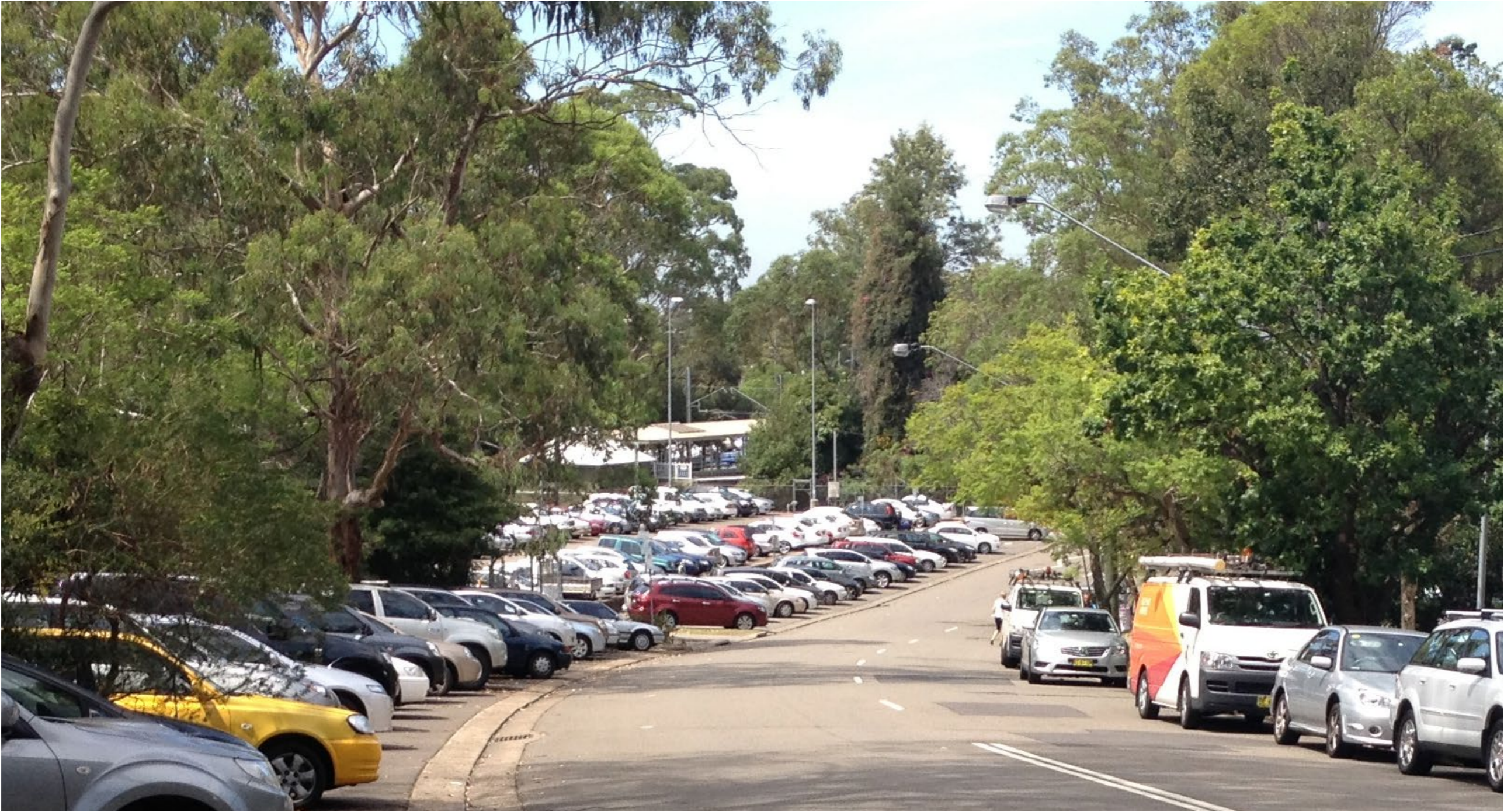
Figure 3-44 Pre-construction works view - looking south along Wongala Crescent towards Beecroft Station
