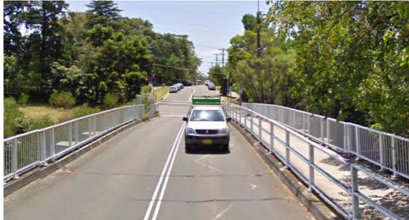
Figure 6-37 Existing Cheltenham Road Bridge, Cheltenham
