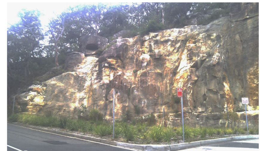
Figure 6-4 Example of rock cutting shotcrete colour matching
