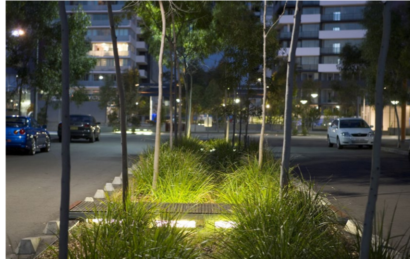
Figure 6-46 Example of a bioretention basin situated in a street median at Victoria Park, NSW
