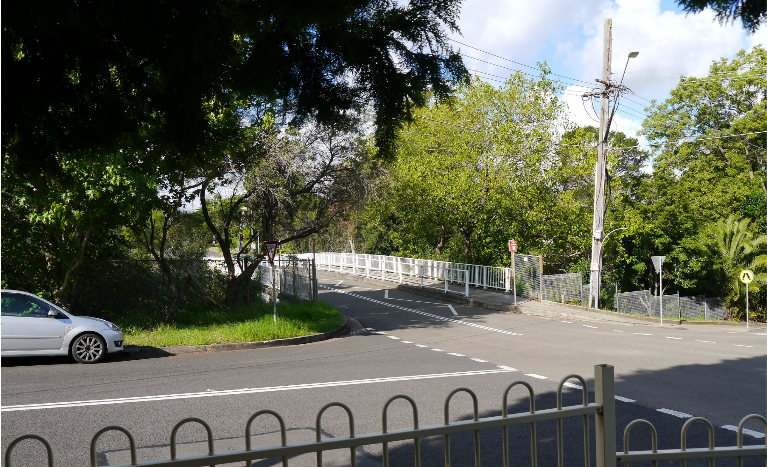
Figure 3-16 Pre-construction works view - looking east from the corner of The Crescent and Cheltenham Road road towards the station
