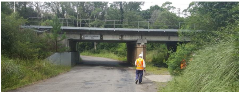
Figure 7 Downstream face of the Chittaway Creek crossing
