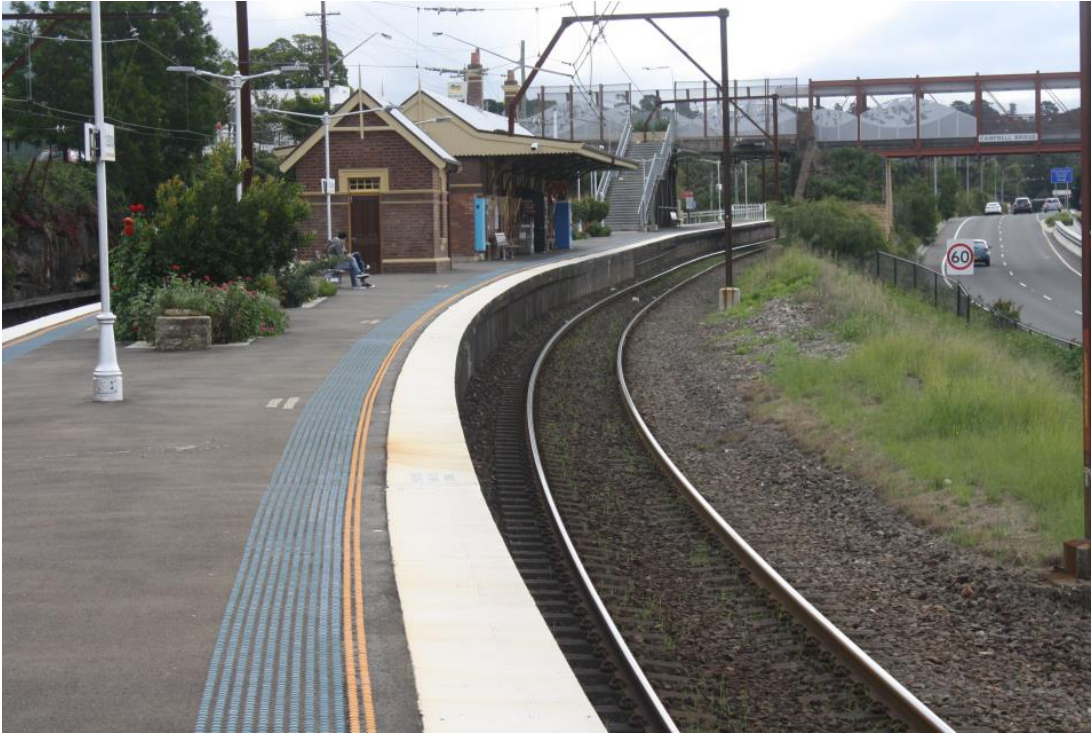
Figure 10 View looking south-east of the 1902 platform 1 at Hazelbrook Station
