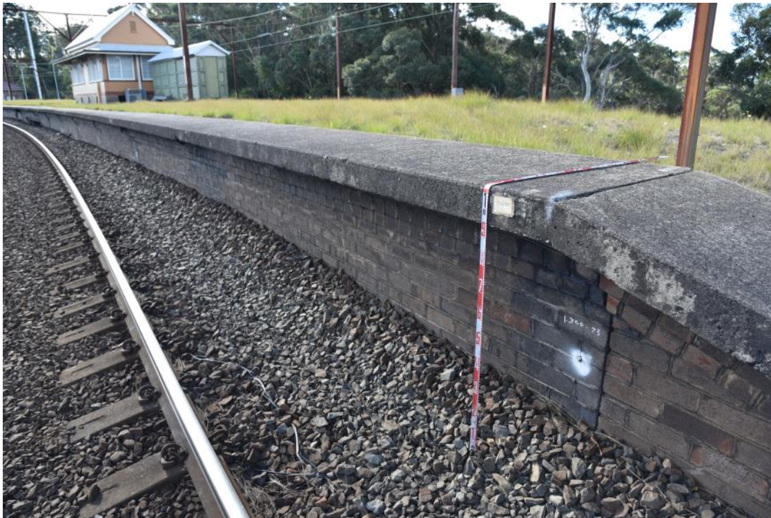
Figure 22 View north west of Newnes Junction island platform (platform 1)
