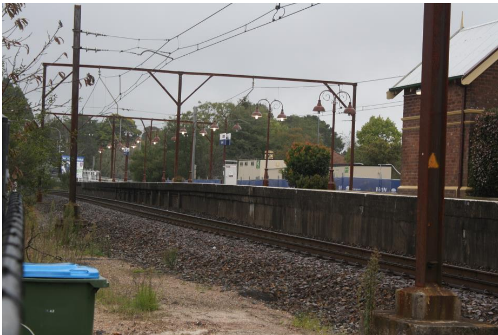
Figure 19 View looking north west of a section of platform 2 at Leura Station
