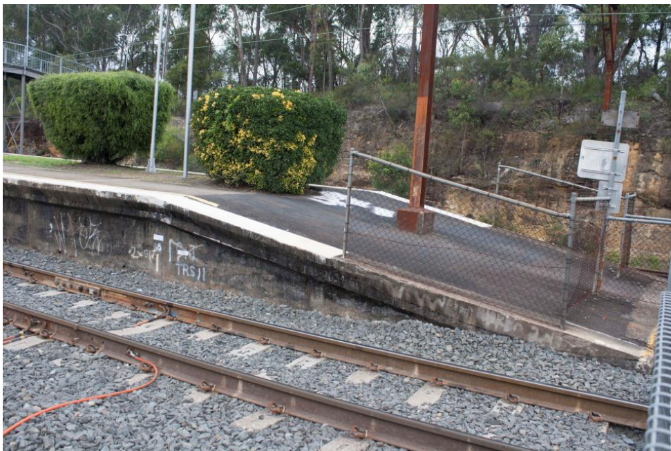
Figure 6 View looking east of a section of Linden Station platform 1
