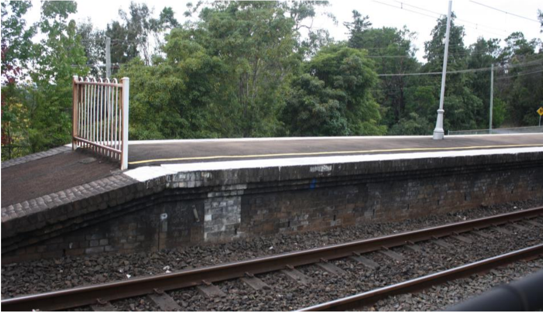
Figure 3 View looking east of the 1940s platform extension at Faulconbridge Station
