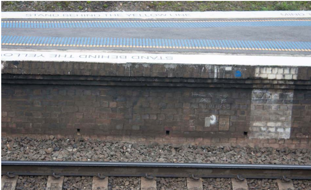
Figure 15 A section of 1902 platform coping at Wentworth Falls Station
