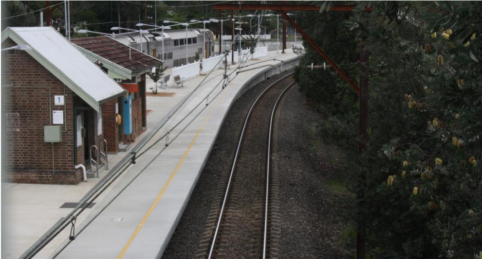
Figure 13 View looking south-west of a section of platform 1 at Bullaburra Station
