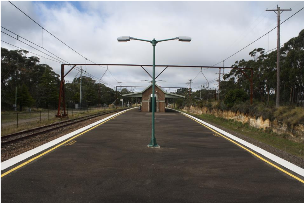
Figure 21 View looking north of a 1911 section of platforms 1 and 2 at Bell Station
