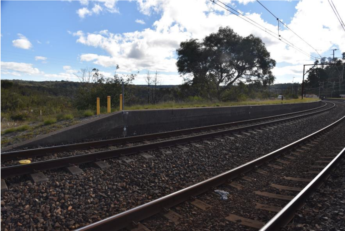
Figure 23 View south west of Newnes Junction siding platform (platform 2)
