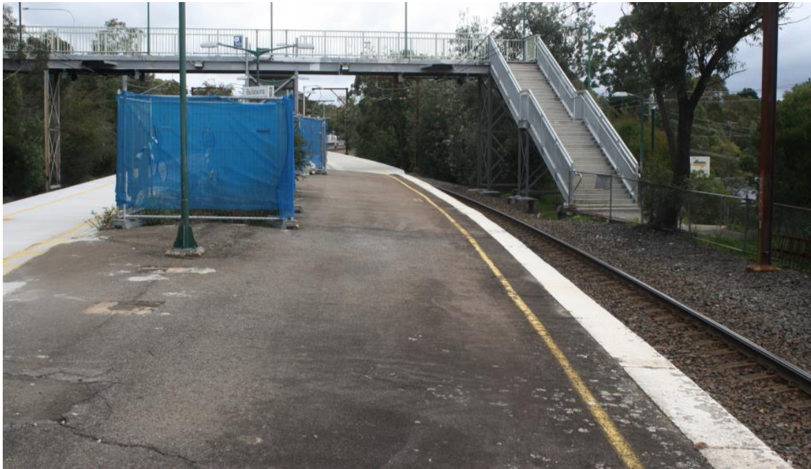
Figure 12 View looking south-west of a section of 1924 platform of Bullaburra Station
