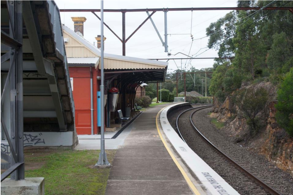
Figure 4 View looking east of Linden Station platform
