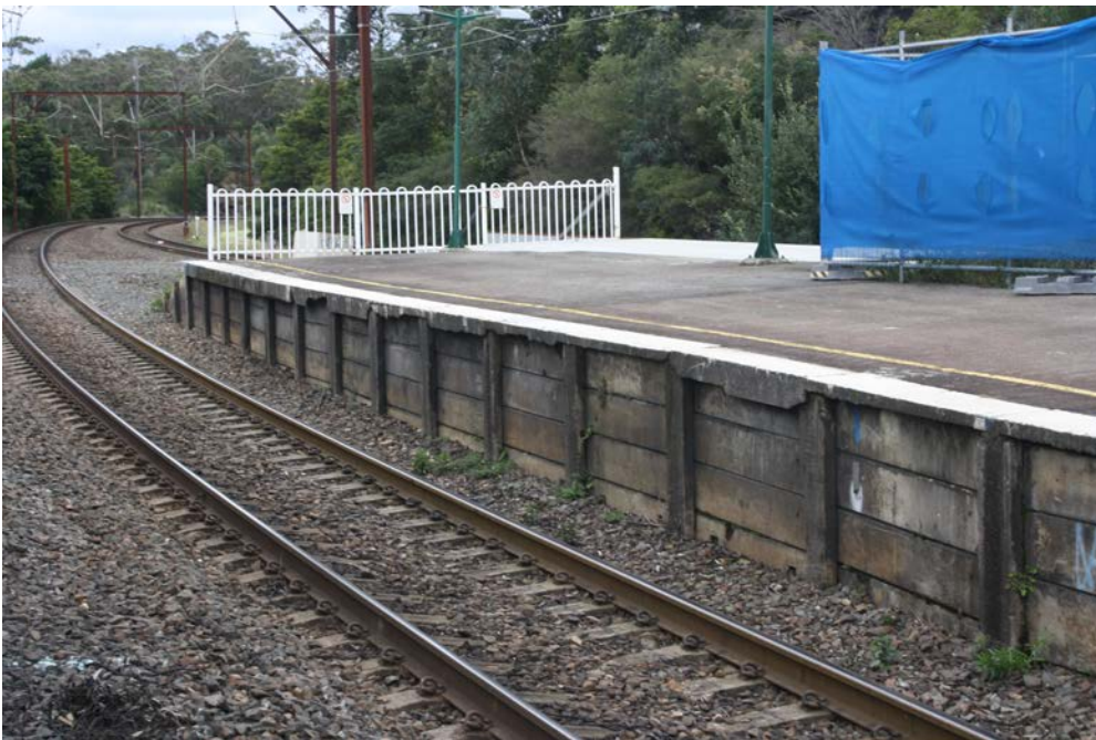
Figure 14 View looking south-west of a section of platform 2 at Bullaburra Station
