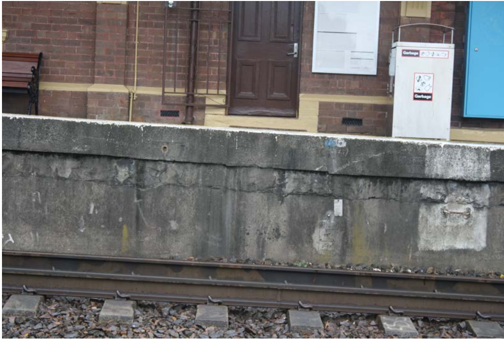
Figure 18 View looking north of a section of platform 2 at Leura Station
