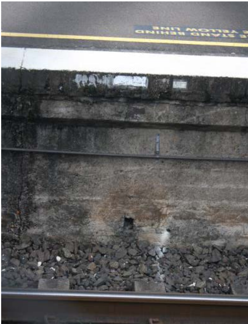
Figure 2 A section of the 1902 platform coping at Faulconbridge Station
