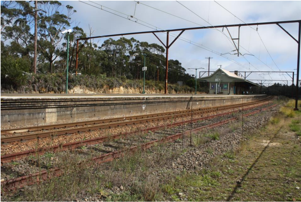
Figure 20 View looking west of a 1911 section of platform at Bell Station
