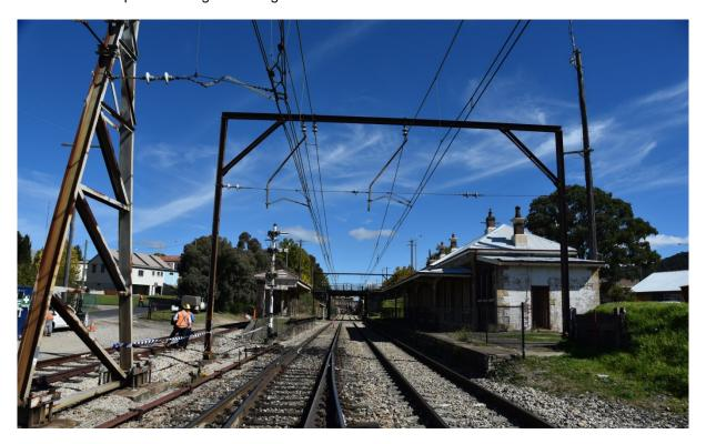
Figure 8: Western main lines near station platforms, showing portal overhead wiring structure and signalling lights. West aspect
