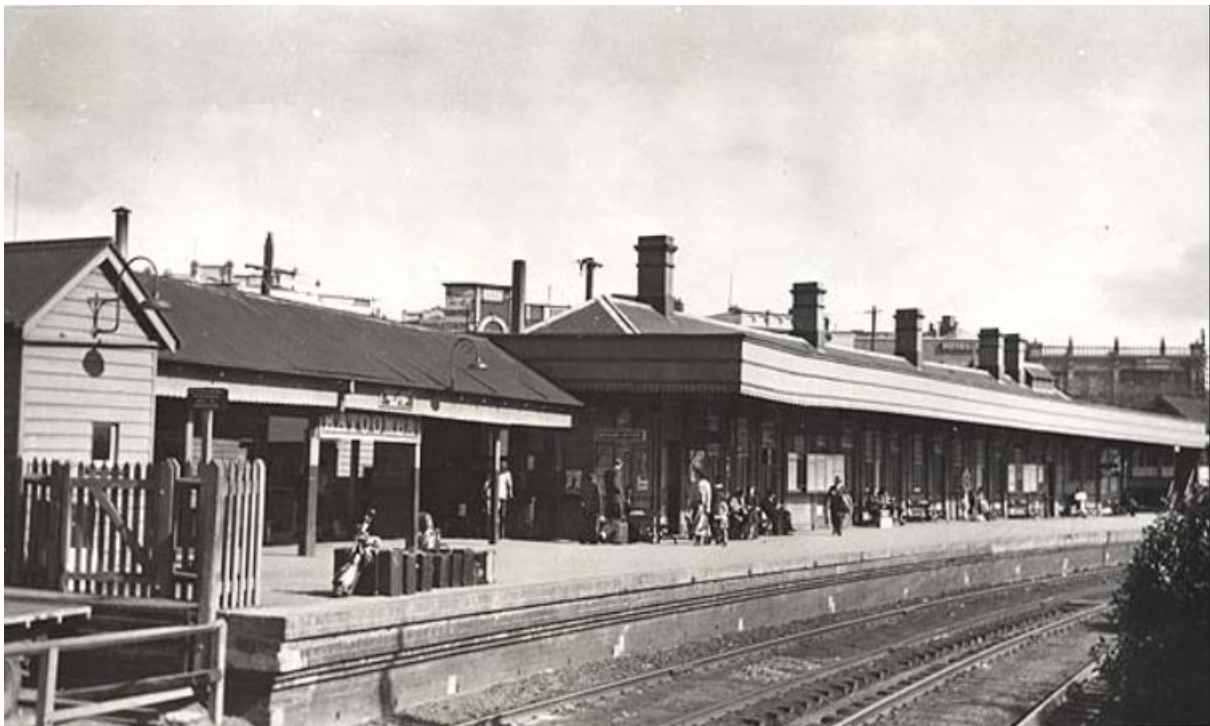
Figure 10 View of Katoomba Railway Station c1947. Note the additional courses of brickwork and the removal of the original bullnose coping. Source: State Archives & Records. Digital ID 17420_a014_a014000744
