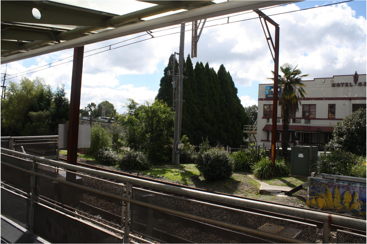
Figure 12 Overview of stanchion SL109+838. View north west
