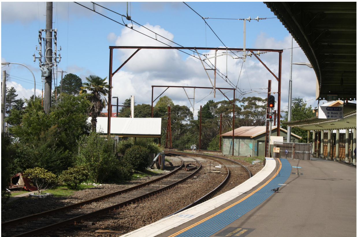
Figure 11 Overview of stanchion SL109+838. View east
