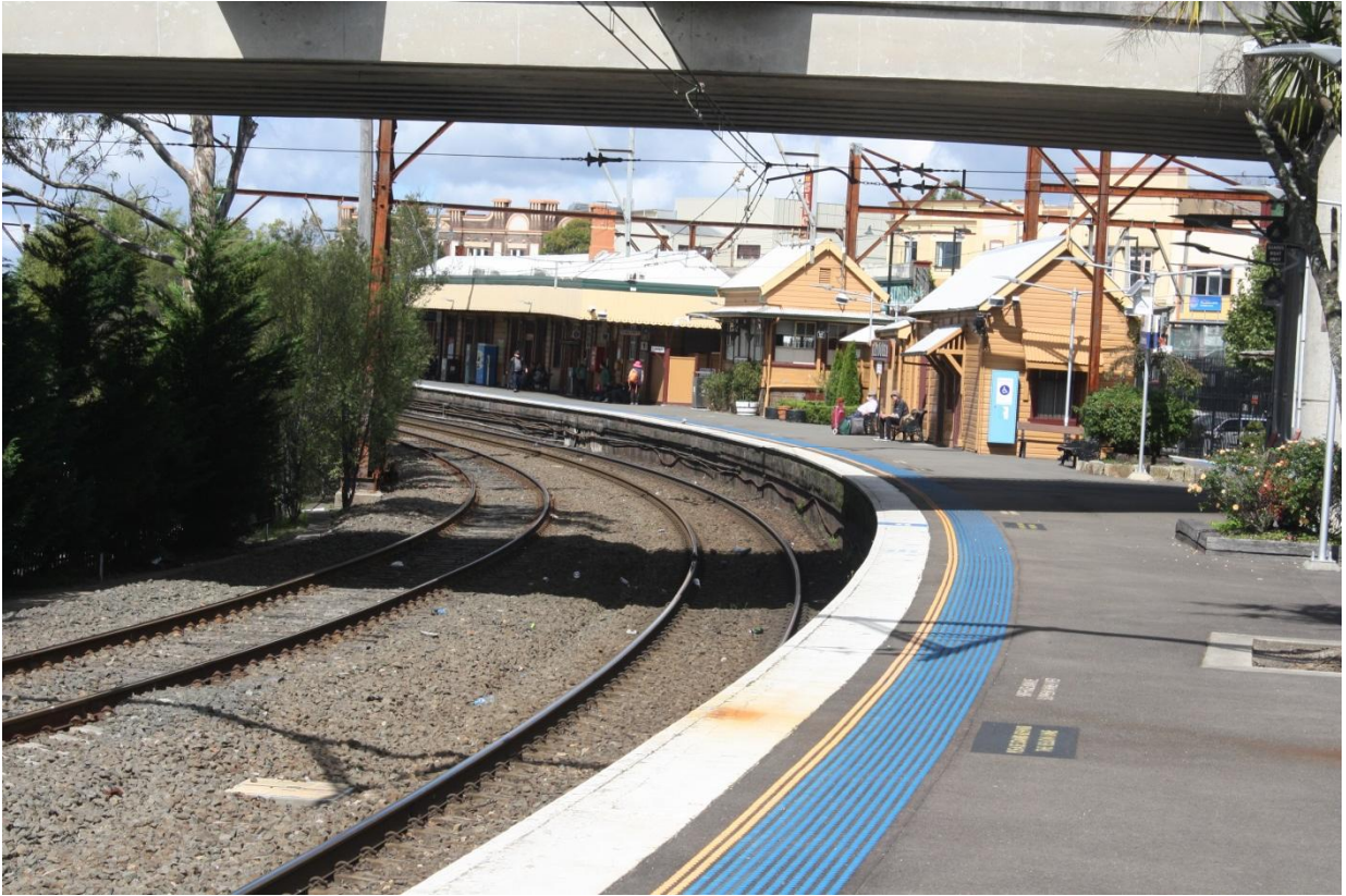
Figure 5 View east along platform 1, showing curvature of platform. Note addition of coping to edge of the platform
