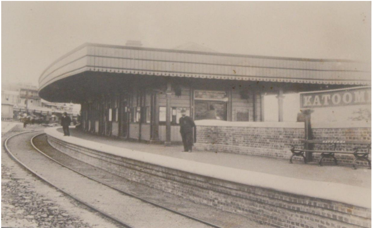
Figure 9 View of Katoomba Railway Station 1891. Note bullnose coping. Source: State Archives & Records. Digital ID 17420_a014_a014000745
