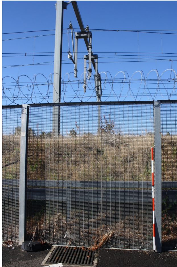
Figure 11: Detailed view of the difference in ground level between where the second Station Master's residence was built and the built up level of the current track level (view to southeast). (Photo scale = 20 cm gradients)
