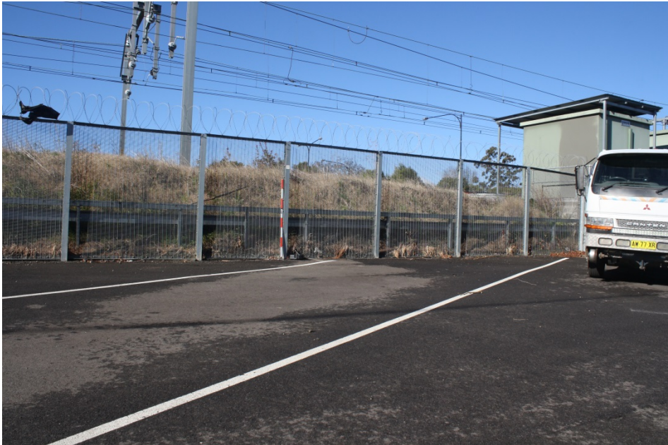
Figure 10: View showing the difference between the ground level between the current track and the former ground level associated with the second Station Master's residence (view to south) (Photo scale = 20 cm gradients)
