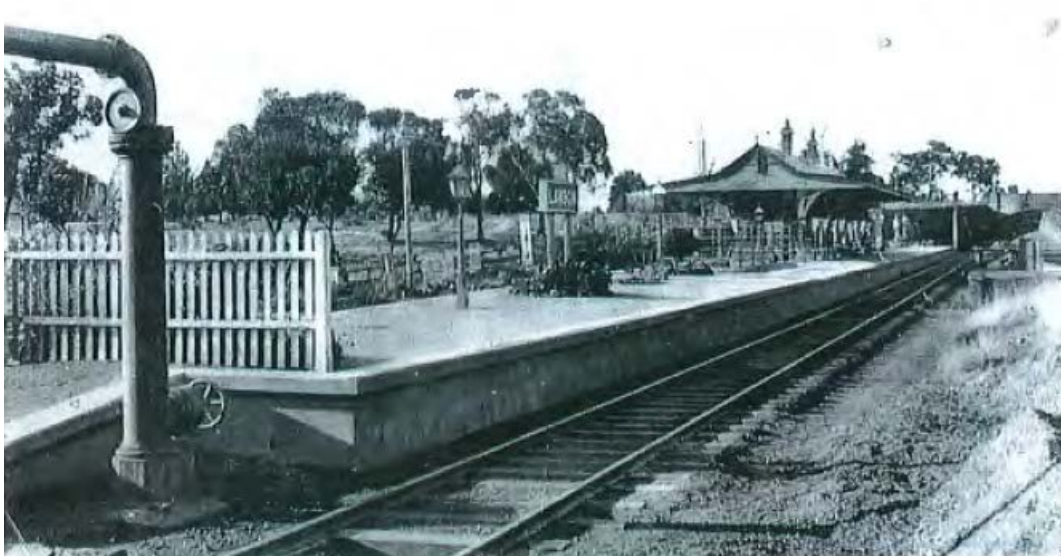
Figure 3 Lawson Station 1908 from the south-west . Note squared edge to coping. Source: ARHS Railway Resource Centre, 0000628 in AMBS 2013:22
