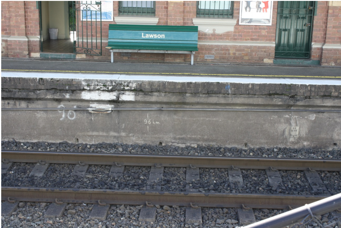
Figure 6 View of 1902 section of the platform showing brick additions above the original concrete coping
