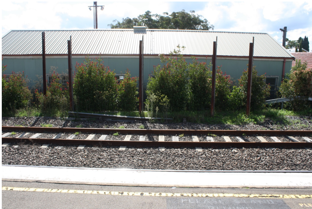
Figure 8 View north of tracks showing concrete sleepers
