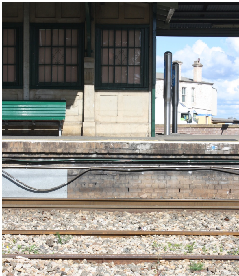
Figure 7 View of 1946 brick extension to platform
