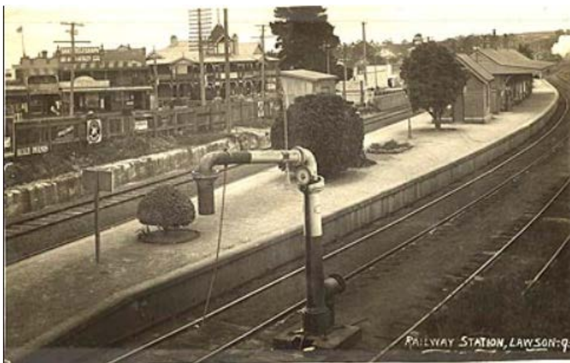
Figure 4 Lawson Station c.1910 from the north-east. Note rounded edge to coping. Source: NSW State Archives and Records Authority, digital id 17420_a014_a014000736
