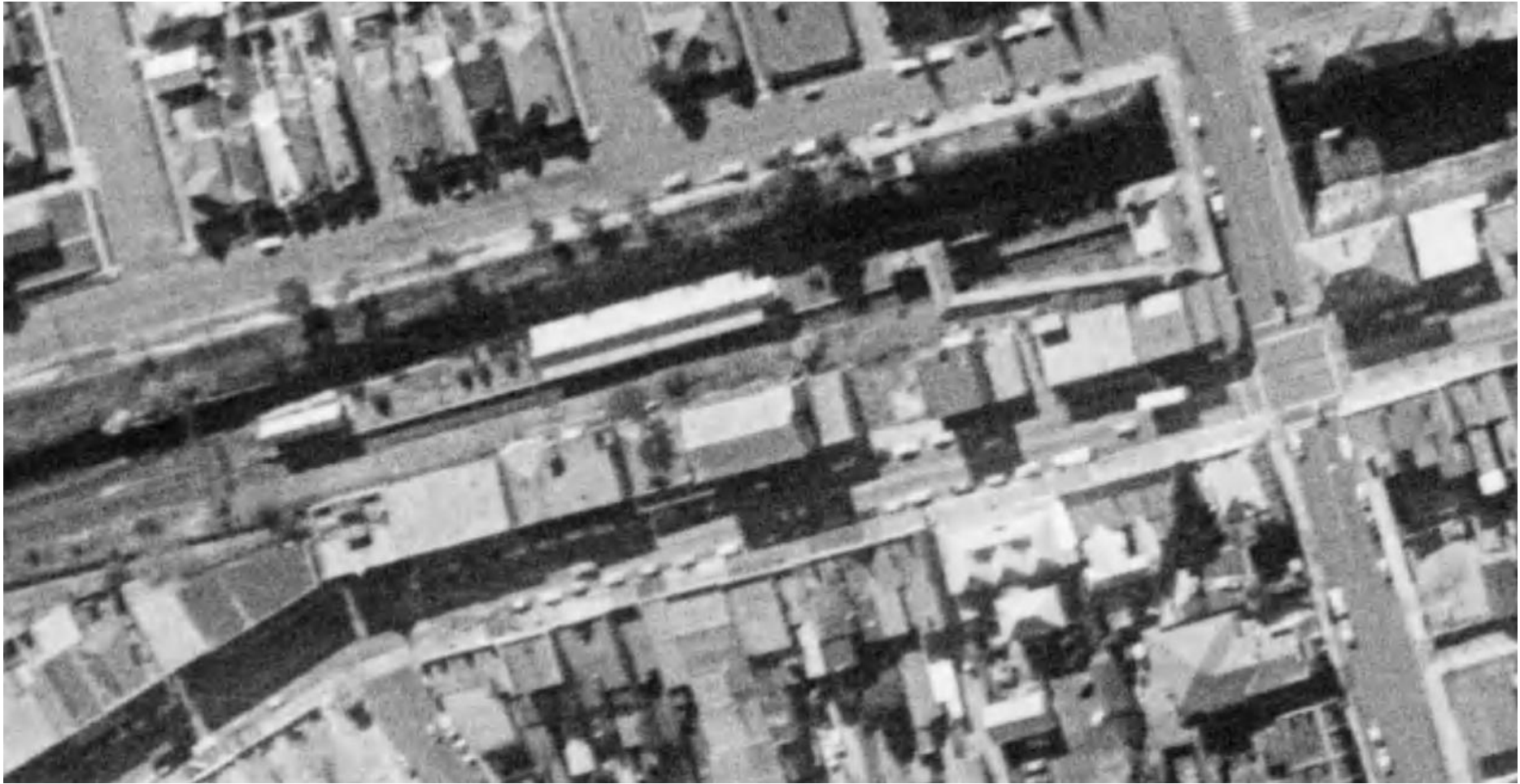
Figure 12: Aerial photograph of Lithgow Station in 1975 16
