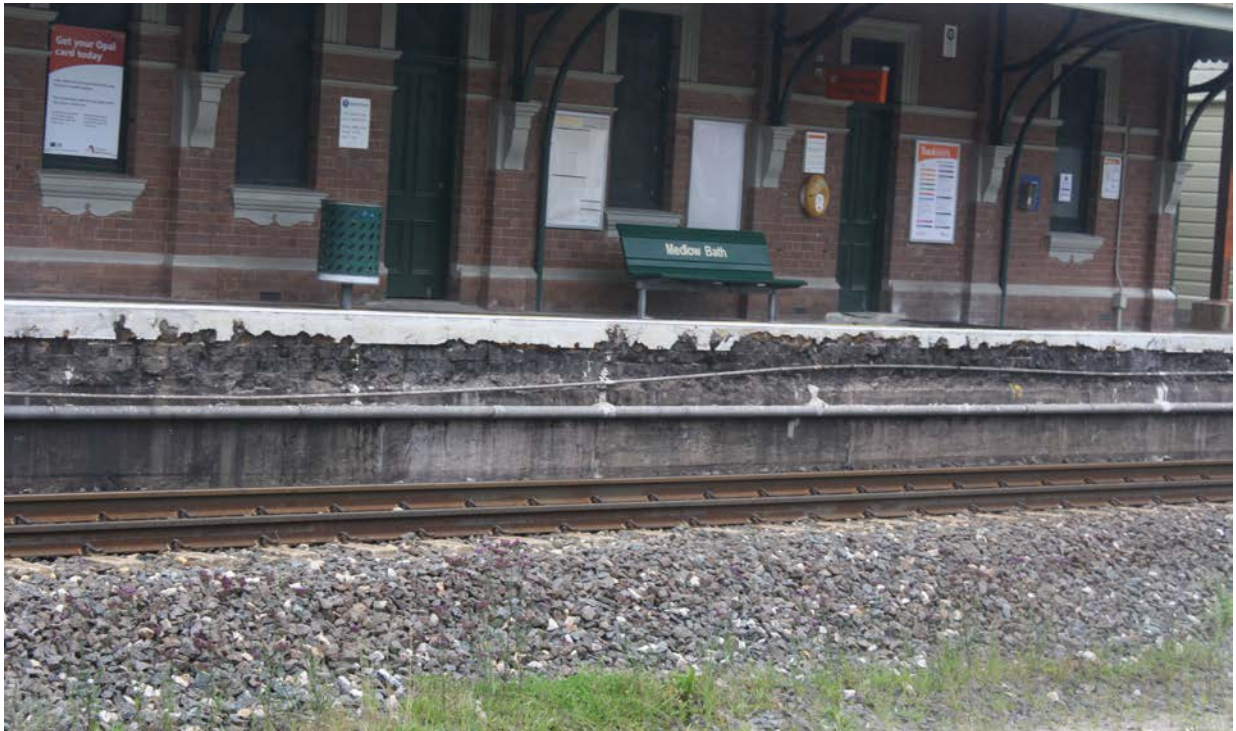
Figure 8 View of 1980/1981 coping modifications on platform 1
