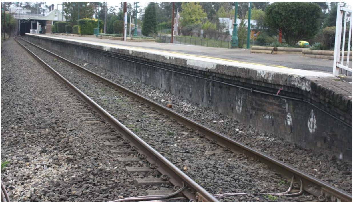
Figure 9 View north of tracks. Note concrete sleepers
