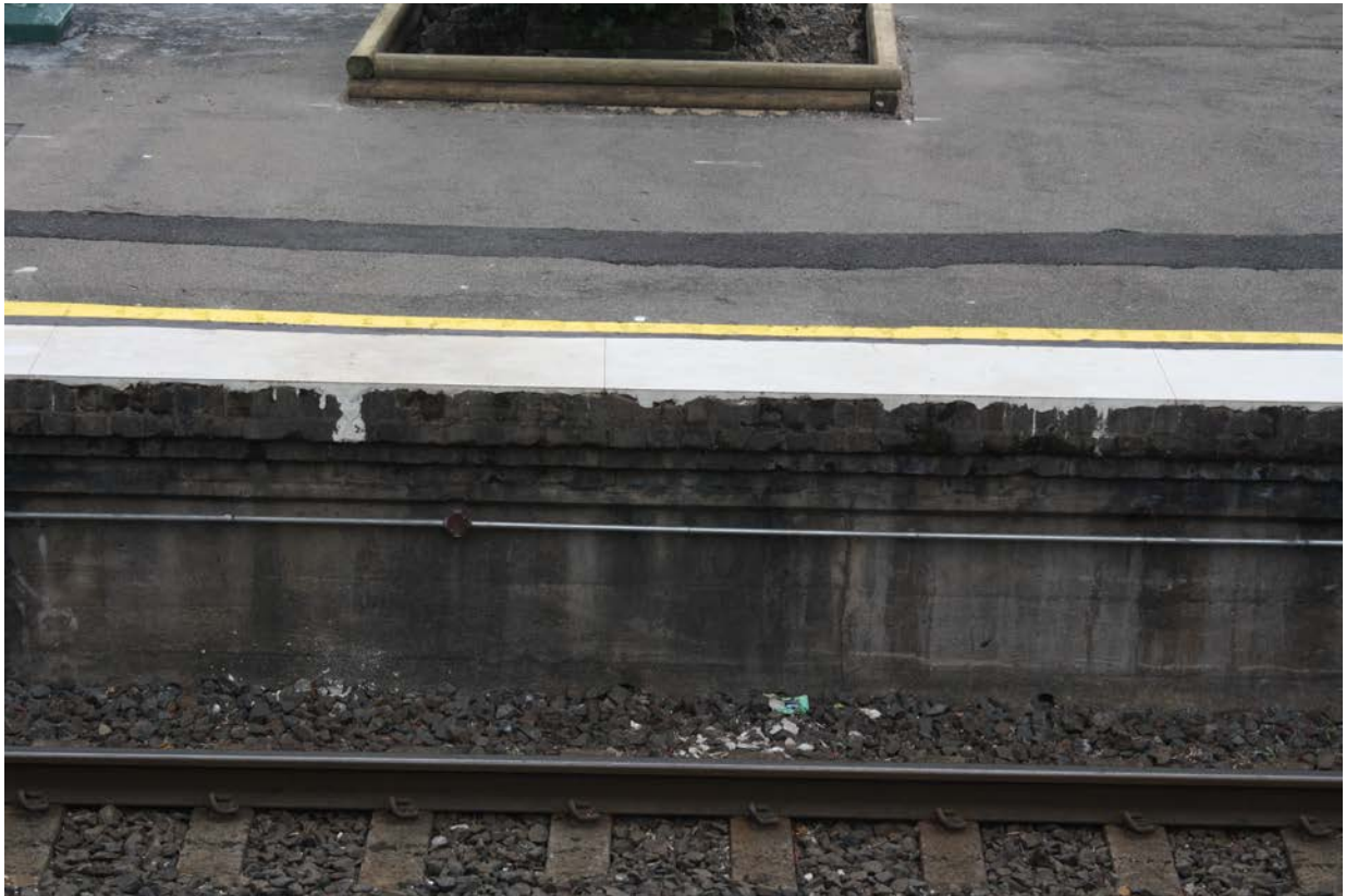
Figure 6 View of 1902 section of the platform showing the brick additions above
