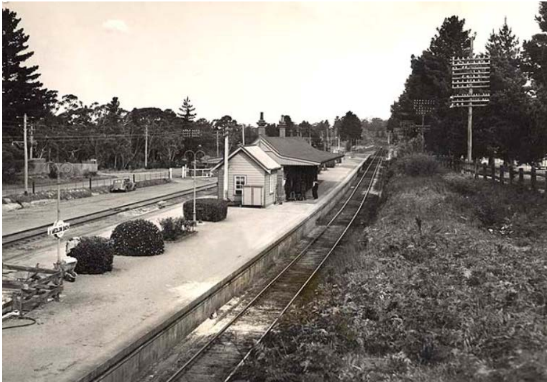
Figure 3 “Medlow Bath Railway Station (NSW)” 1954. View south. Held by State Archives & Records. Digital Id 17420_a014_a014000748
