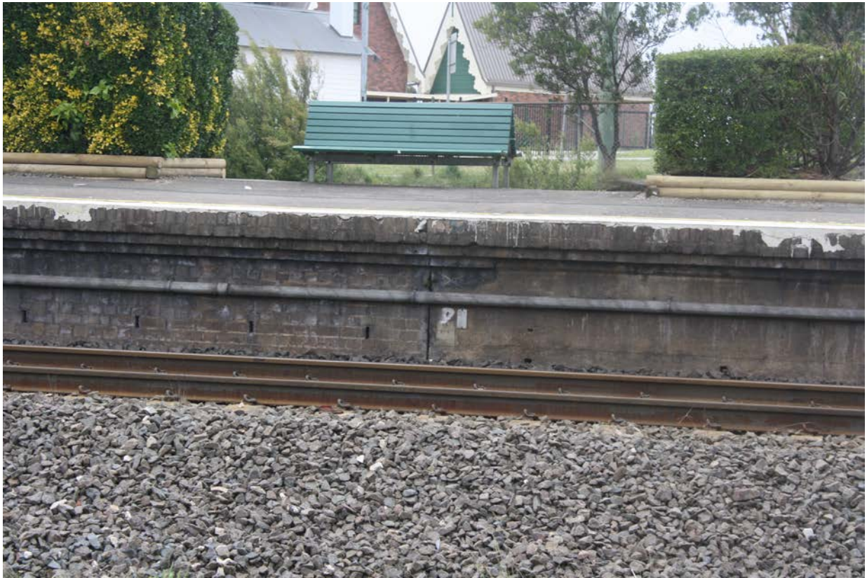
Figure 7 View of juncture between the 1902 unreinforced concrete platform (right of image) and the 1946 brick extension to platform (left of image)
