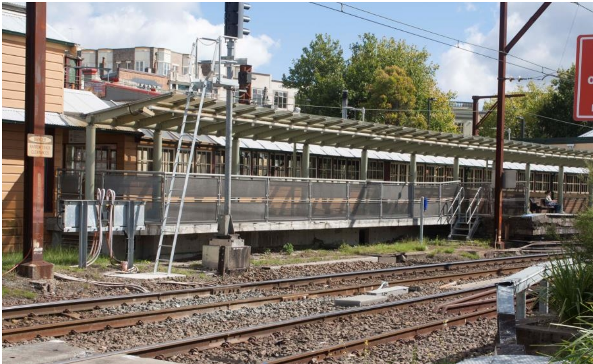
Figure 7 Junction between heritage platform and 2009 extension
