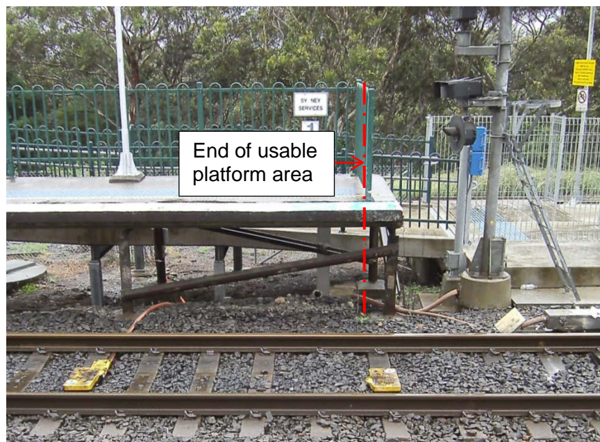
Figure 11: Measurement point for Edge of Platforms
