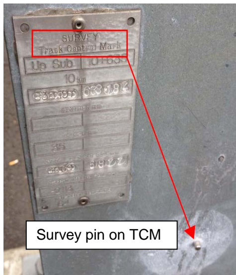
Figure 5: Survey pin located on an Overhead Wiring Structure
