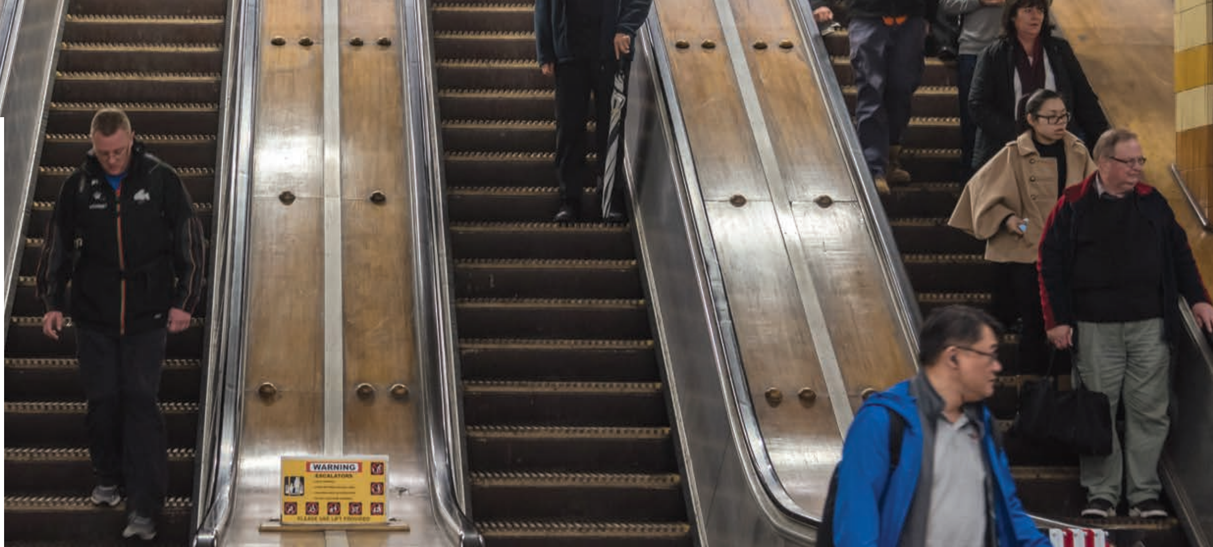
Figure 41: Wynyard Escalators 2016 in the last months of service. The distinctive timber panelling was a well-loved feature of the escalators and an element of the heritage that was included in the interpretation of the new escalators. (Source: Sydney Trains)
