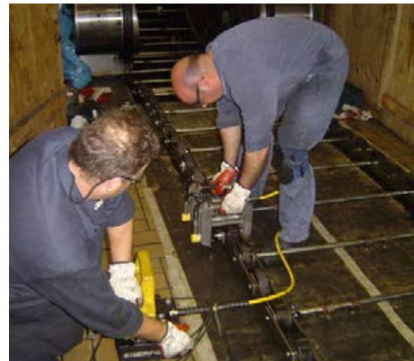
Figure 39: Step chain replacement. (Source: Sydney Trains)
