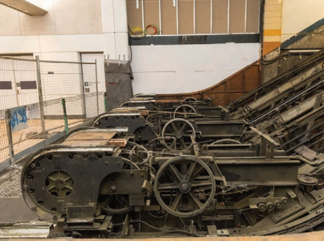
Figure 43: Escalator landings during demolition at Wynyard Station. (Source: Transport for NSW)
