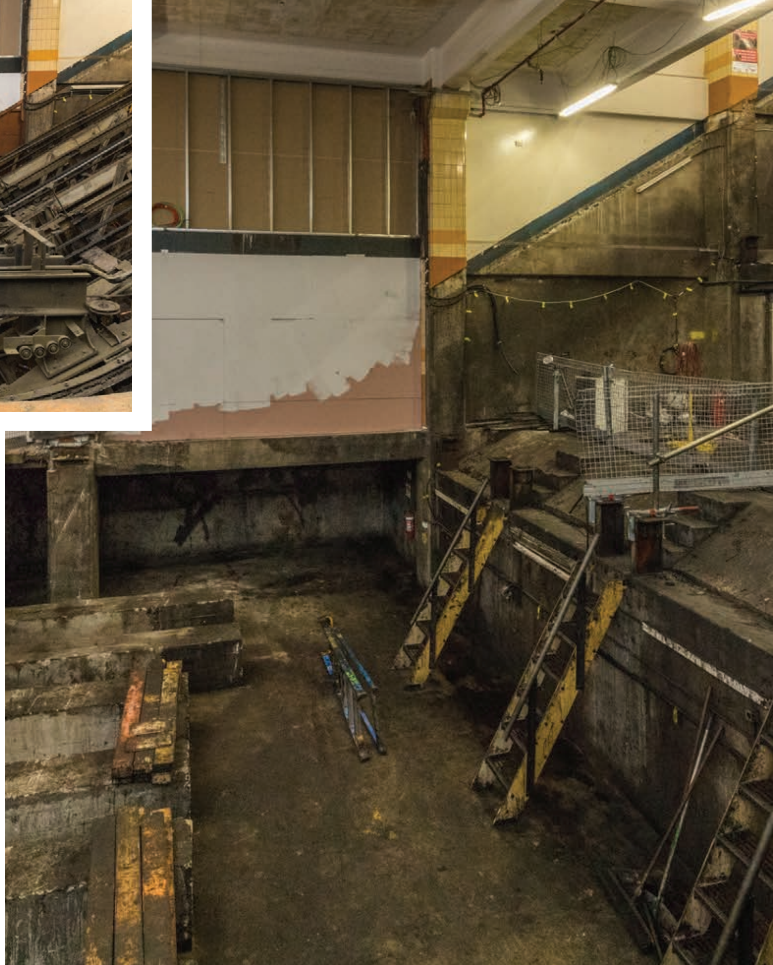
Figure 44: Void left after removing all four escalators from the York Street entry at Wynyard Station. (Source: Transport for NSW)
