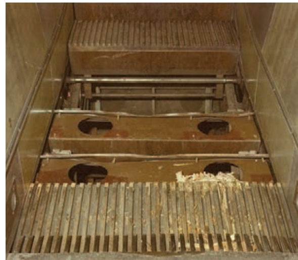
Figure 38: Town Hall escalator under repair in the 1980s. (Source: Sydney Trains)
