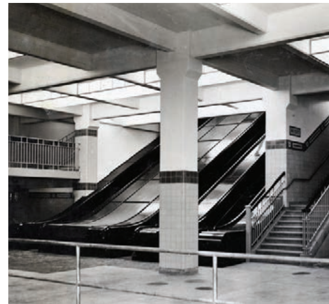
Figure 22: York Street entrance escalators to Wynyard Station just prior to the opening of the station in 1932. The station finishes are now complete. Note the set of stair either side of the escalator bank, which provided extra capacity for peak hours and as a back-up exit in case of emergency. (Source: State Archives and Records NSW 12685_a007_a00704_8722000031r)
