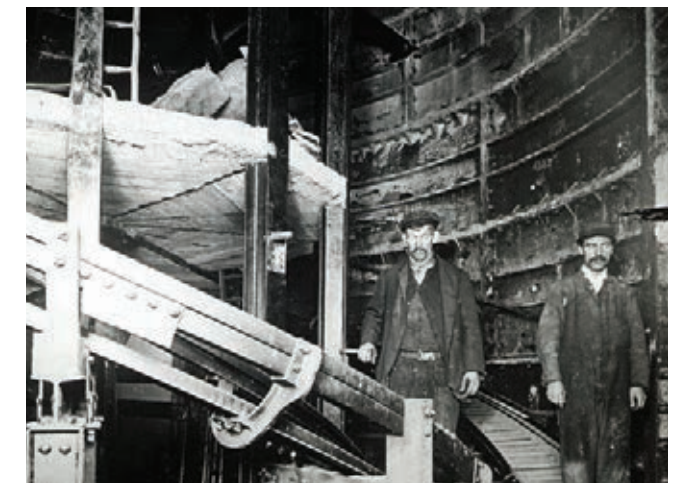
Figure 4: Two workmen stand on the double spiral. (Source: © TfL from the London Transport Museum collection). In March 1993 the remains of this walkway were found at the bottom of the lift shaft in Holloway Station, and are now in the care of London's Transport Museum depot at Acton.
