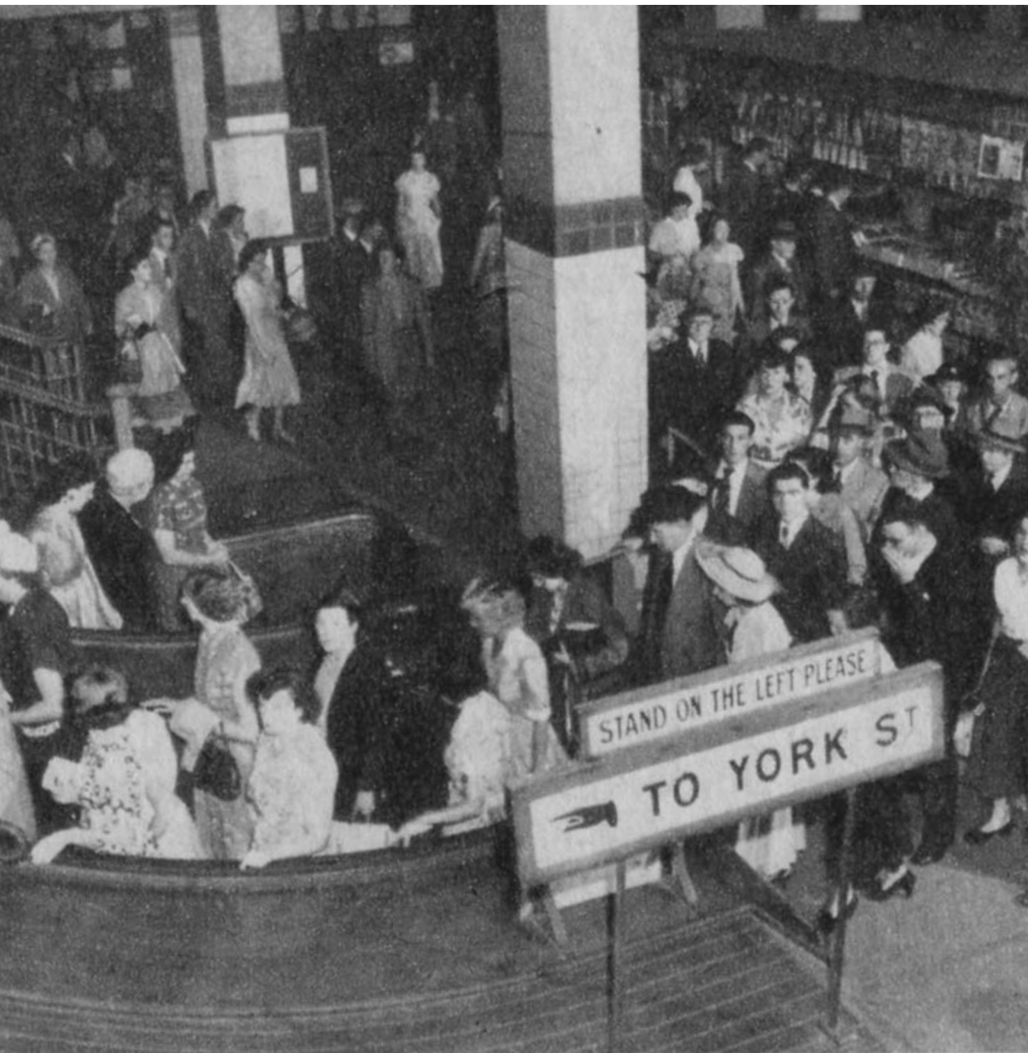
Figure 28: The Wynyard escalators at the morning peak hour in 1953. One escalator is running down, whilst the other two run up to York Street (the escalator on the near side is out of the frame in this photograph). Note the instructions to stand on the left. (Source: John Tipper, Collecting Books and Magazines)
