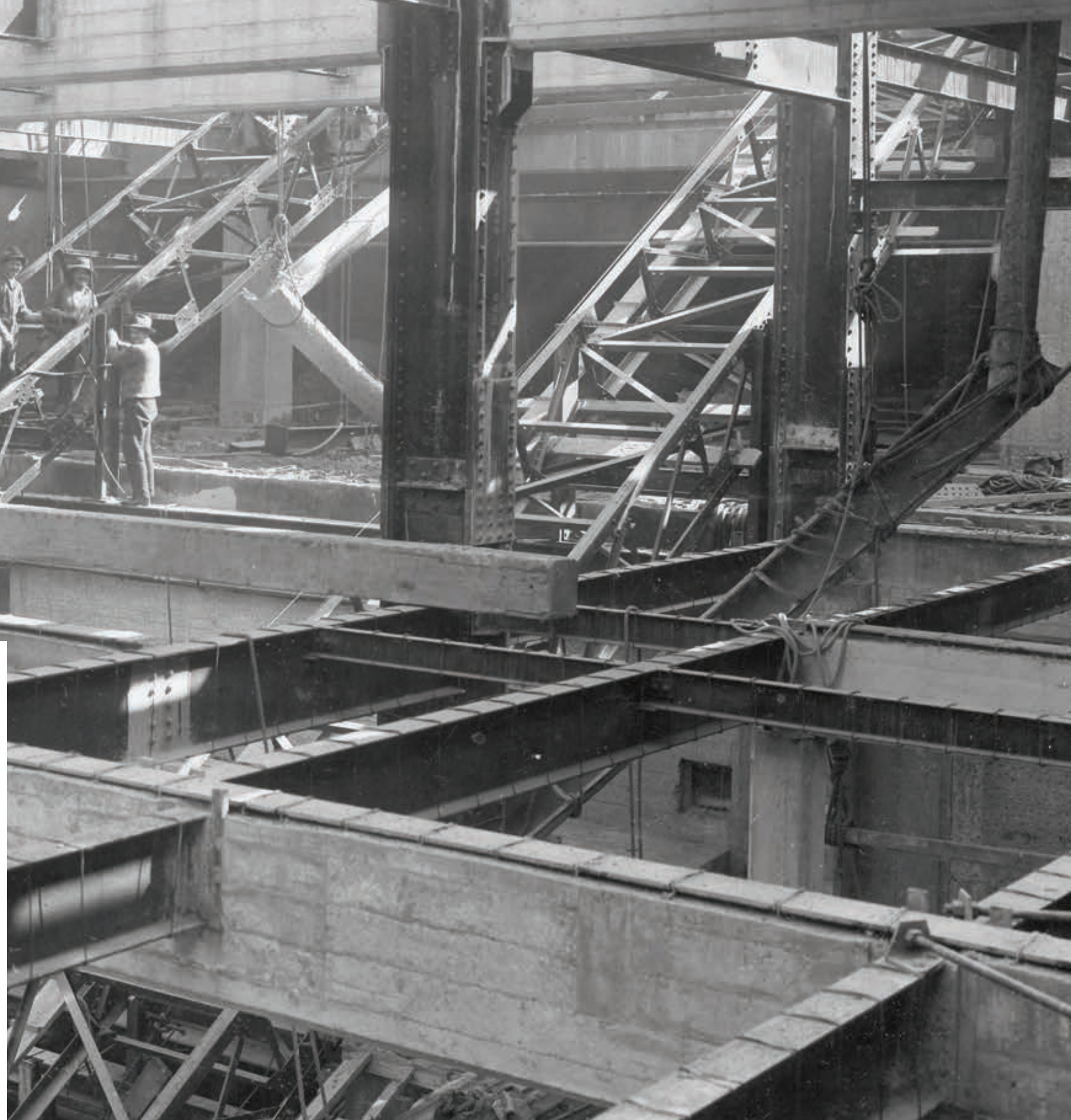
Figure 19: Installing the escalator trusses at Wynyard, August 1930. (Source: Sydney Trains)
