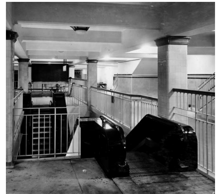
Figure 23: View of the Town Hall escalators from the concourse to platform 6 in a crossover pattern just prior to the station opening in 1932. (Source: State Archives and Records NSW. 12685_a007_a00704_8735000046r)
