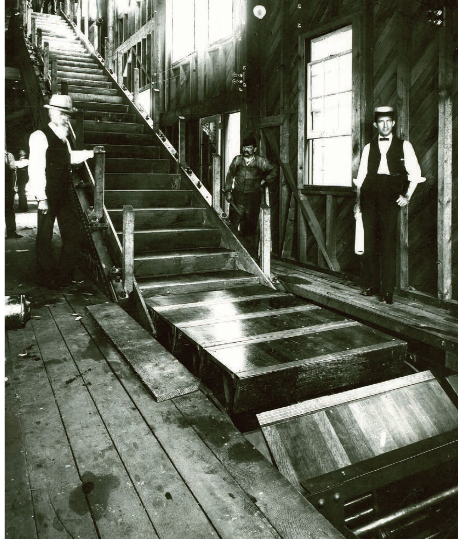
Figure 8: A flat step escalator under construction in Otis factory at Yonkers New York showing the completed treads and risers, 1899. (Source: Otis Elevator Company Archives)
