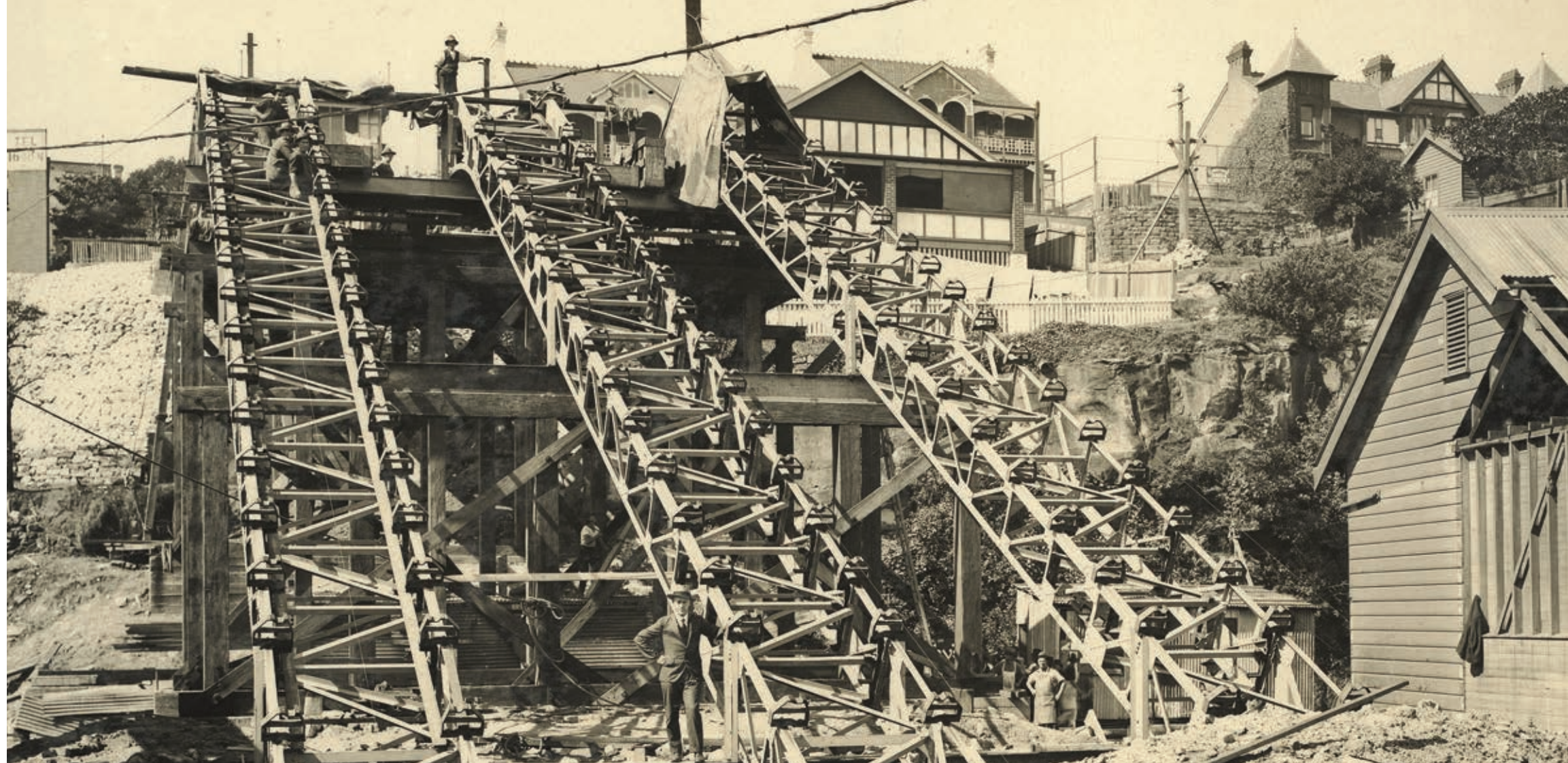
Figure 10: Milsons Point Station escalators in the course of installation by Waygood-Otis, 1924. The truss work is in place, with bracing for the escalators themselves also visible. (Source: State Archives and Records NSW ID 12685_a007_a00704_8722000084r)
