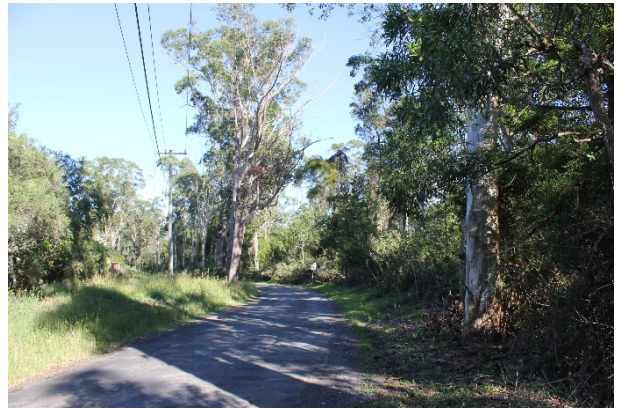
PCT 1564 – low condition – along Hereford Street
