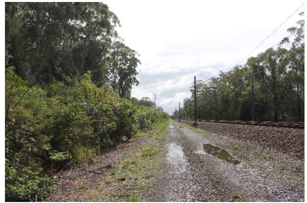
PCT 1568 – low condition – within rail corridor
