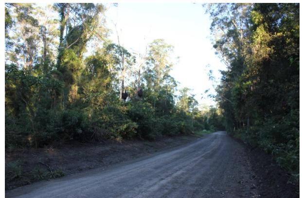
PCT 1568 – moderate condition – along Hereford Street
