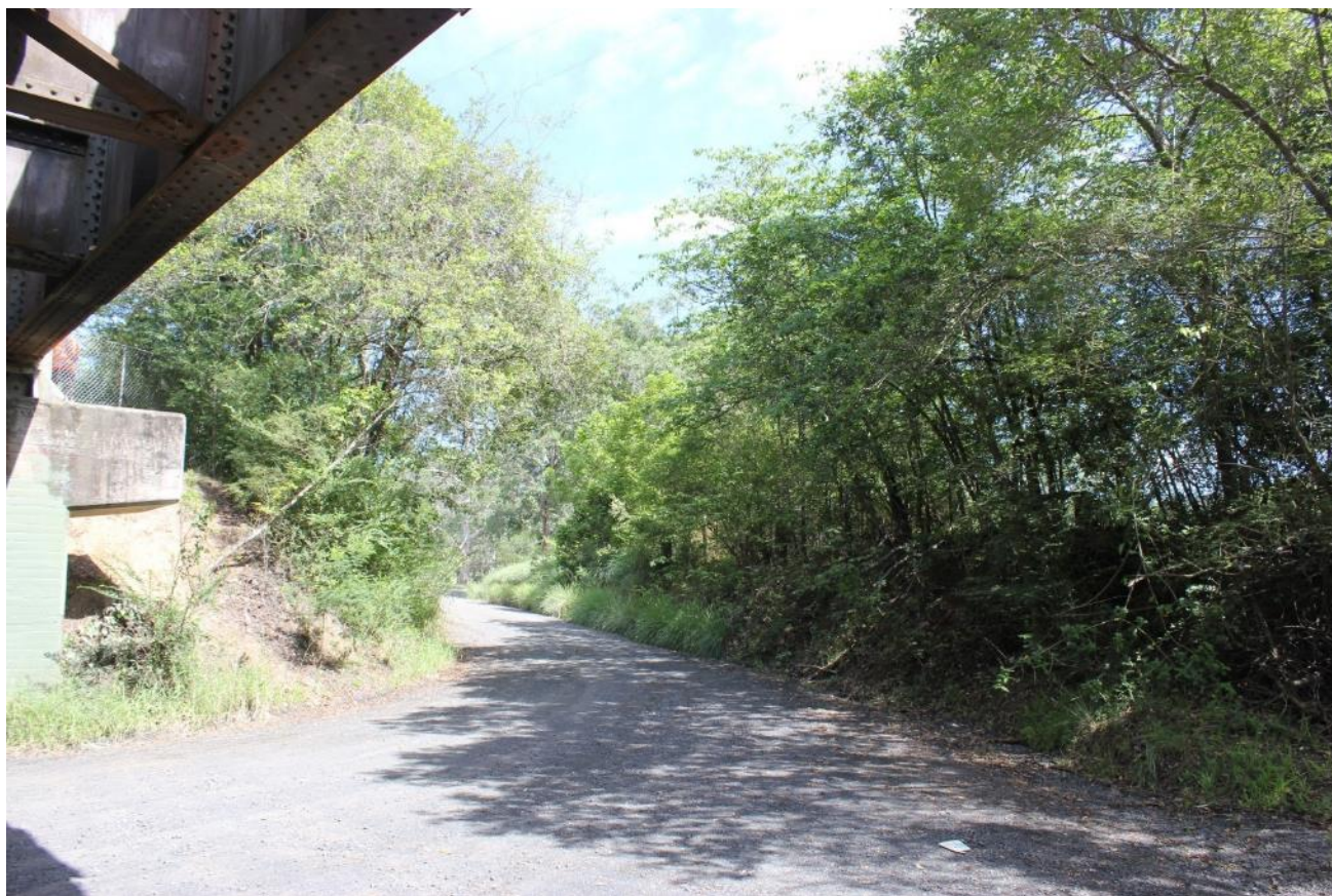
Figure 3.3 Existing Chittaway Road underpass (western side)
