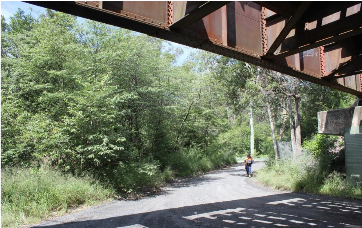
Figure 3.2 Chittaway Road underpass (eastern side, facing south-east)
