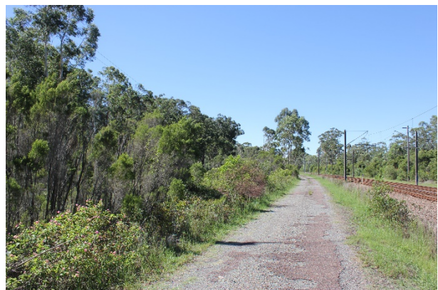
PCT 1718 – low condition – within rail corridor
