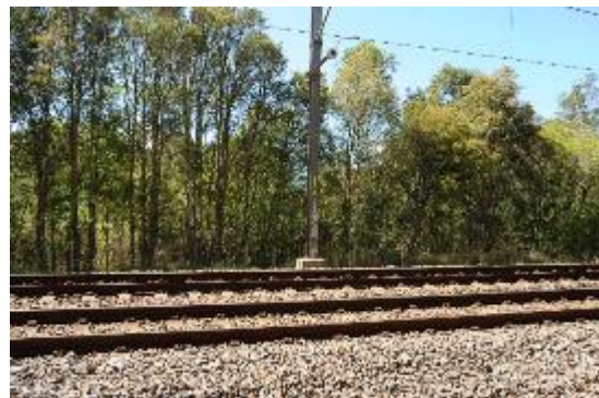
Plate 6.2: Detail of existing rail line including ballast base
