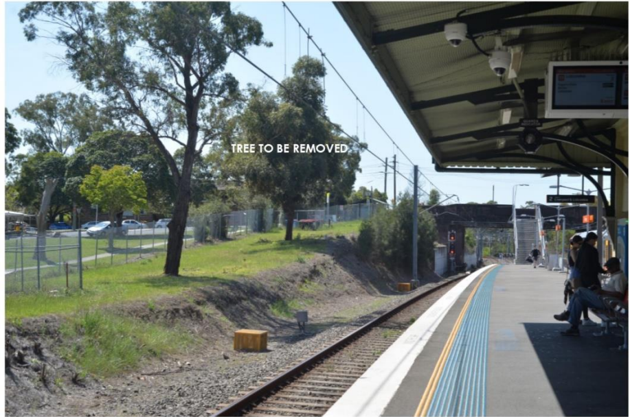
FIGURE 4-3: TREE REQUIRING REMOVAL TO ALLOW FOR CONSTRUCTION OF PROPOSAL
