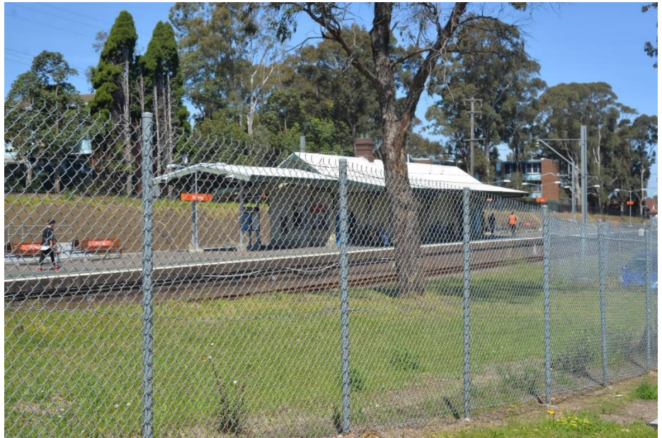
FIGURE 3-3: VIEW OF BIRRONG STATION BUILDING FROM HUDSON PARADE
